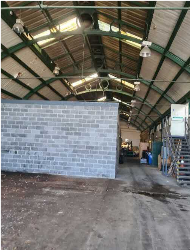
Fig 35. Platform 2. The floor filled in. Free standing storage units in blockwork fill the space.
