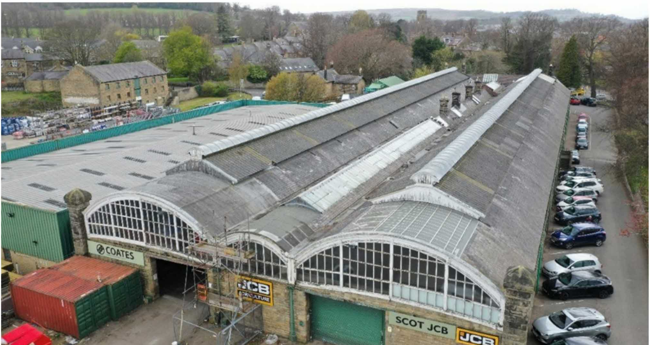
Fig 29. - The roof has lost much of the original glass and been replaced with asbestos sheets. However, the roof remains largely original in structure, profile and slates. Original chimneys are in place.
