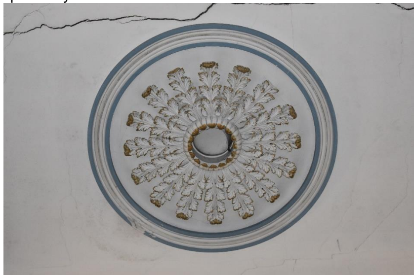
Central Ceiling Rose – the crack is not thought to be structural and is repairable.
