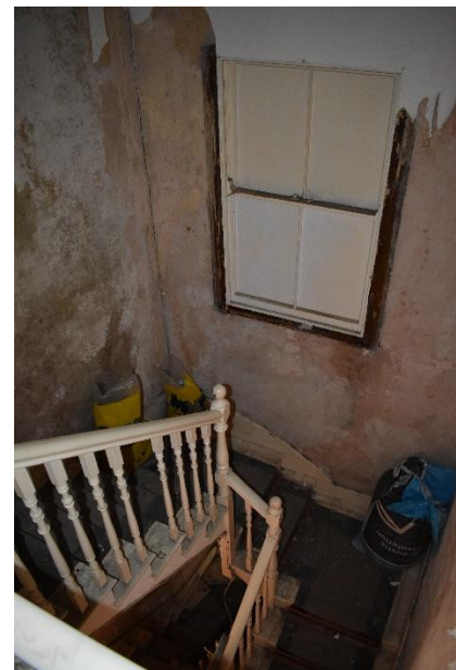
Stairwell with blocked original sash window
