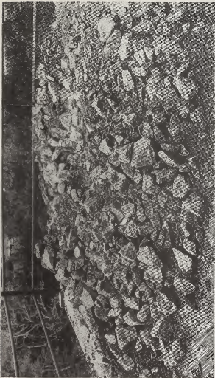
Plate 8. Frosterley lime kilns, 1969: the limestone piled high on the kiln-top, became hot to the touch, before it gradually sank into the kiln.
