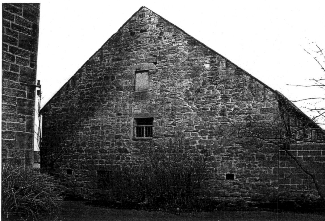
Figure 16 The Maltings: the west gable, seen from the school house garden. An earlier gable end is visible here between the levels of the cill of the upper window and the lintel of the lower one.
