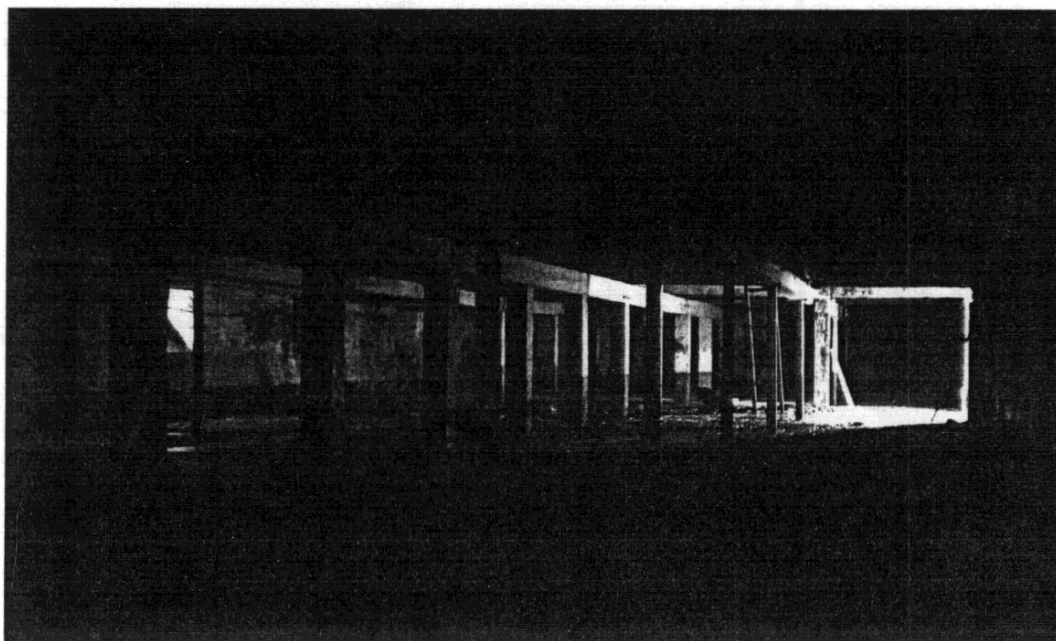
Figure 19 A view of the lower growing floor (the ground floor) in the malthouse. This view, from the same relative position as Figure 18, shows the dark state of this part-buried room. The floor, like that above, is a concrete screed. The square columns along the centre of the floor are made of sandstone.
