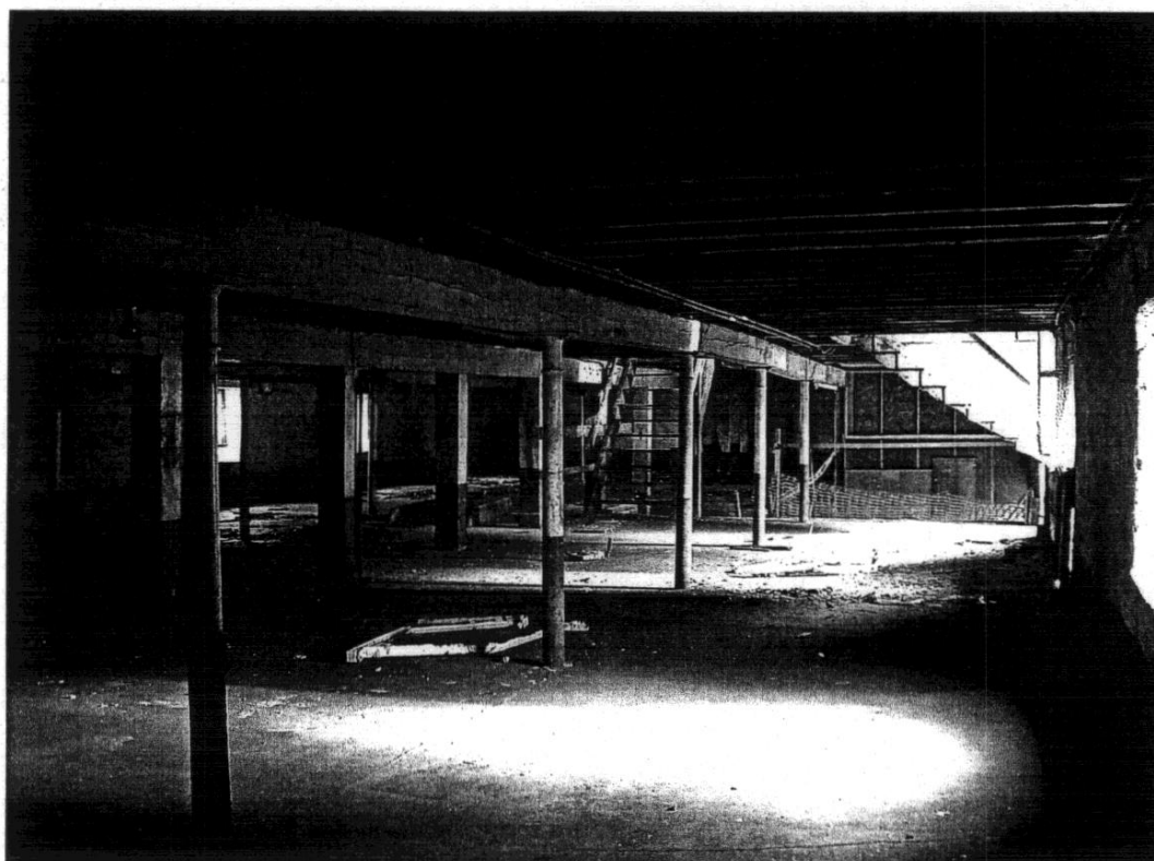
Figure 18 The upper growing floor of the malthouse, looking north-east. Cast iron and timber supports to the floor above are carried by iron and stone columns on the ground floor.
