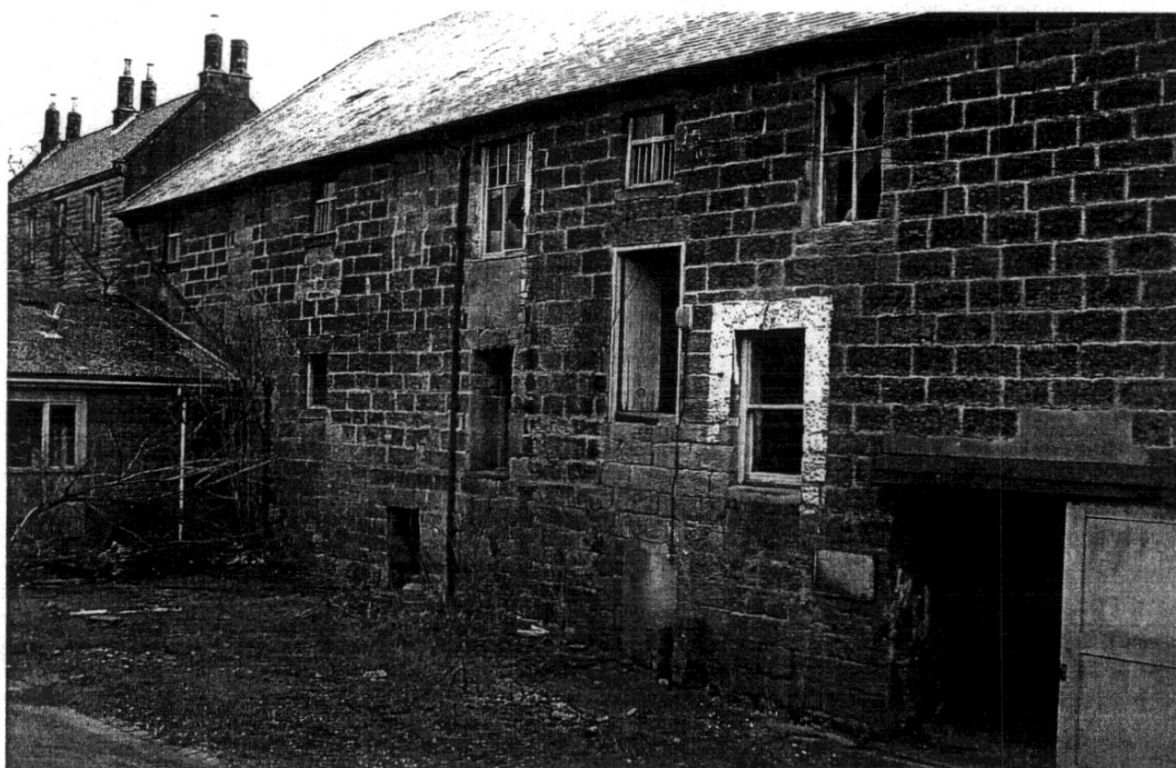
Figure 14 The Maltings: west end of the south front. Contrast the squared masonry with the rubble seen in Figure 10. A regular pattern of tall upper windows can be made out, despite later changes.
