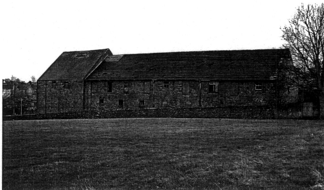
Figure 10 The Maltings, from the north-west. The irregularity of the fenestration can be seen in this view; the malt kiln to the left has no original openings left. The lower row of windows serves the upper growing floor, and the west end of the ground floor is below ground level.
