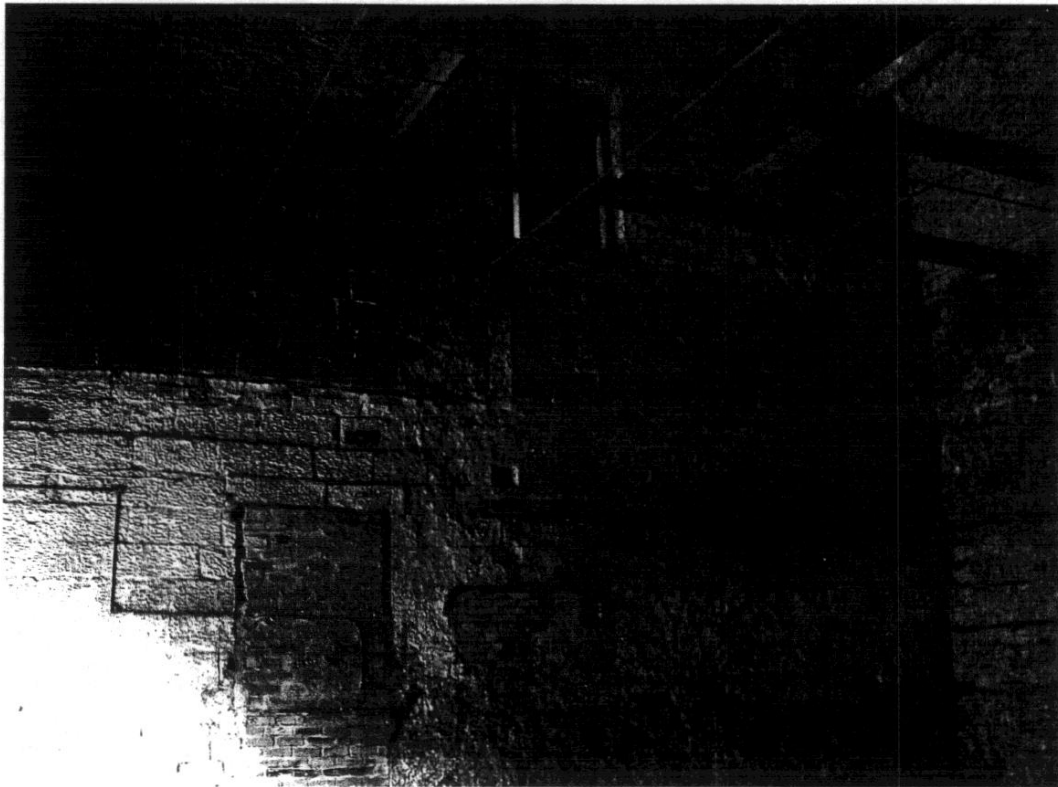
Figure 20 The malt kiln. A view from the south-east corner, looking at the east end of the malthouse. The lower door led to the hearths, and the upper gave access to the drying floor, which lay at the level of the steel joists. Between the levels of the doors there was once a row of four windows across the width of the wall.
