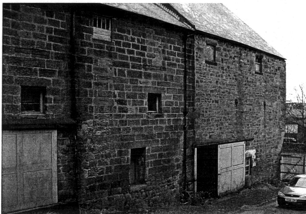
Figure 15 The Maltings: the east end of the south front. The straight joint between the fabric of the malting and the kiln is clear here. Altered windows, like those seen in Figure 14 are visible on the upper floor. Behind the left-hand downpipe the ends of a flight of stone steps rise towards a blocked door. This gave access to the upper growing floor.
