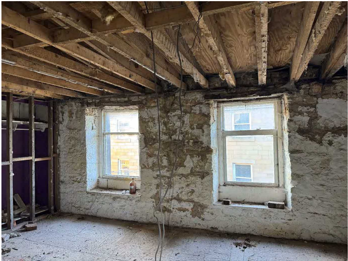
P37 – Internal view – front elevation wall, second floor level – room (6) Severe decay within timber lintels above window openings (viewed from distance).
