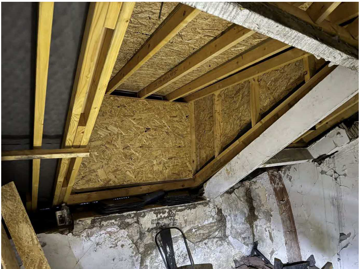
P44 – Recently constructed timber dormer to rear of property. Dormer constructed off original timber roof structure.
