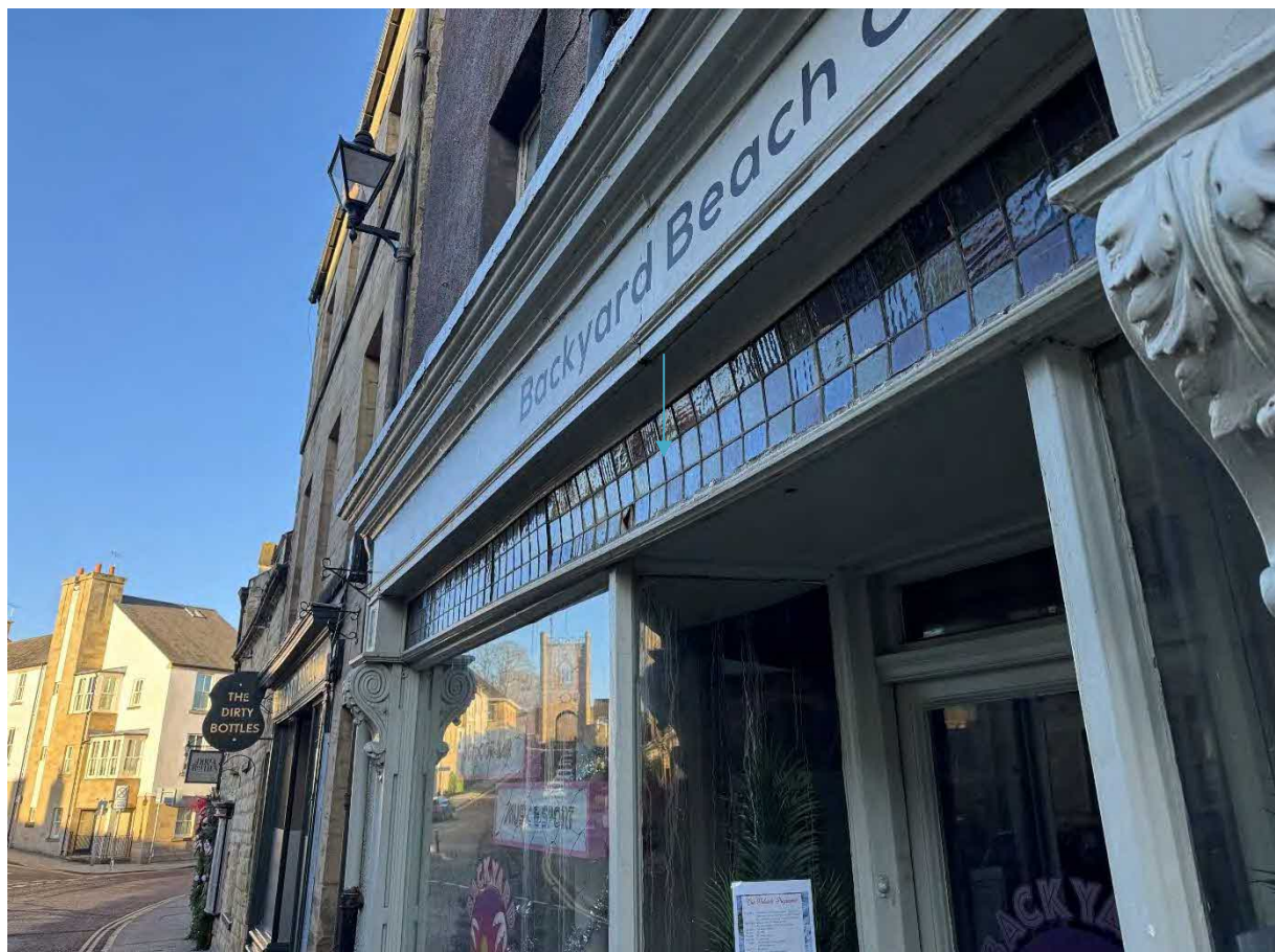
P10 – Deflection within shopfront beam above ground floor entrance with cracking to first floor wall and distortion and damage to shopfront fascia.
