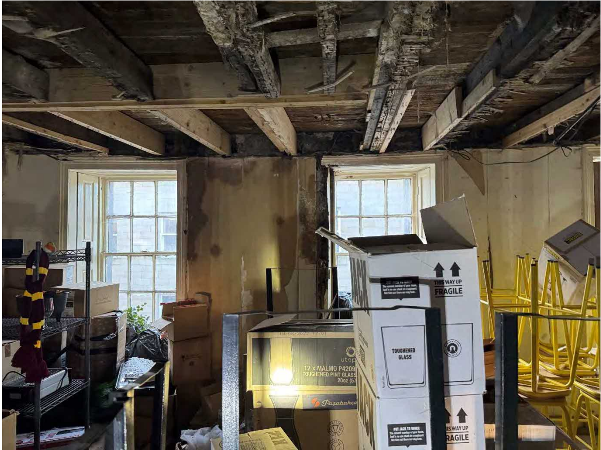
P25 – First floor level – front room (3). Severe decay (wet and dry rot) within timber second floor structure. Past modifications and repairs to second floor structure appear to have been poorly implemented and the floor is potentially unsafe.
