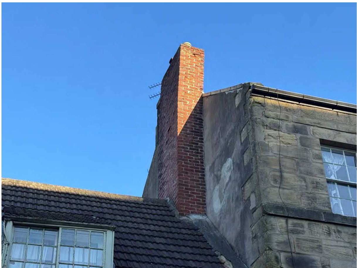
P54 – Chimney stack to party wall of 30-32 Narrowgate – viewed from front (south). Chimney stack has poor vertical alignment, leaning out to east (estimate approx 100mm).
