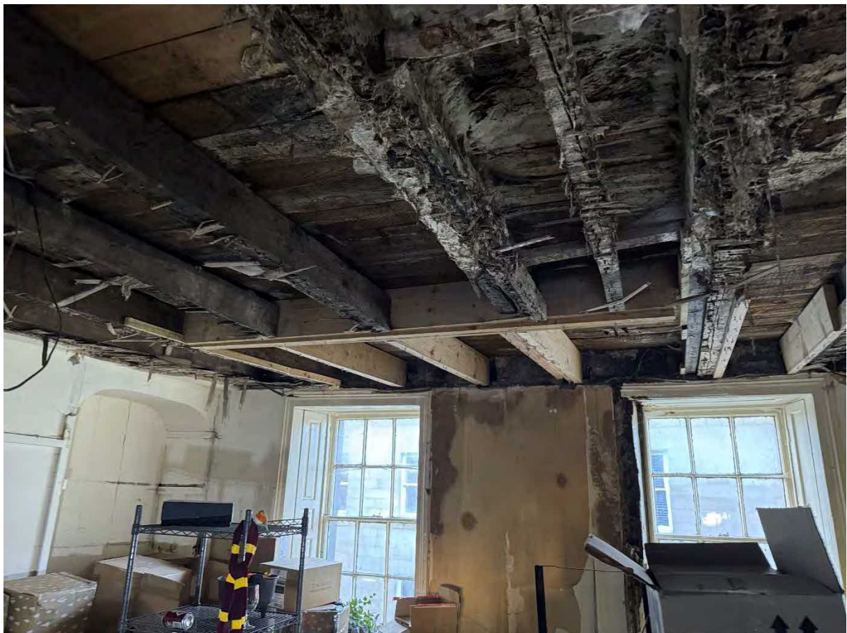
P24 – First floor level – front room (3). Severe decay (wet and dry rot) within timber second floor structure. Past modifications and repairs to second floor structure appear to have been poorly implemented and the floor is potentially unsafe.
