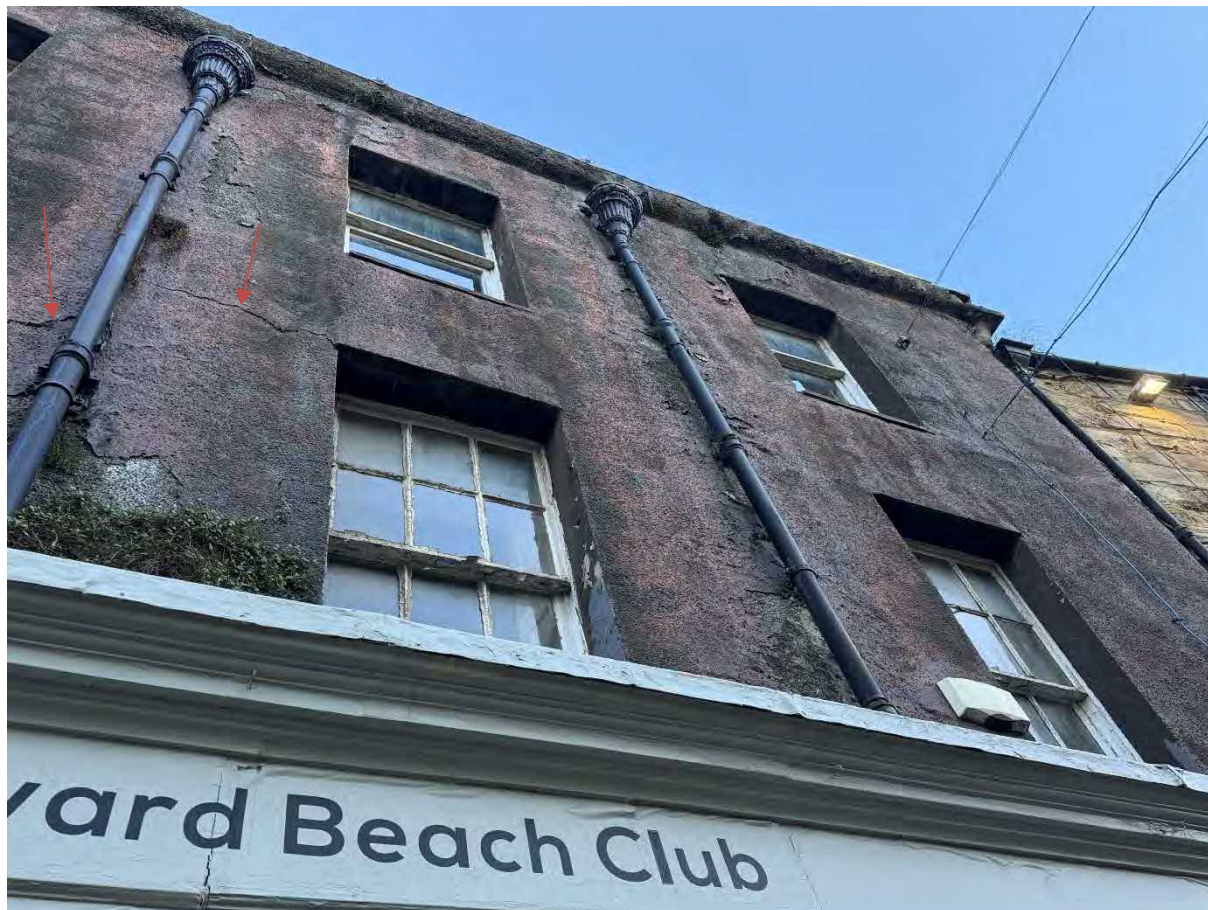
P13 – Cracking within first floor wall above defective shopfront beam. Defective roof rainwater drainage.
