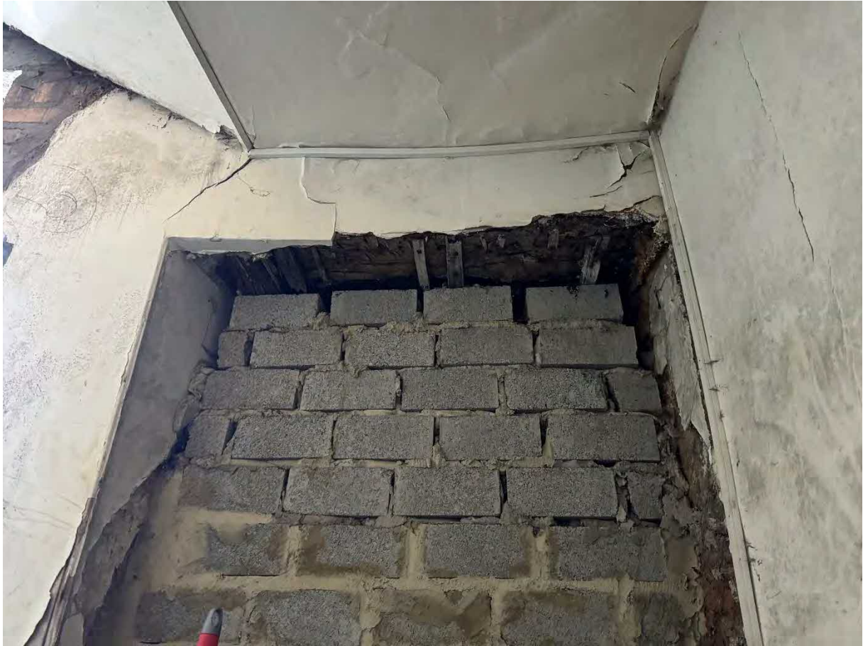
P47 – Poorly infilled window opening within rear elevation wall – staircase. Built in timber lintels appear decayed.
