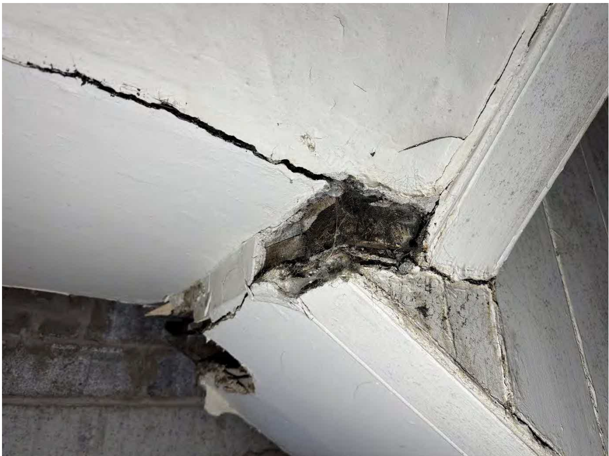
P50 – Underside of internal timber staircase – first to second floor level - has poor alignment with evidence of timber decay. Staircase is potentially unsafe.
