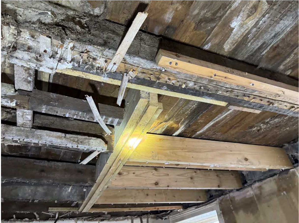
P27 – First floor level – front room (3). Severe decay (wet and dry rot) within timber second floor structure. Past modifications and repairs to second floor structure appear to have been poorly implemented and the floor is potentially unsafe.
