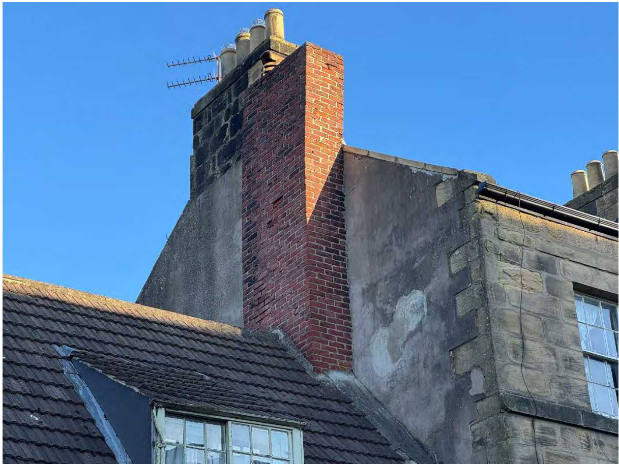
P53 – Chimney stack to party wall of 30-32 Narrowgate – viewed from rear. Chimney stack has poor vertical alignment, leaning out to east (estimate approx 100mm).
