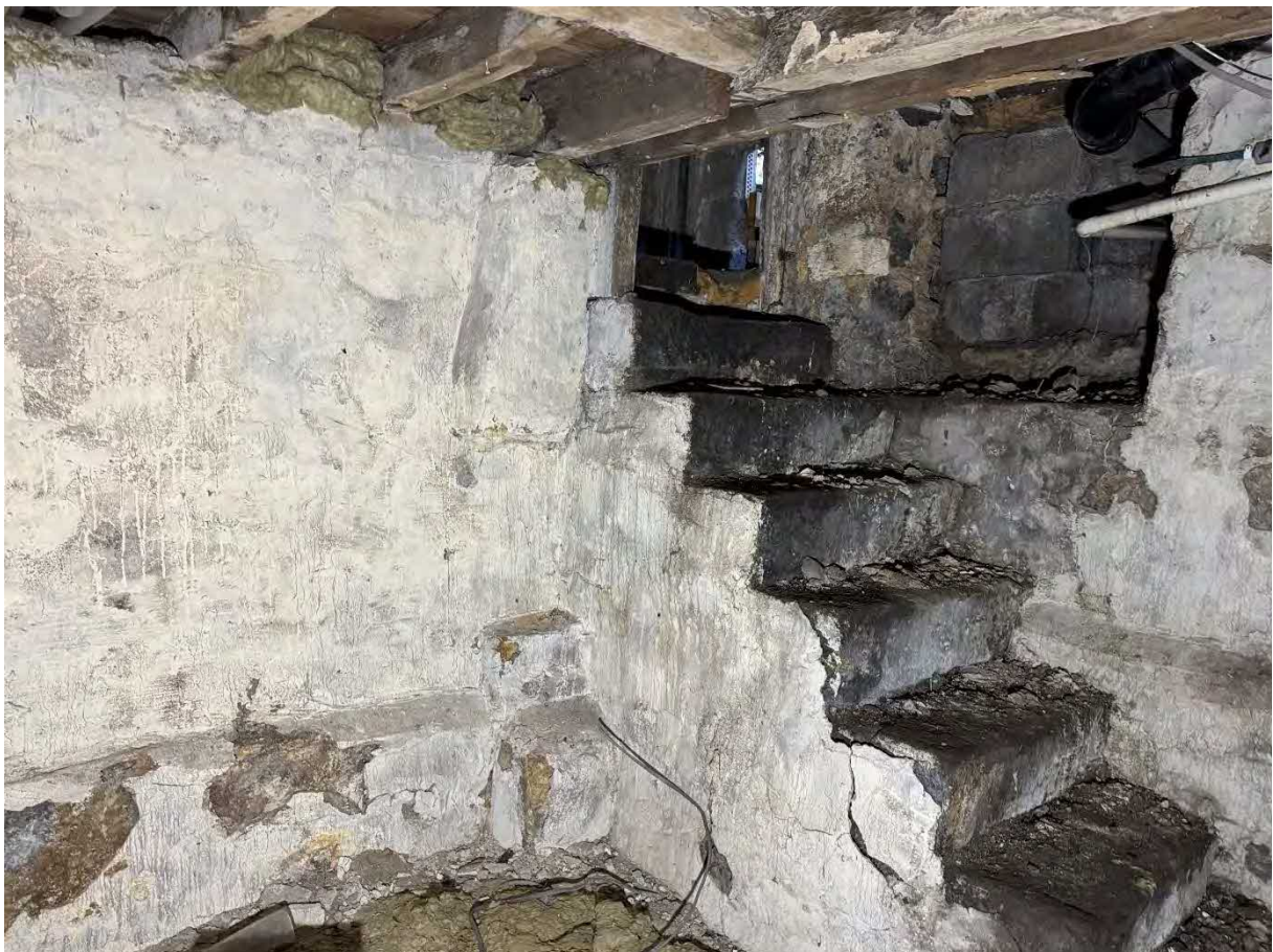
P16 – Entrance to partial basement to rear of property. Stone steps into basement – timber ground floor over.
