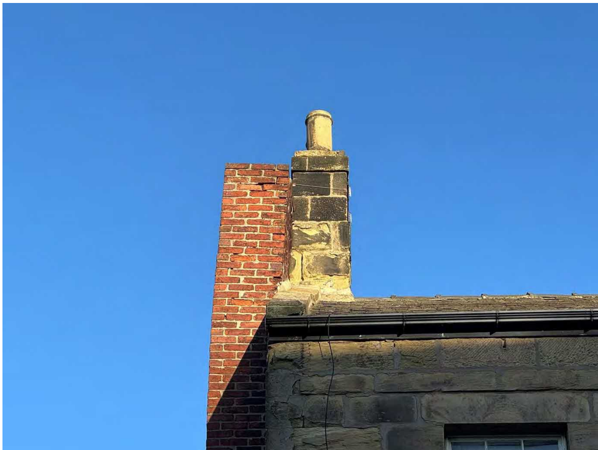
P55 – Chimney stack to party wall of 30-32 Narrowgate – viewed from front (south). Chimney stack has poor vertical alignment, leaning out to east (estimate approx 100mm).
