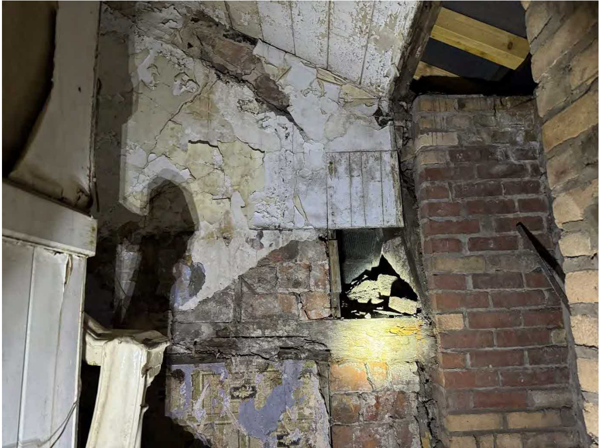
P33 – Loose masonry and decayed timber within wall at second floor landing.
