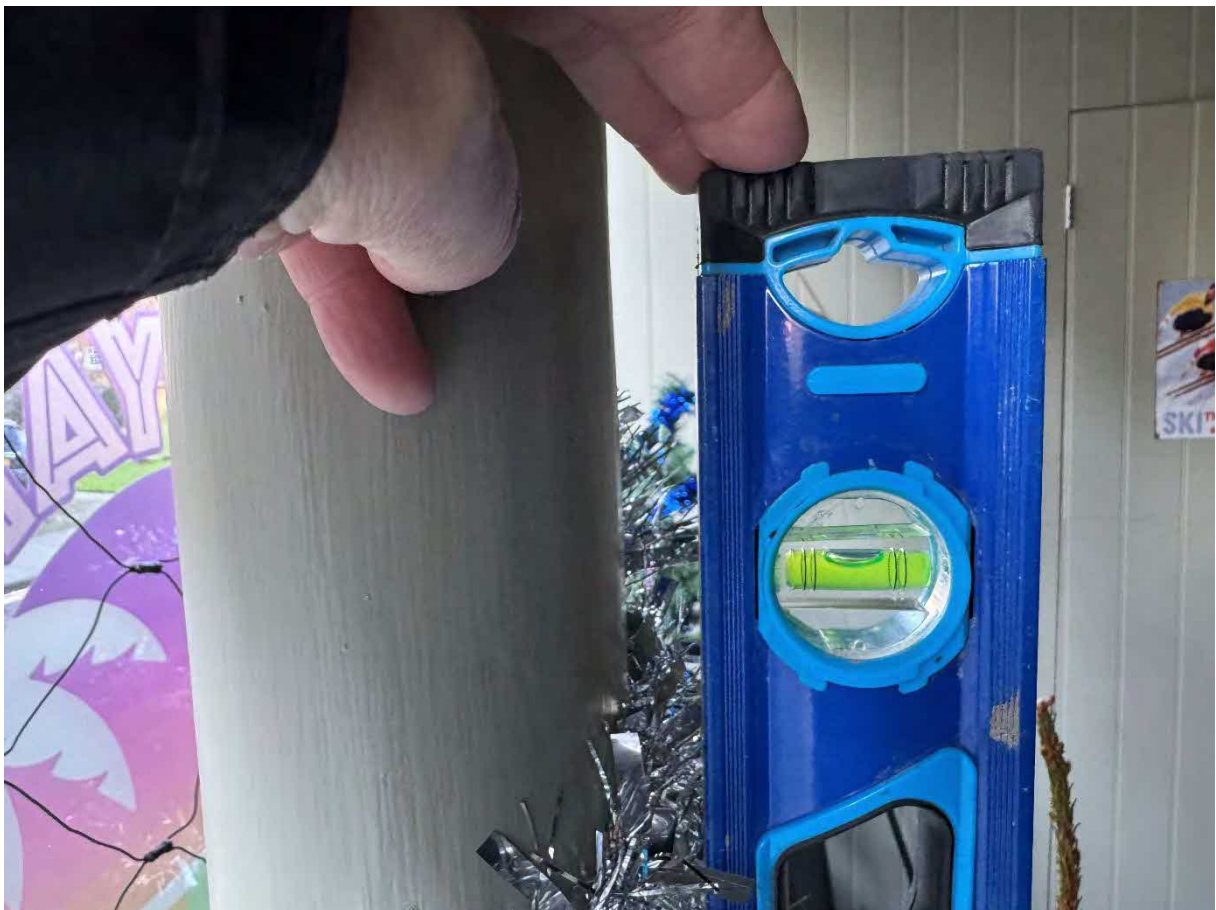
P20 – Head of outer (two) cast iron columns lean out to south by approx 20mm over 1.0m level length.
