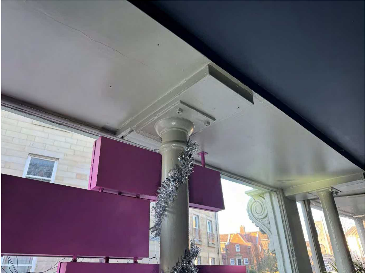
P19 – Cast iron columns supporting shopfront beams.
