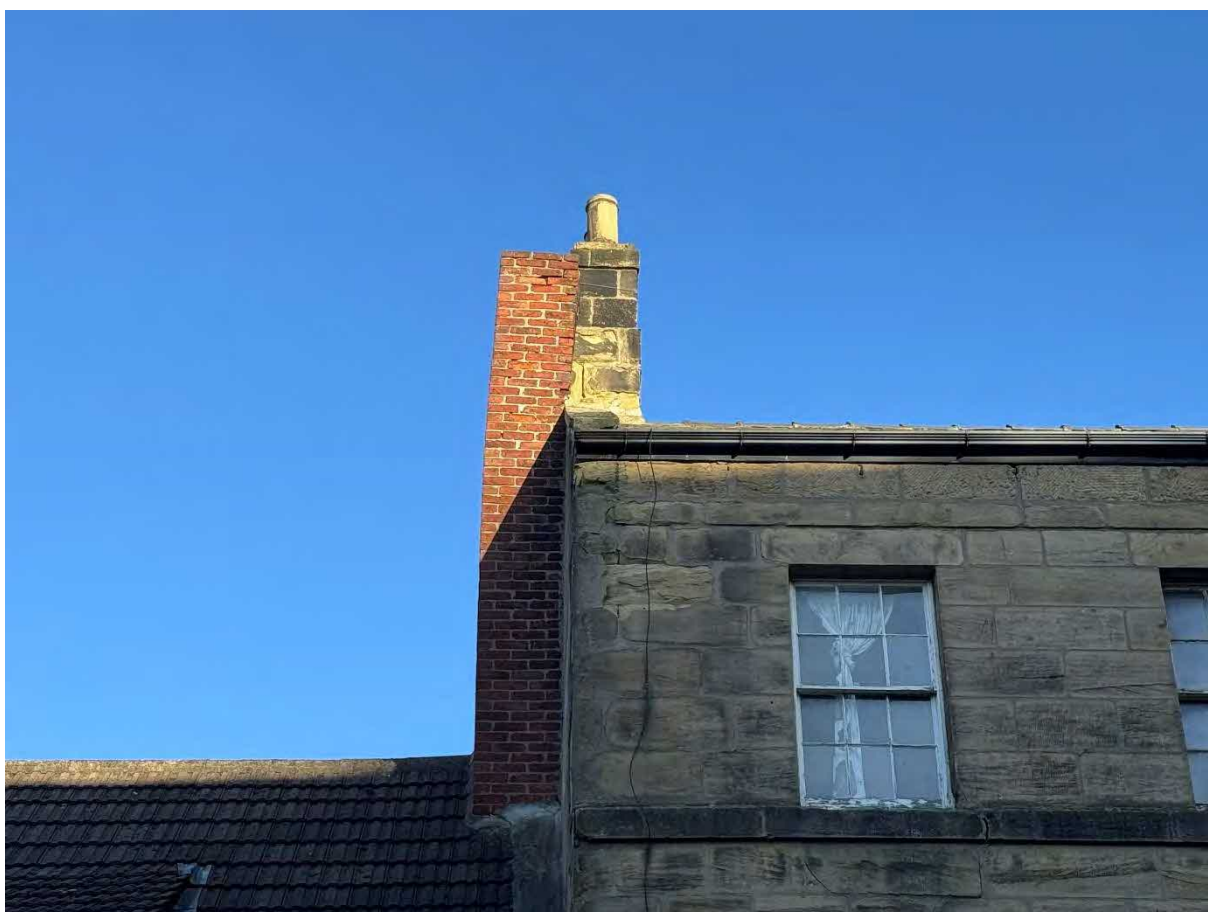
P56 – Chimney stack to party wall of 30-32 Narrowgate – viewed from front (south). Chimney stack has poor vertical alignment, leaning out to east (estimate approx 100mm).
