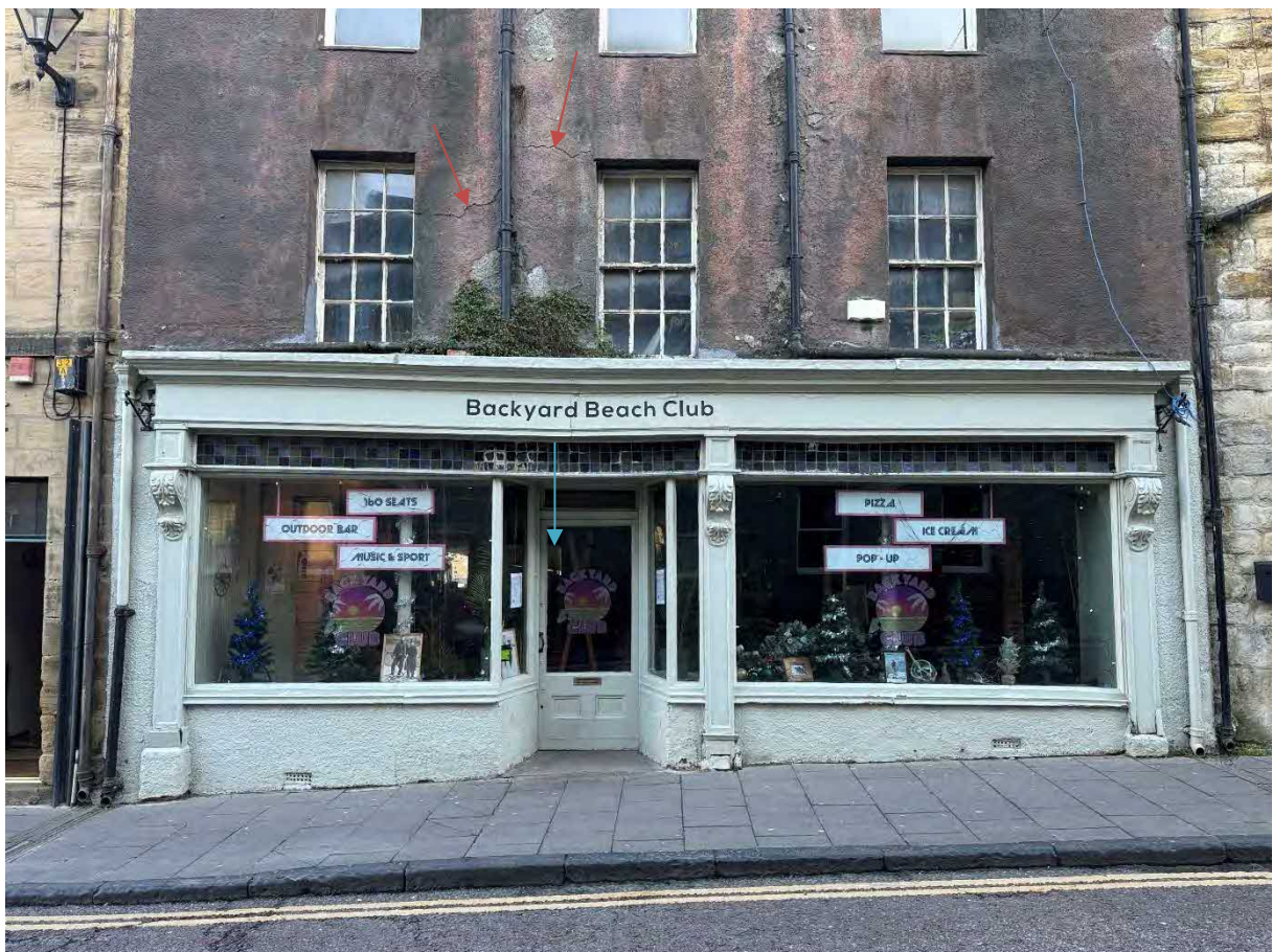
P8 – Cracking within first floor wall (red arrows) above deflected shopfront beam (blue arrow)
