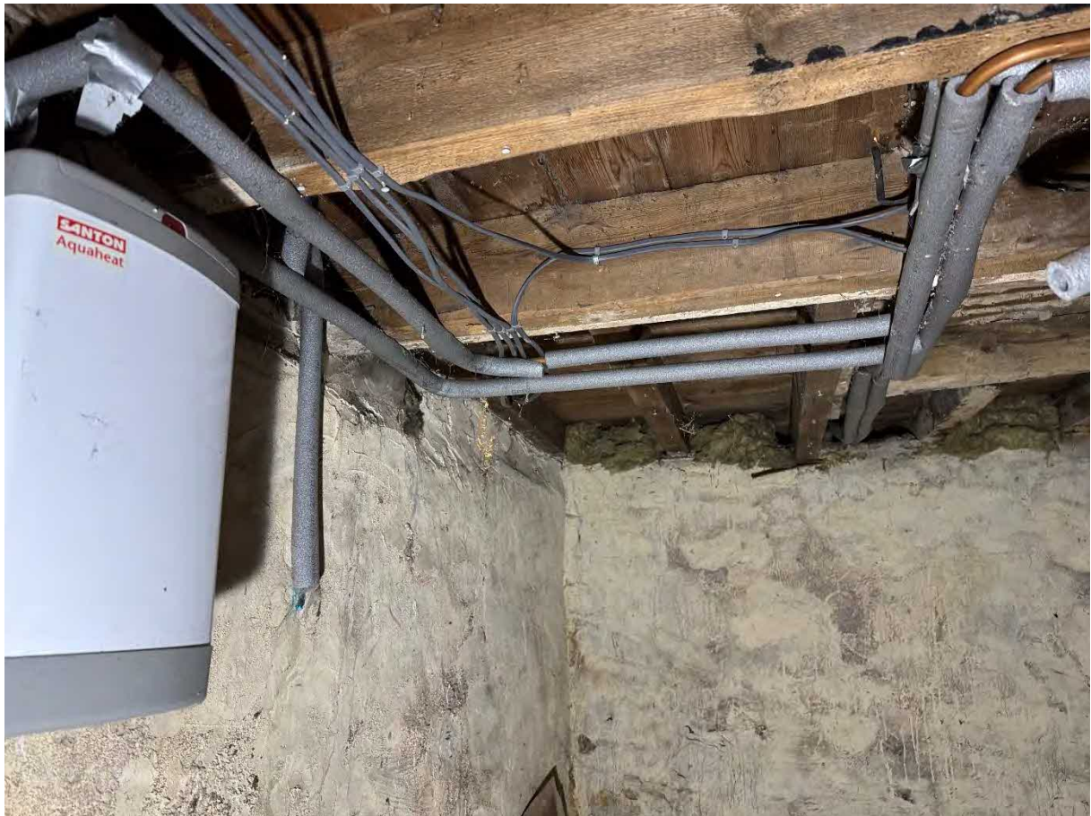
P17 – Underside of timber ground floor – viewed from within basement.
