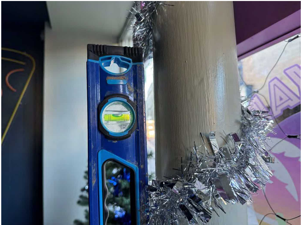
P21 – Head of outer (two) cast iron columns lean out to south by approx 20mm over 1.0m level length.
