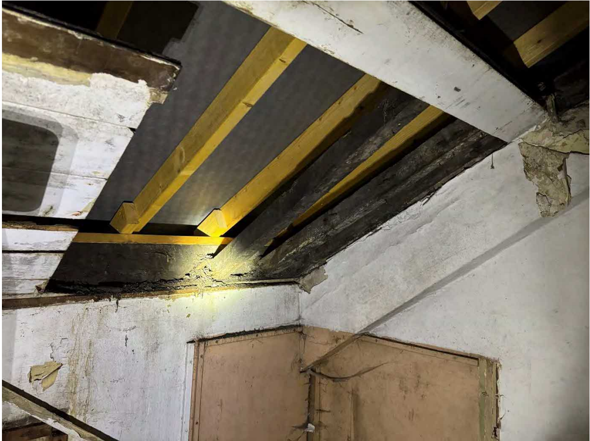
P45 – Recently installed timber rafters and roof membrane – supported on original timber roof structure. Rear roof slope.
