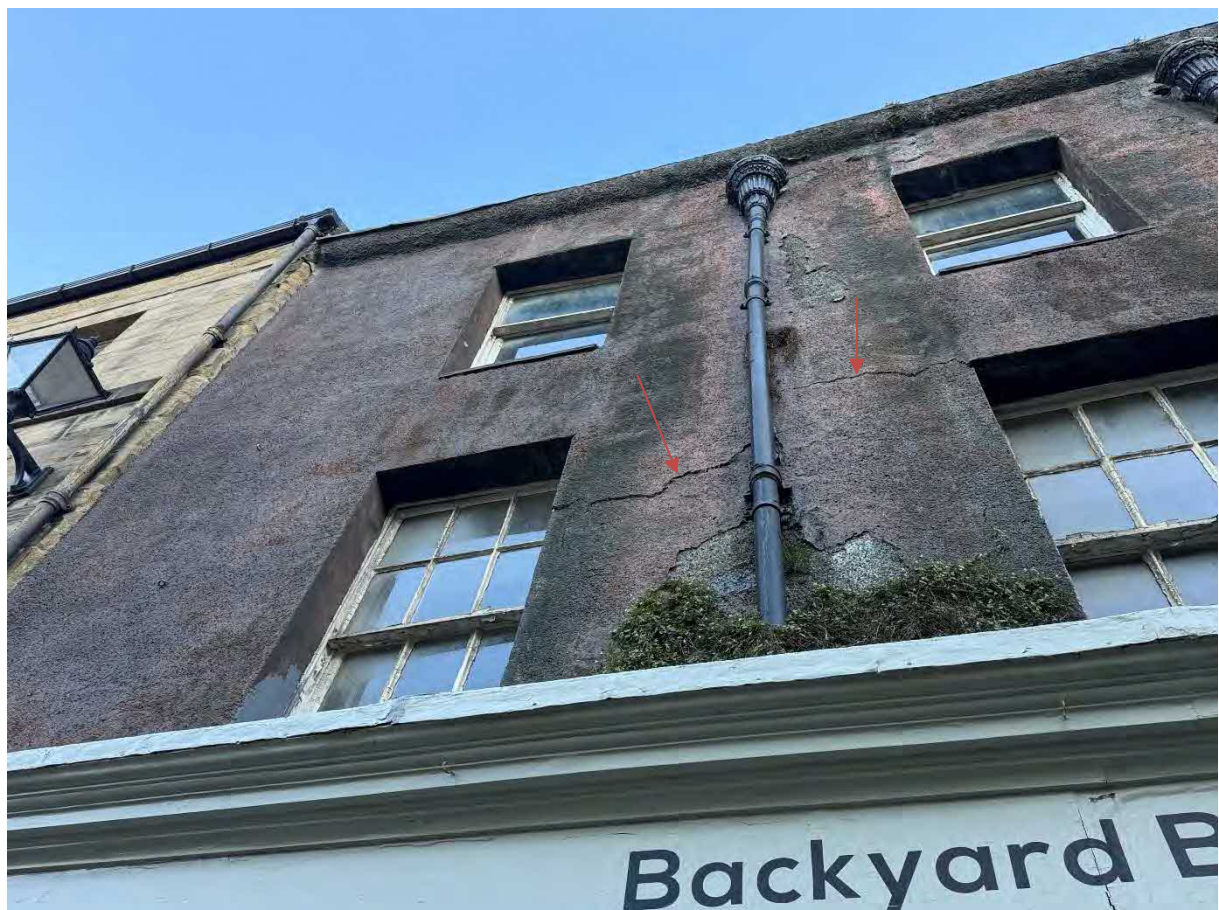
P12 – Cracking within first floor wall above defective shopfront beam. Defective roof rainwater drainage.
