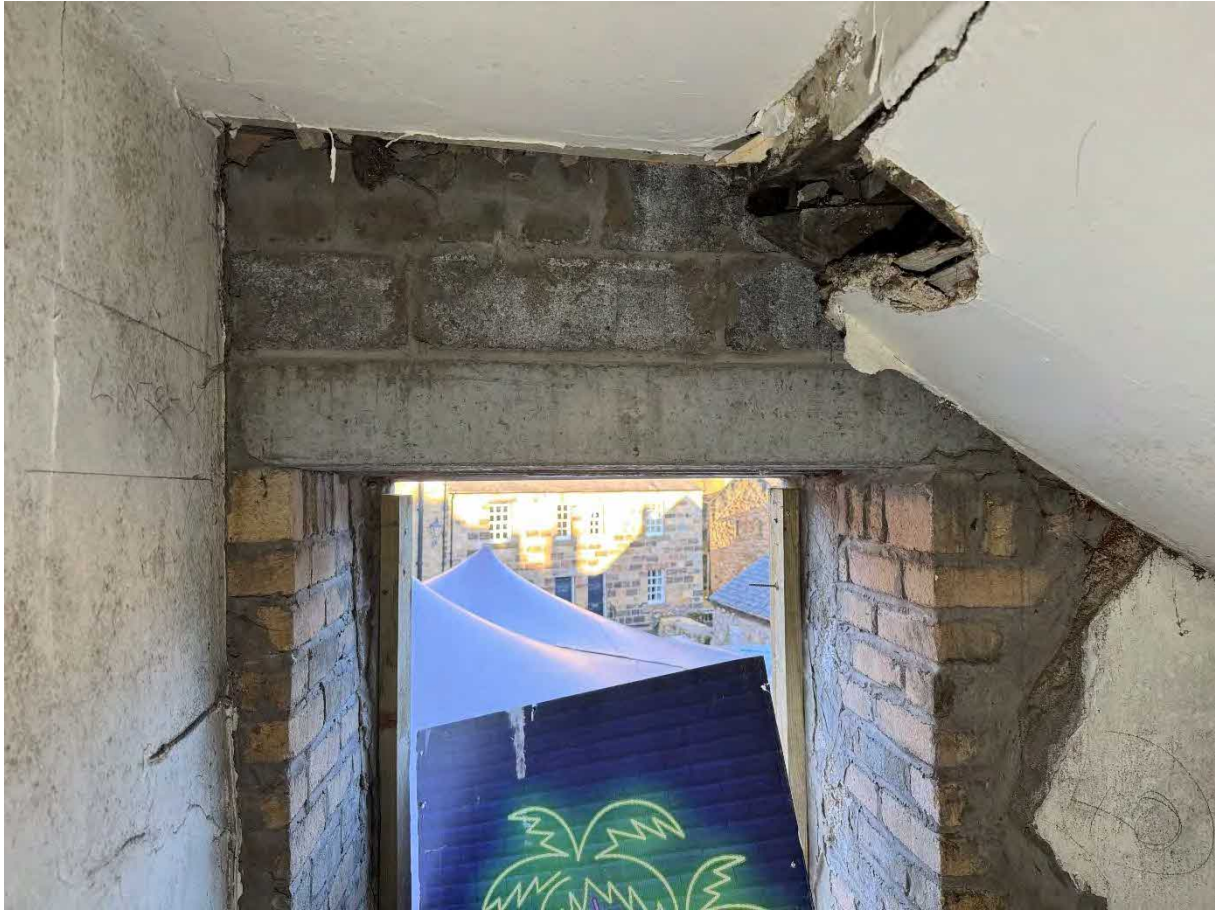
P49 – Recently replaced lintels forming opening within rear elevation wall. Internal timber staircase – first to second floor level (RHS) has poor alignment with evidence of timber decay.
