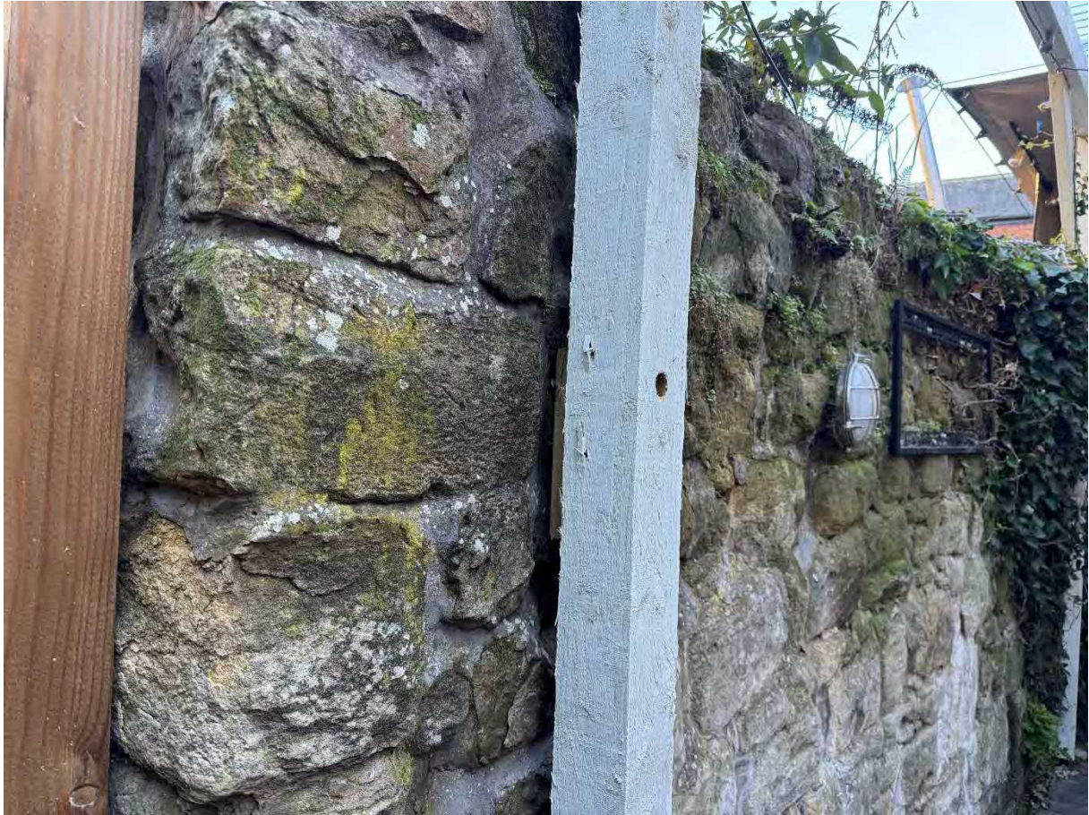
P63 – Timber framed pergola to rear beer garden. Rear posts bolted to rear stone boundary wall.
