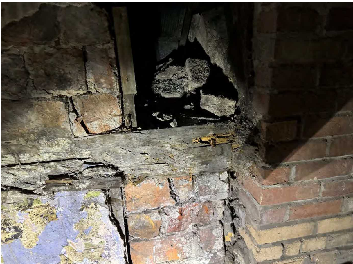
P34 – Loose masonry and decayed timber within wall at second floor landing.
