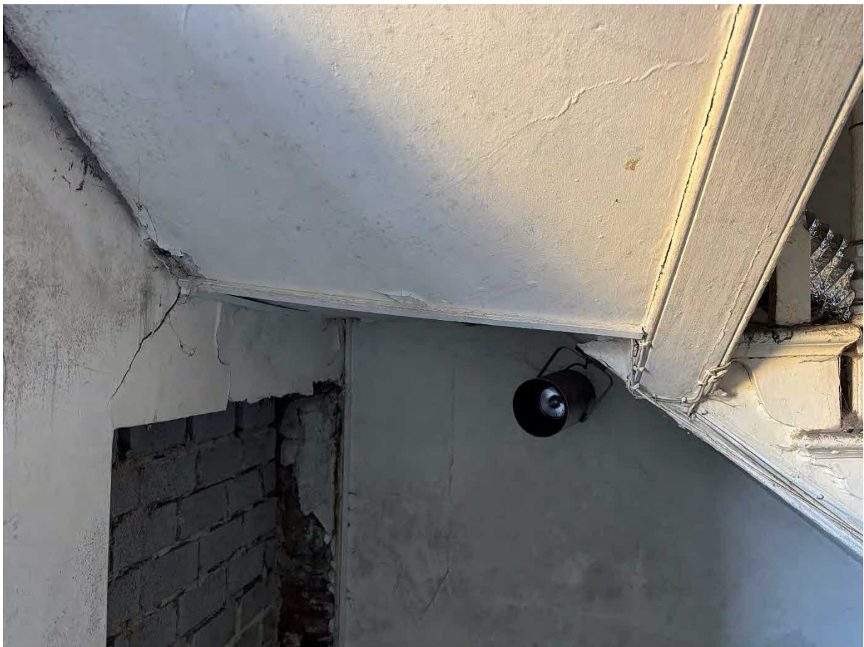
P48 – Internal timber staircase – ground to first floor level. Staircase has poor alignment.
