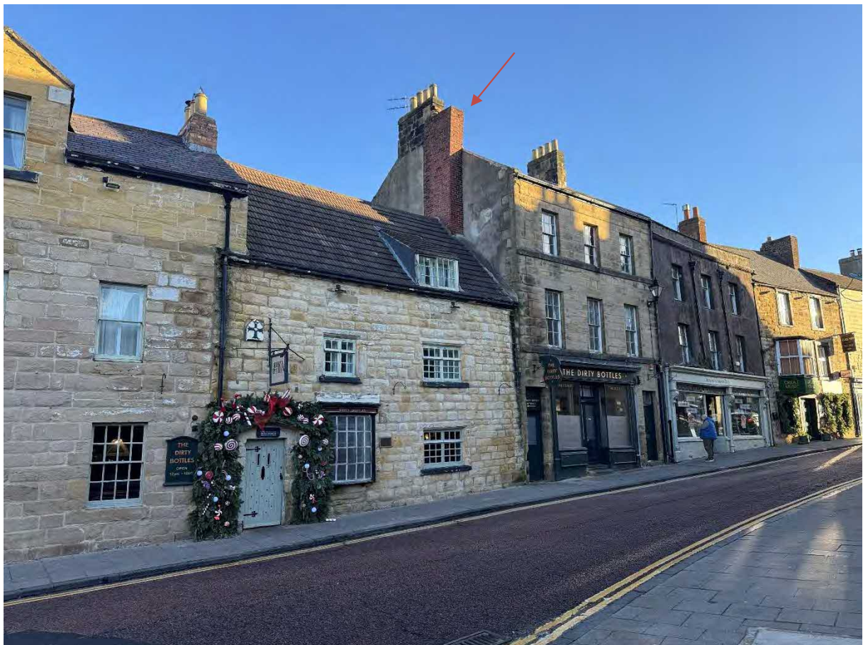
P4 – The Dirty Bottles – No. 28 - 32 Narrowgate - Alnwick - Front, southwest elevation. Red arrow highlighting chimney stack with poor vertical alignment.
