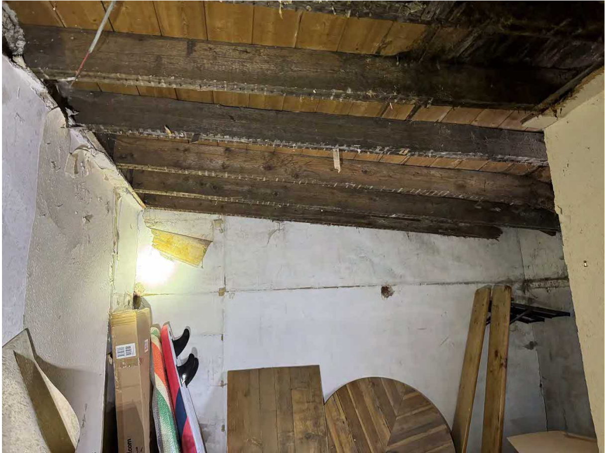
P29 – First floor level – front room (1). Second floor structure (over) has failed at bearing onto rear elevation wall. Second floor over has poor horizontal alignment and is unstable.
