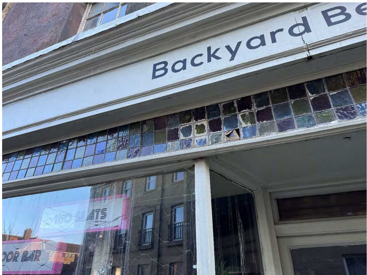
P11 – Deflection within shopfront beam above ground floor entrance with cracking to first floor wall and distortion and damage to shopfront fascia.
