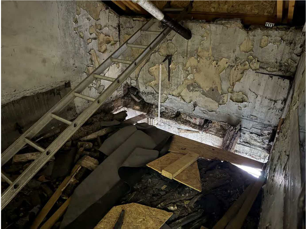
P35 – Second floor level – rear room (4). Second floor structure has failed at bearing onto rear elevation wall. Timber floor structure has poor horizontal alignment and is unstable.
