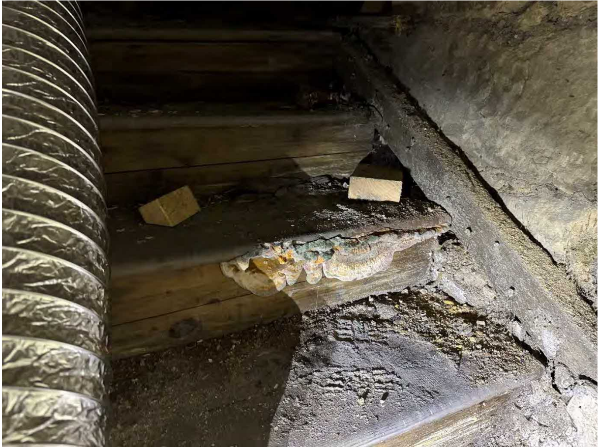
P51 – Dry rot (fruiting body) – timber staircase, first to second floor level.
