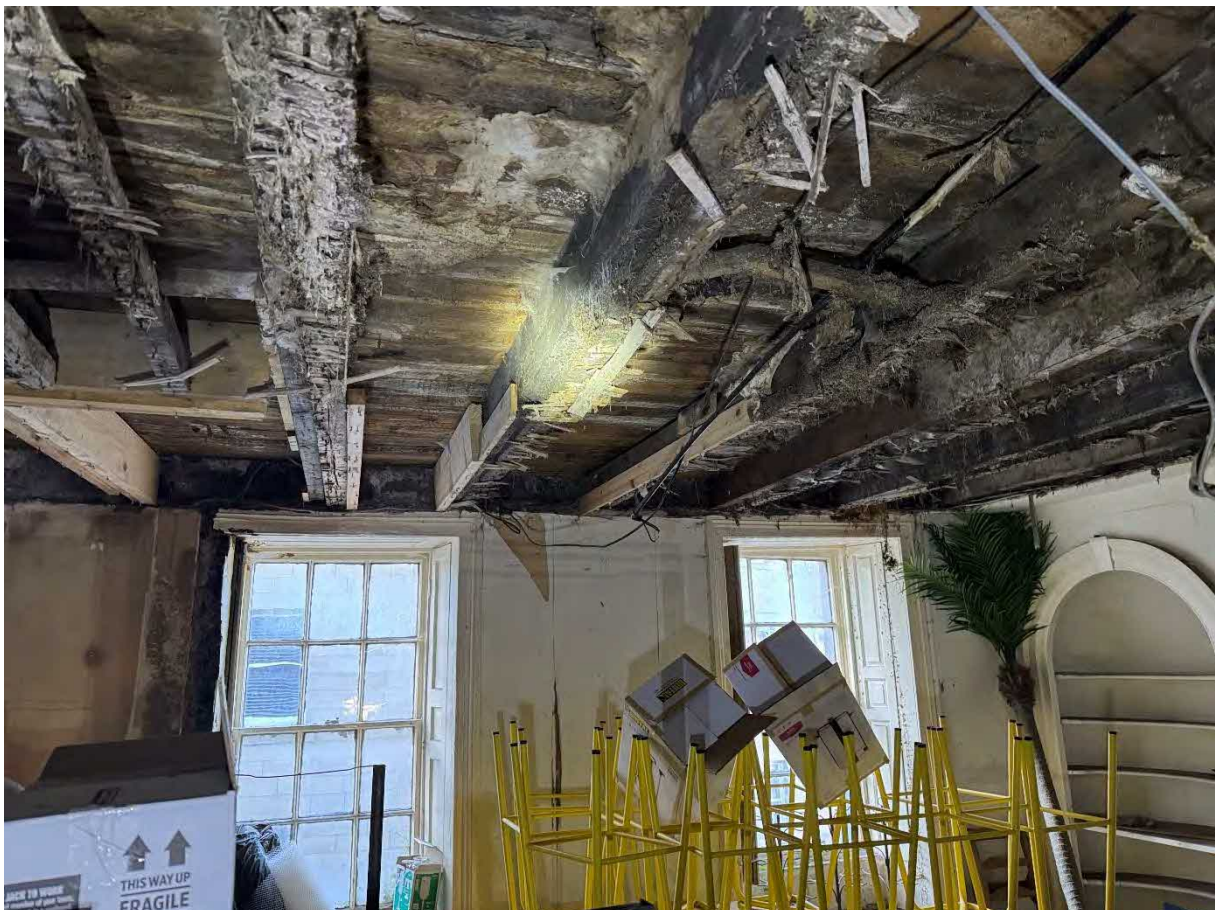
P26 – First floor level – front room (3). Severe decay (wet and dry rot) within timber second floor structure. Past modifications and repairs to second floor structure appear to have been poorly implemented and the floor is potentially unsafe.
