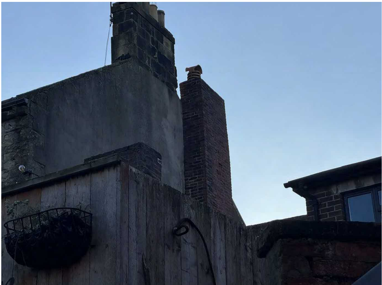
P52 – Chimney stack to party wall of 30-32 Narrowgate – viewed from rear. Chimney stack has poor vertical alignment, leaning out to east (estimate approx 100mm).
