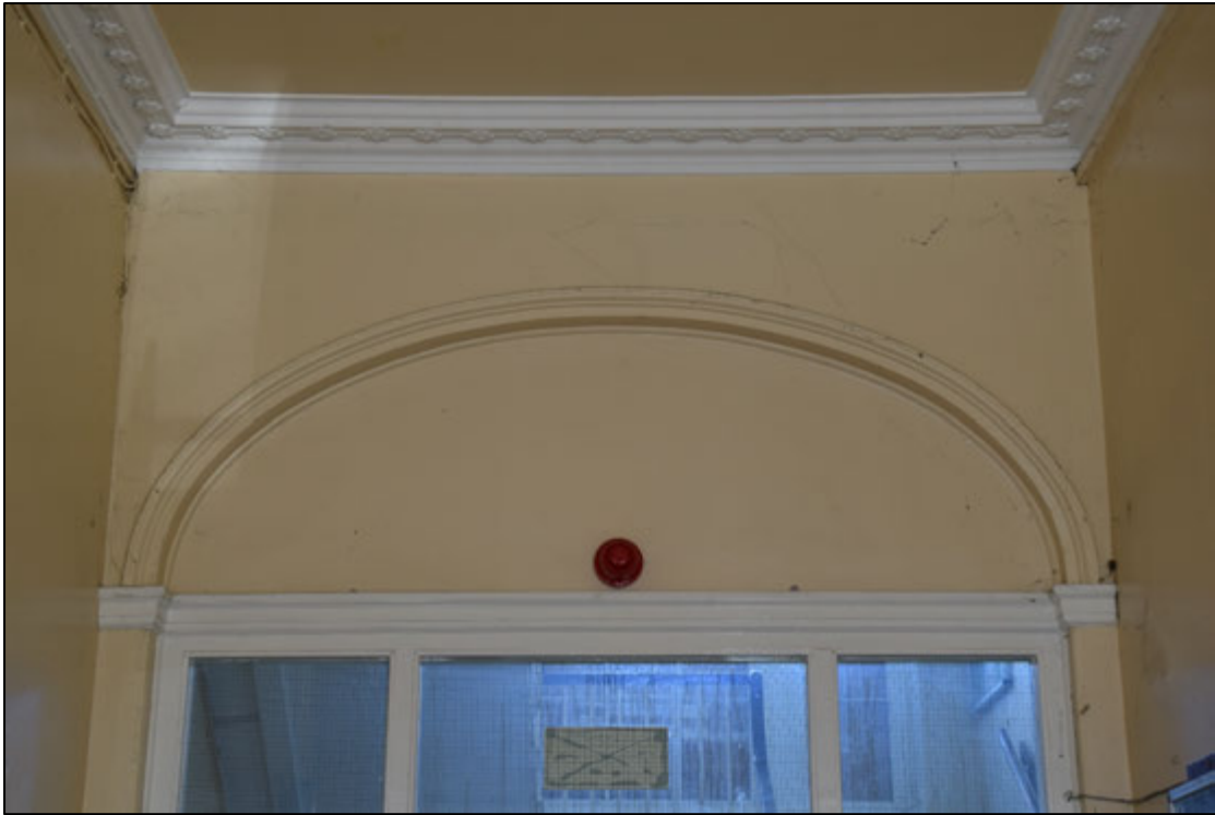
Photograph 71: Plaster arch and cornice at the north end of the hall [1]
