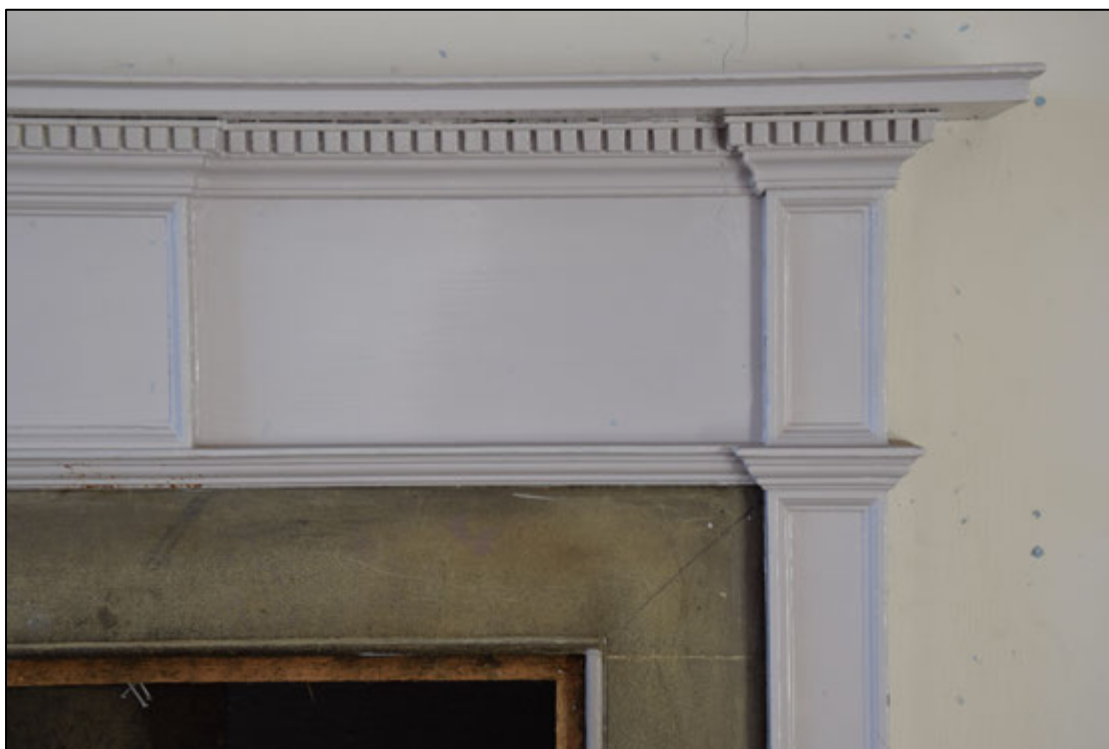
Photograph 114: Detail of the dentillated undermantel, plain frieze and sandstone slips in the fireplace of room [23]
