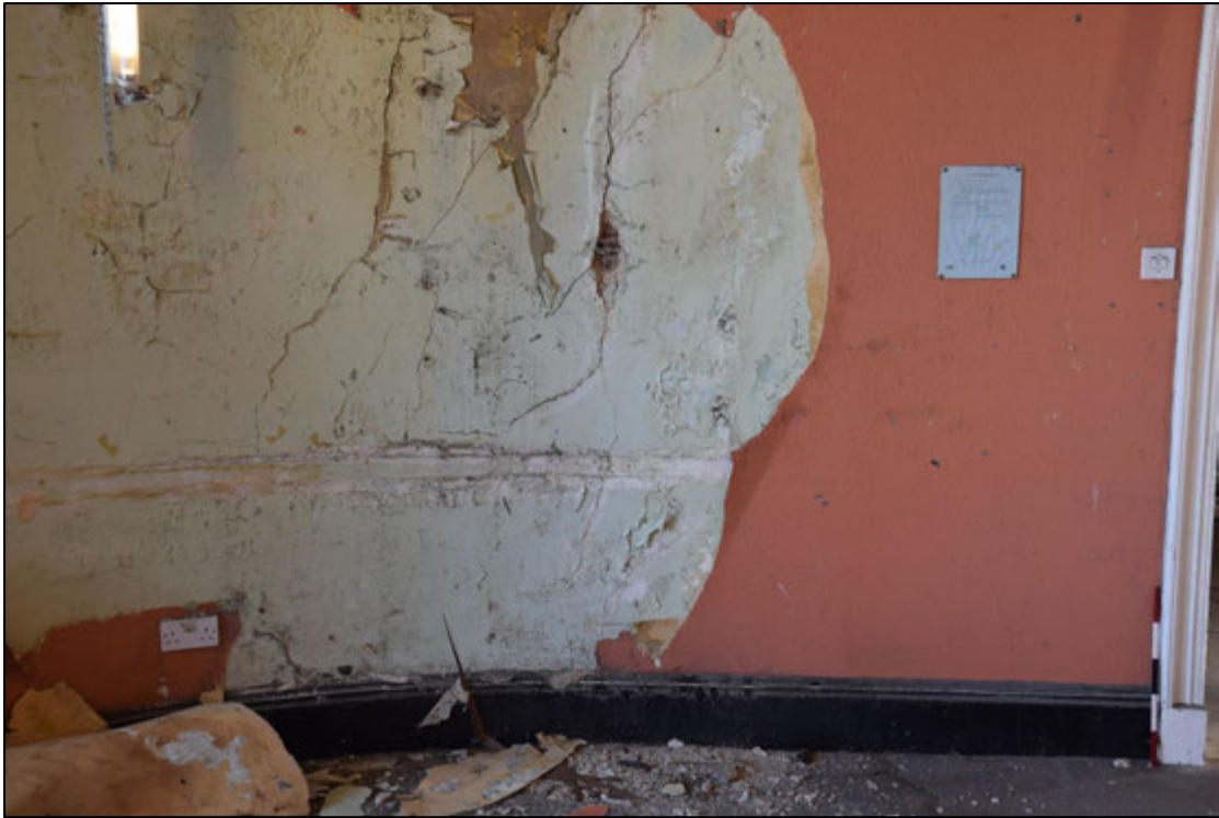
Photograph 199: A timber for a low dado rail in room [75]
