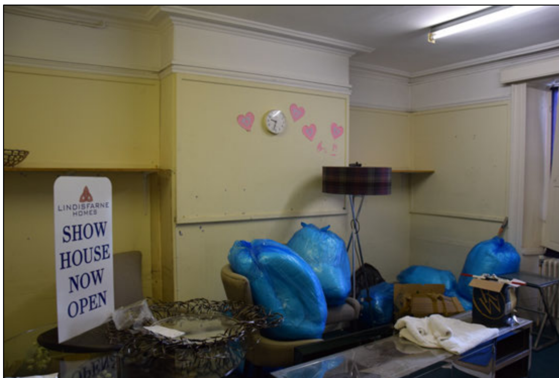
Photograph 141: The blind chimney breast, ceiling cornice and picture rail in room [35]
