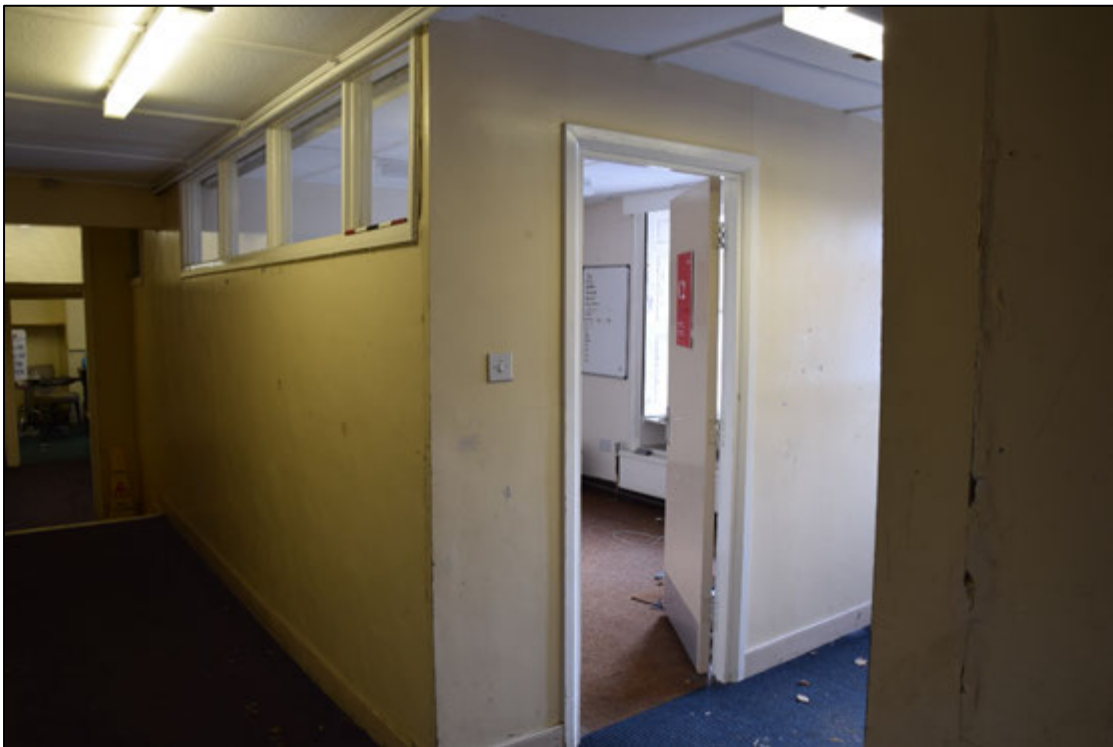
Photograph 178: A modern partition with borrowed lights forms the north wall of room [67]
