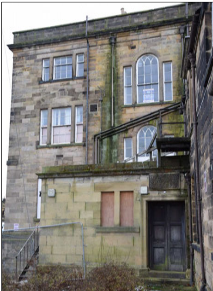
Photograph 48: The north face of no. 2, showing the Venetian windows on the stairs. In the foreground is the school entrance block, present in the 1920s. Design drawings show that the rough panel above the door was intended to carry the Duke's crescent badge
