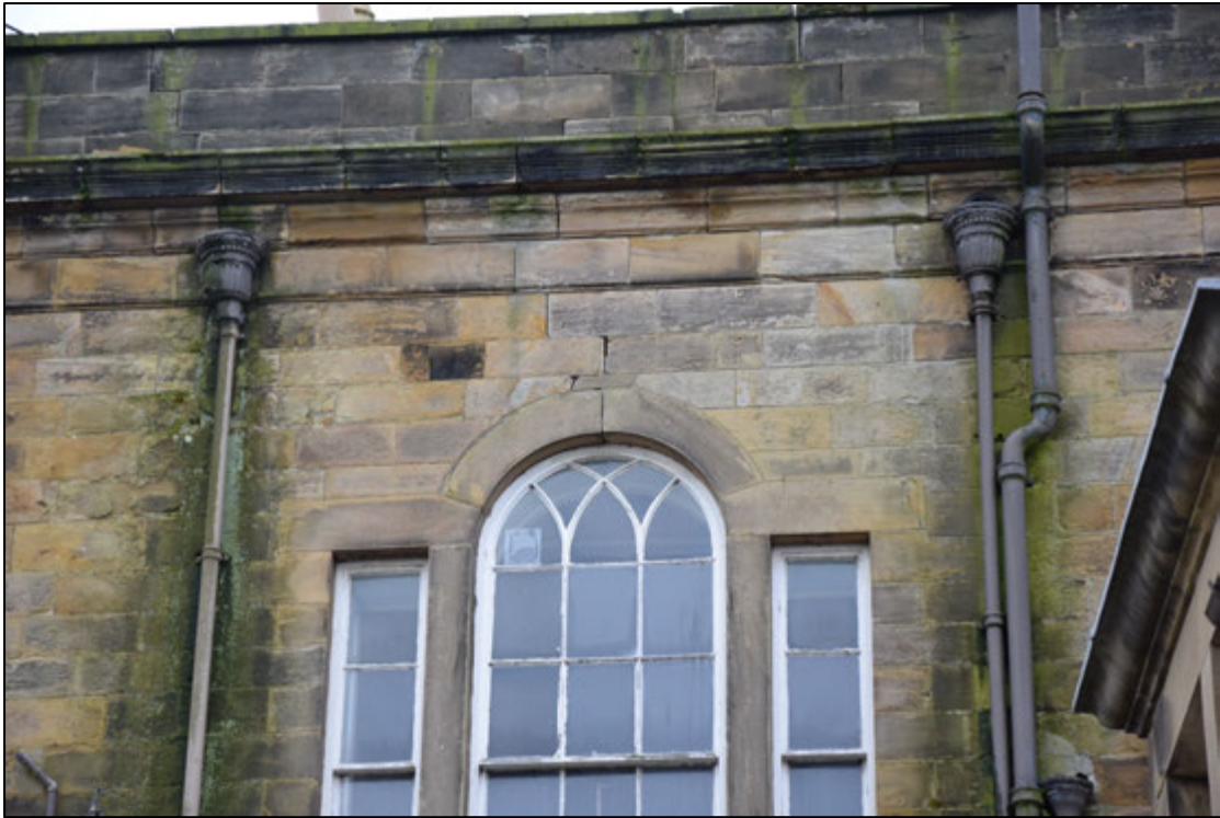
Photograph 49: Detail of the parapet, cornice, rainheads and upper stair window
