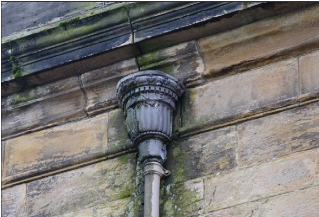
Photograph 50: The eastern rainhead. The lead inscription reads '17 DN 97'
