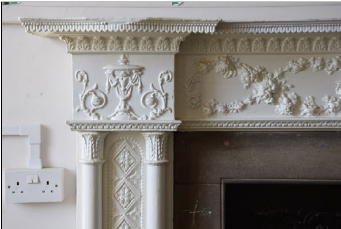
Photograph 80: Detail of the mantel, frieze and stone slips, with the heads of the columns
