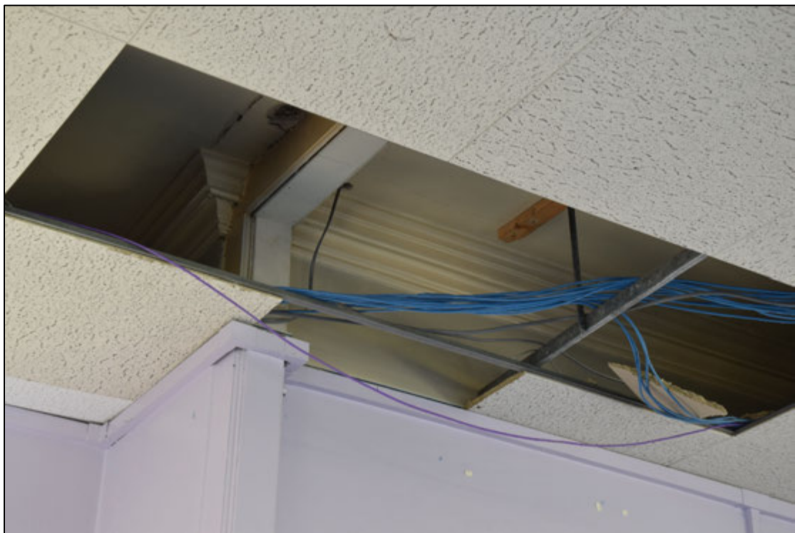
Photograph 120: The old ceiling cornice revealed above a modern suspended ceiling
