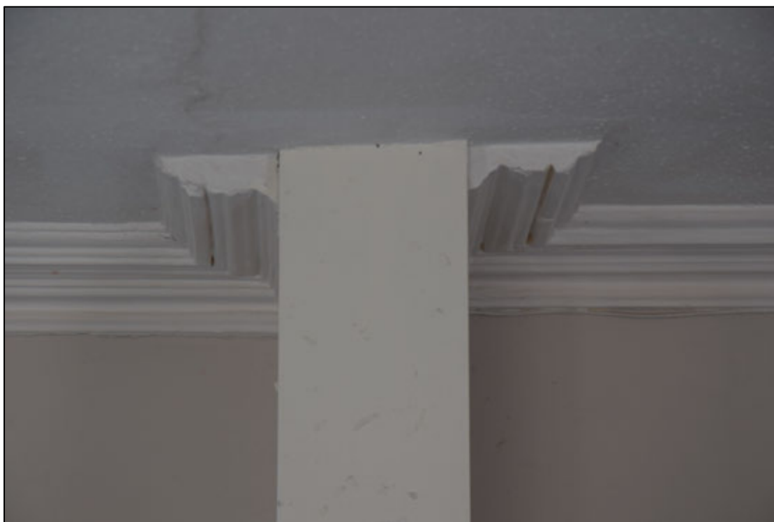
Photograph 172: The stub wall and cut cornices show how room [60] was created by removing an internal wall
