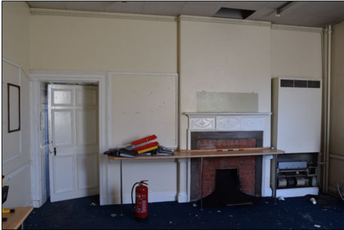
Photograph 89: The west wall of room [5], with modern brick filling an original fireplace
