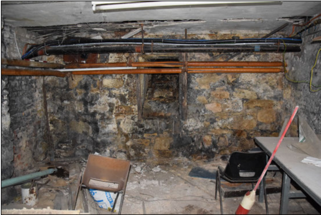
Photograph 159: The main cellar [52] in no. 4, with a coal chute and a projection (far left) for a chimney breast
