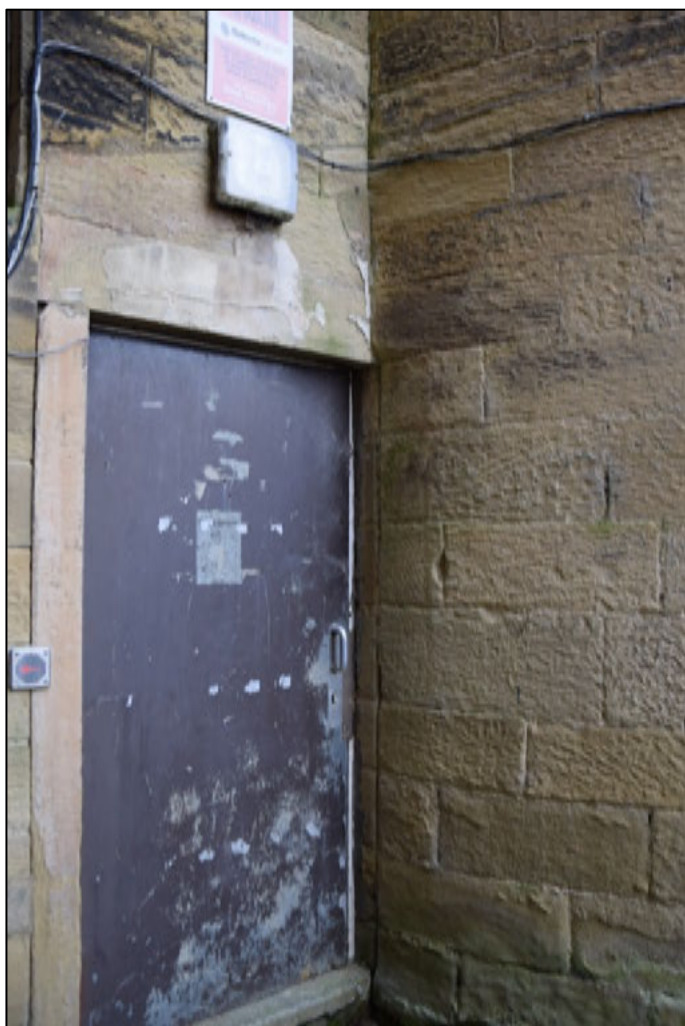
Photograph 67 (left): A straight joint can be seen between the north wall of no. 8 and the bow
