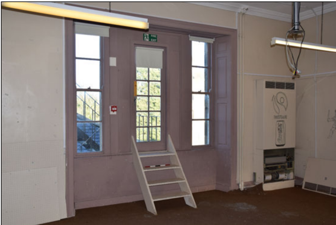
Photograph 112: The tripartite north window in [22], altered to make a fire escape
