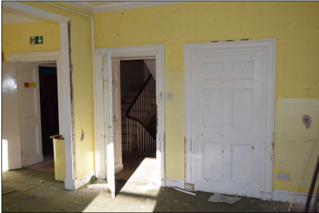
Photograph 163: Doors in the north wall of room [54], with the stub of the former internal wall. The right-hand door is fixed shut
