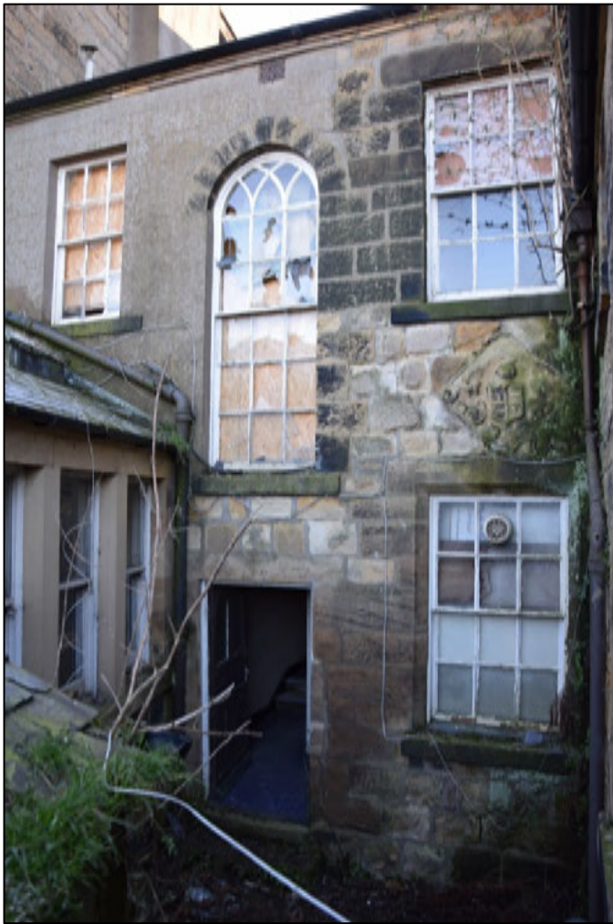
Photograph 55 (left): The back wall of no. 4 shows different stonework around the lower window that higher up; left of the tall window, the wall is rendered. Note the coat of arms above the lower window
