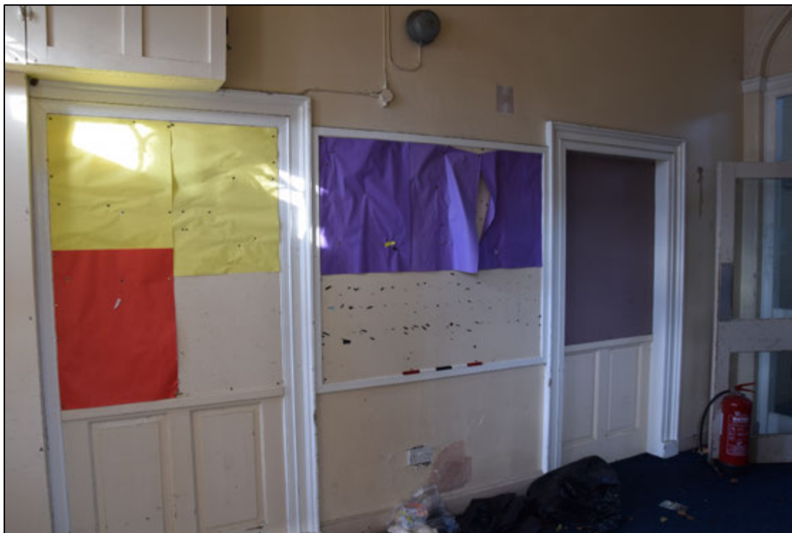
Photograph 69 (above): Doors on the west side of the hall [1]. That on the right gave access to room 3 and the other is a dummy used to create a symmetrical arrangement
