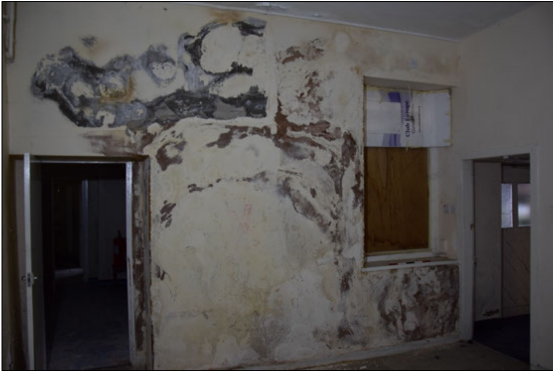
Photograph 143: Damaged modern plaster on the north wall of room [37]. The door at the extreme right leads to the enclosed yard
