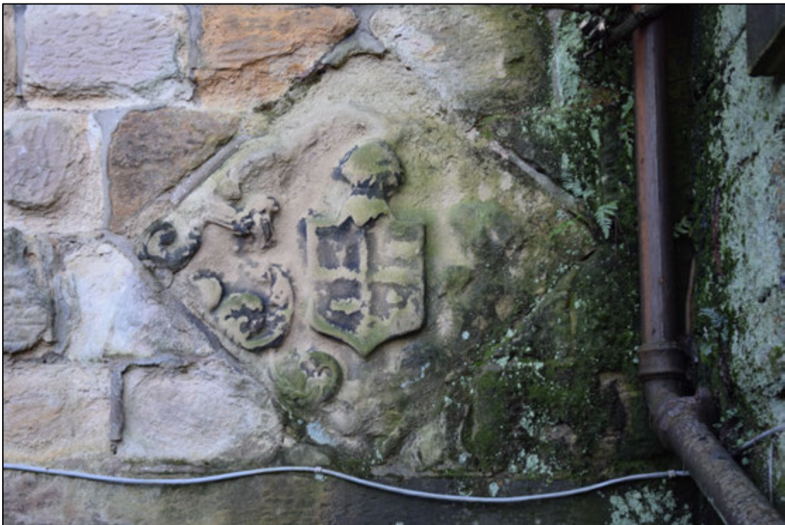
Photograph 58: The arms are so badly decayed that the coat cannot be identified
