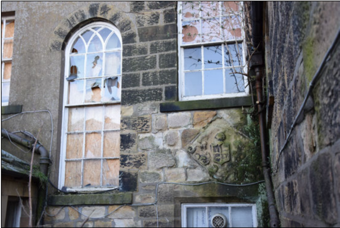
Photograph 57: Detail of the rear wall of no. 4, showing changes in stonework and the lozenge-shaped stone with the coat of arms
