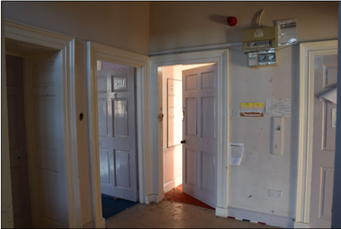
Photograph 109: Looking south-east across the first-floor landing of no. 2. The doors at the right show the change in thickness of the east wall here
