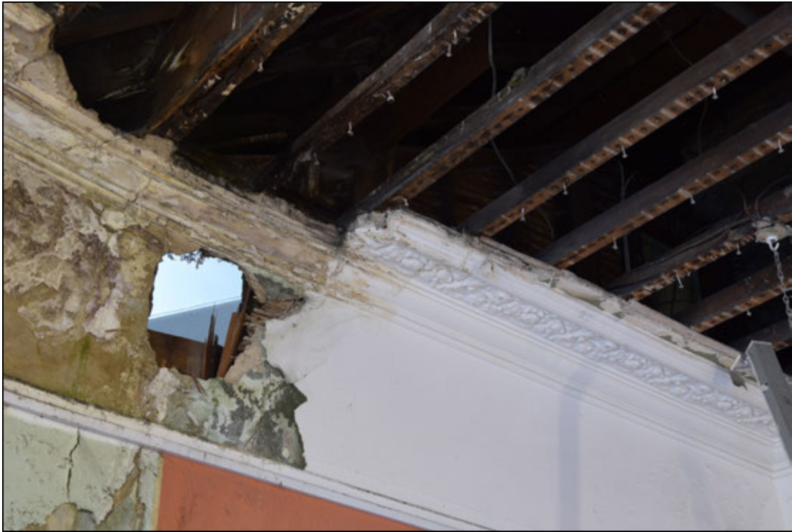
Photograph 197: Detail of the ceiling cornice and picture rail in [75]
