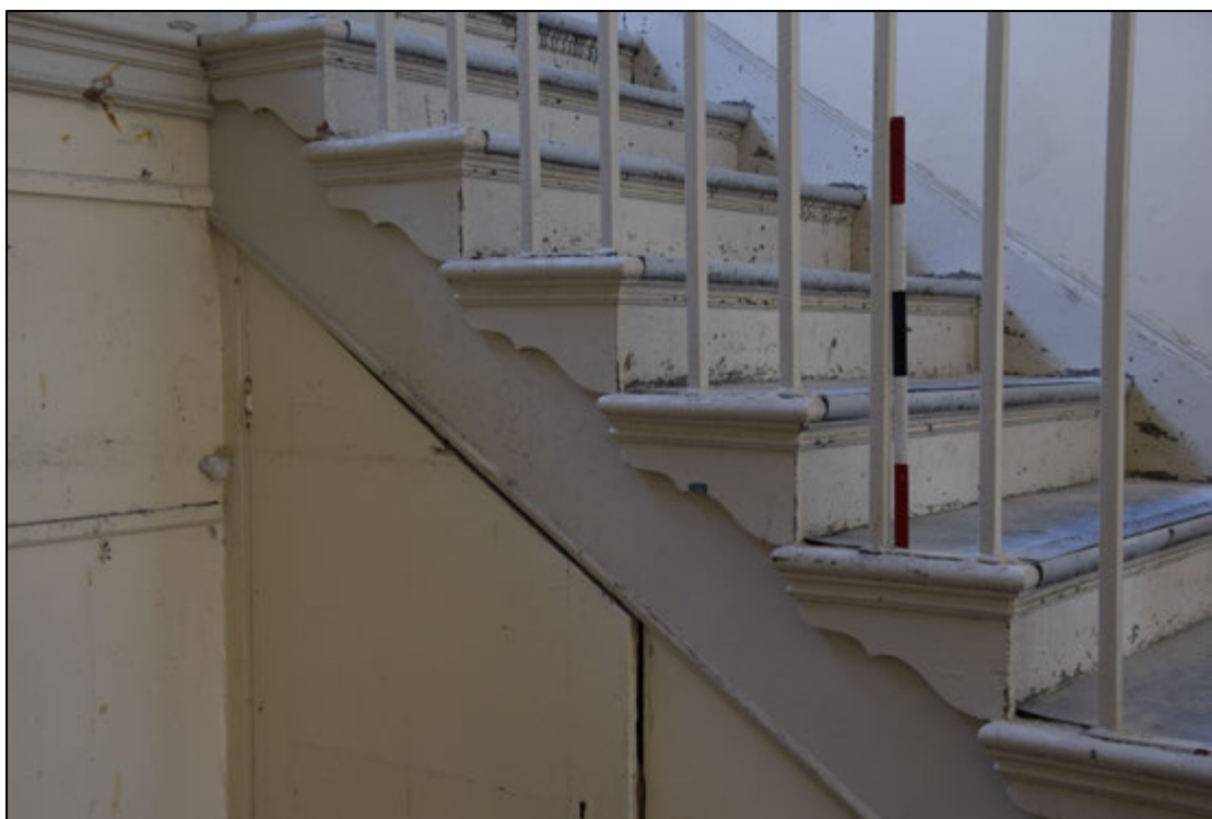
Photograph 73: Detail of the stairs [2]. The cupboard was removed when the stairs to the cellar were installed below this flight
