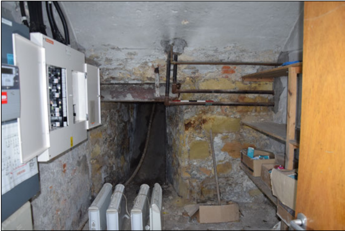
Photograph 107: A coal chute in the small cellar room [18]
