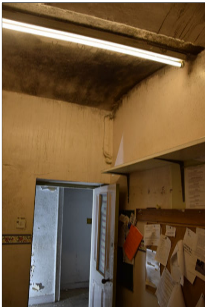
Photograph 95 (left): Jack arches in the ceiling of the cleaner's cupboard, room [9], with the passage [7] beyond
