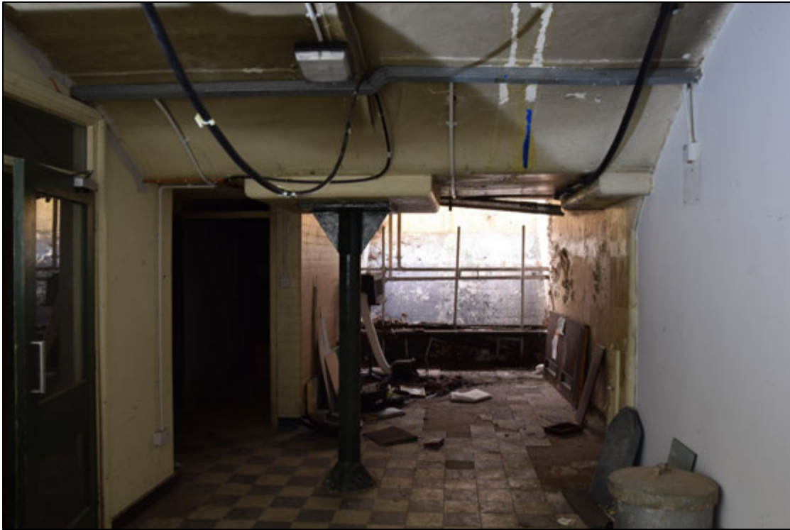
Photograph 99: Cellar room [12] with its pavement light and iron column, seen from the north end
