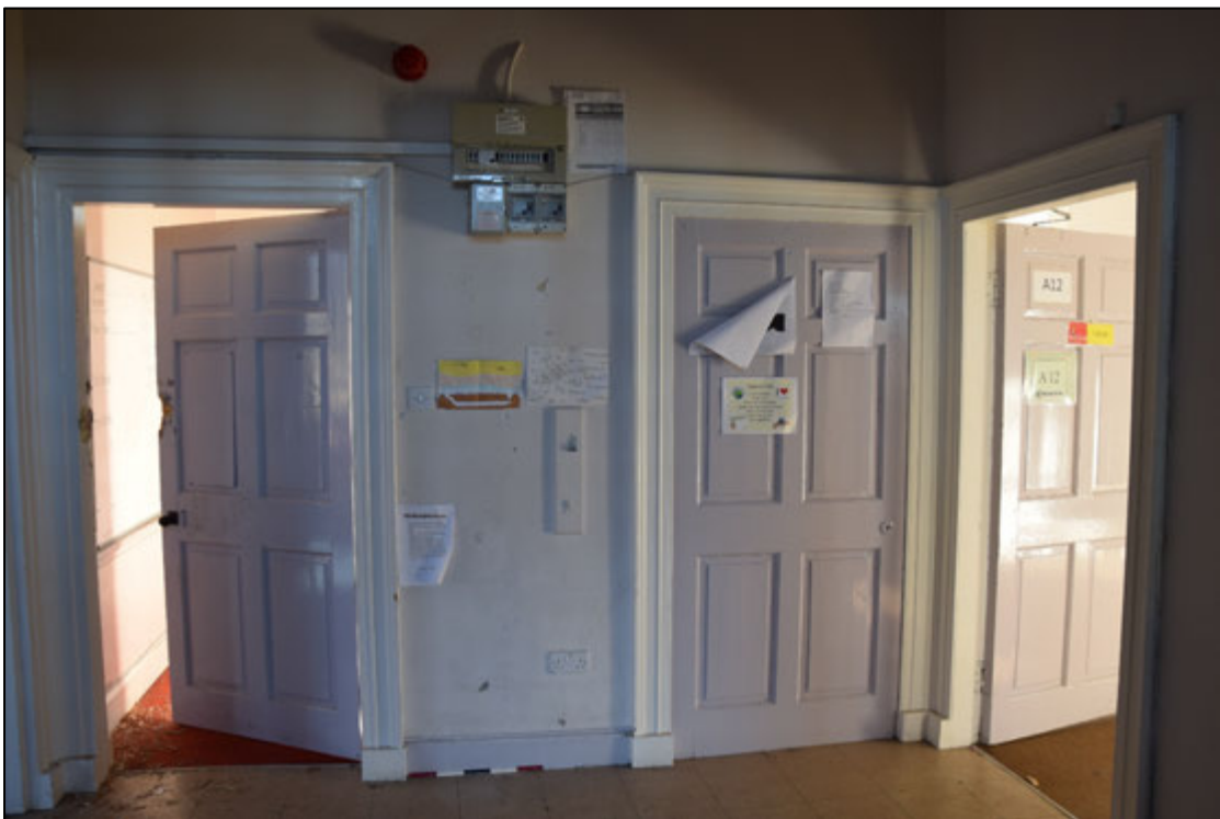
Photograph 110: Two doors on the south of the landing [21]; the right-hand one is a decorative dummy
