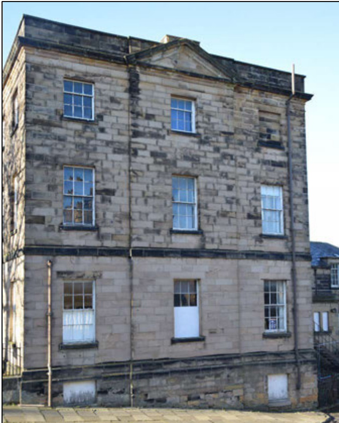
Photograph 47: The east face of no. 2. Note the boarded up windows to the cellar rooms 19 (left) and 17, and the blind second-floor window in room 32
