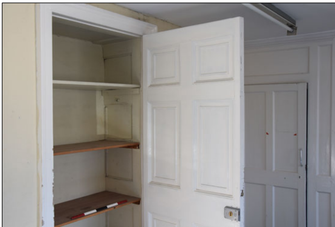
Photograph 206: Panelled lining of the altered door shown above
