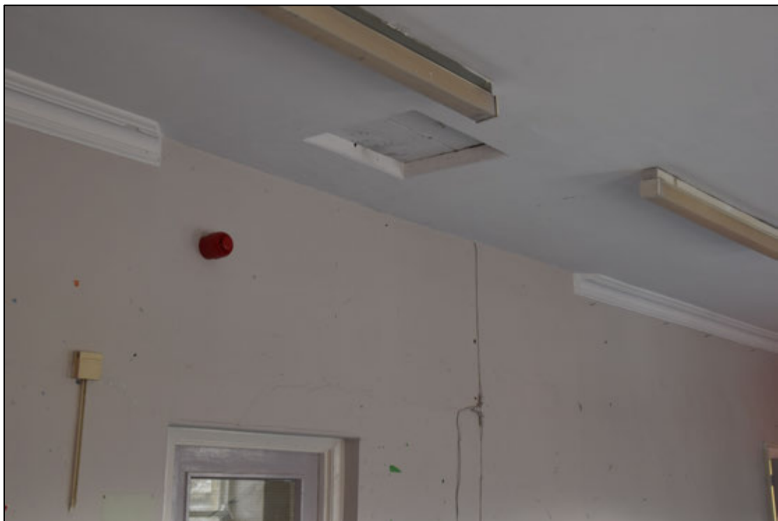
Photograph 214: The ceiling cornice in the north wall of [82] shows this was formerly three rooms, the centre one being narrow and plain
