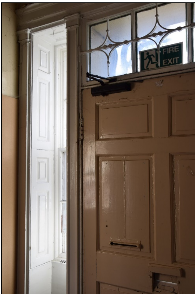
Photograph 69 (above): Doors on the west side of the hall [1]. That on the right gave access to room 3 and the other is a dummy used to create a symmetrical arrangement
