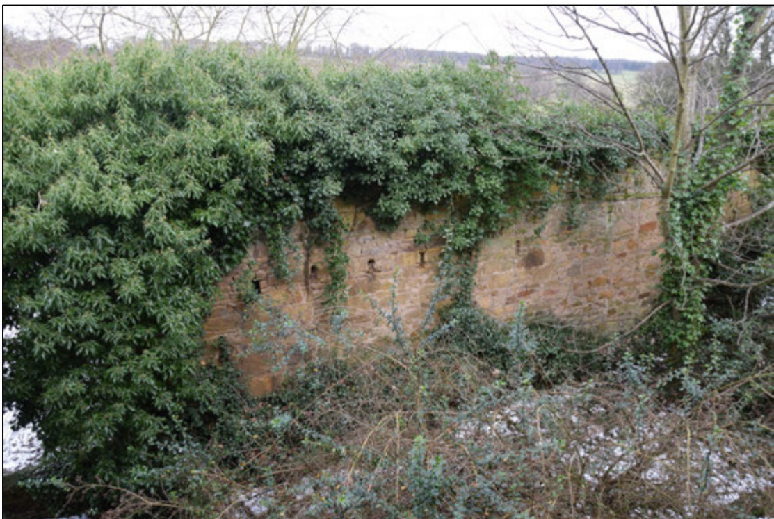
Photograph 226: Joist holes in the south wall of the old glasshouse, seen from the fire escape behind the gym
