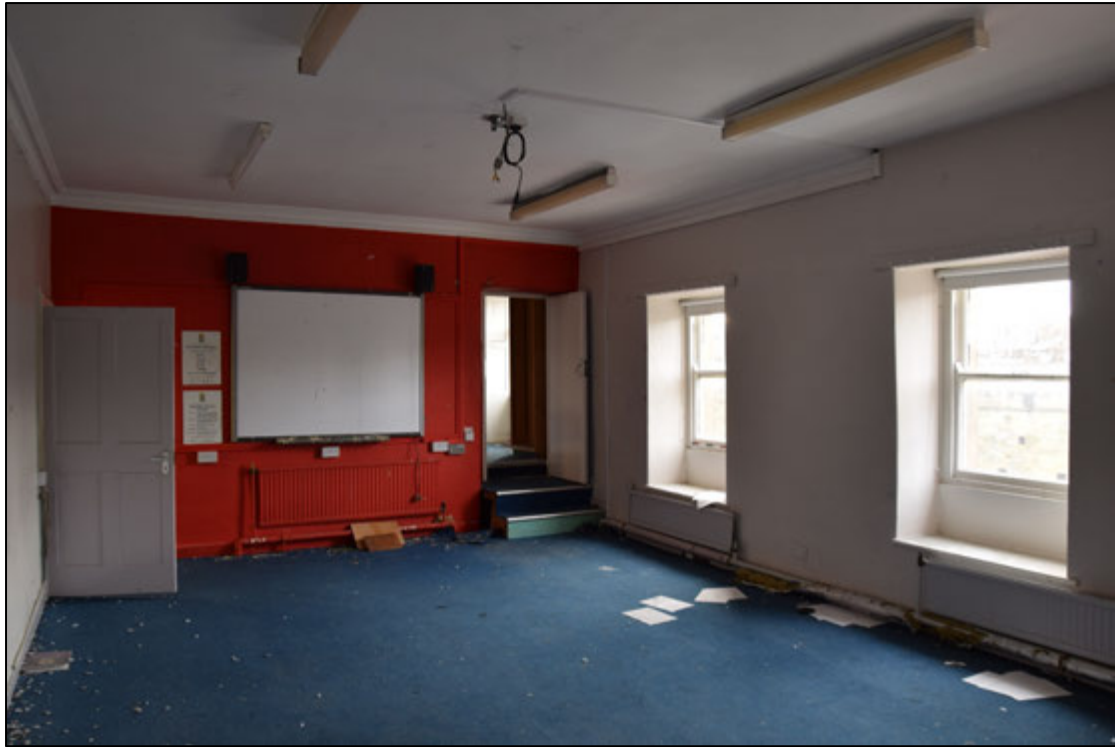
Photograph 213: The east end of room [82], with a modern door to the top floor of no. 4; note the disparity in floor levels here
