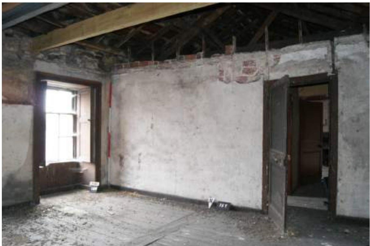
P118 (below). Room 34 looking south-east, showing door [157] leading from lobby Room 37, window [158], and on-edge brick-nogged stud partition. Scale 1m.
