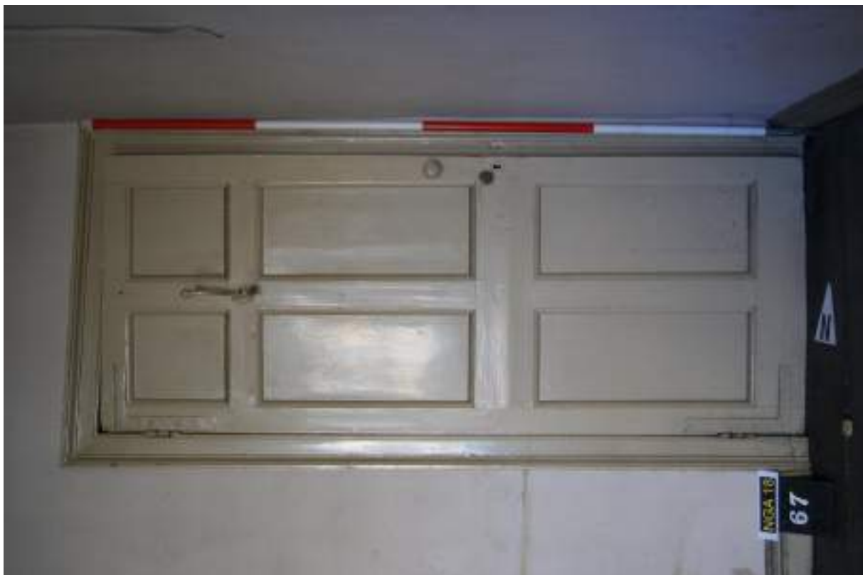
P68 (below). Room 4 showing door [67] formerly leading to passage Room 6.1, subsequently converted into a wall-cupboard. Scale 2m.
