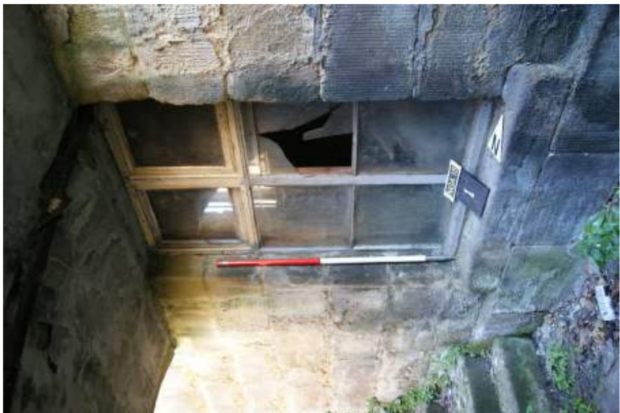
P25 (below). Basement window [1] showing renewed casements and offset plinth course, butted by the steps [200] to Narrowgate. Scale 1m.
