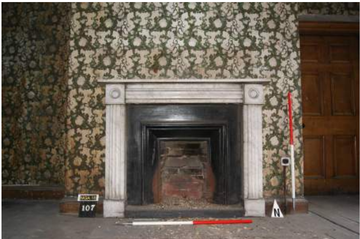
P92 (below). Room 17, late 18 th or early 19 th century fire [107] showing marble surround and wallpaper. Scales 1m.
