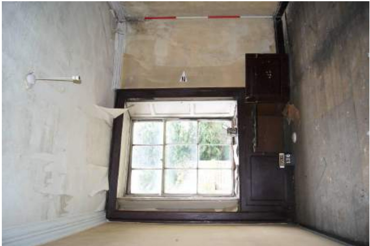
P89 (top). Room 13, looking west showing 3/6 sash window with storage below sill, and cornice to inserted south partition wall. Scale 2m.
