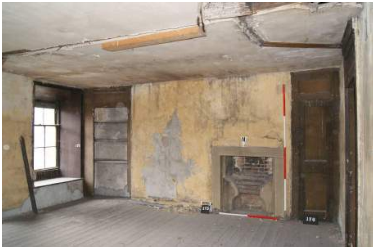
P124 (below). Room 38 looking south-east showing fire [175], door to wall-cupboard [176], window [172] to left and scar of a former partition in ceiling soffit. Scales 1m and 2m.
