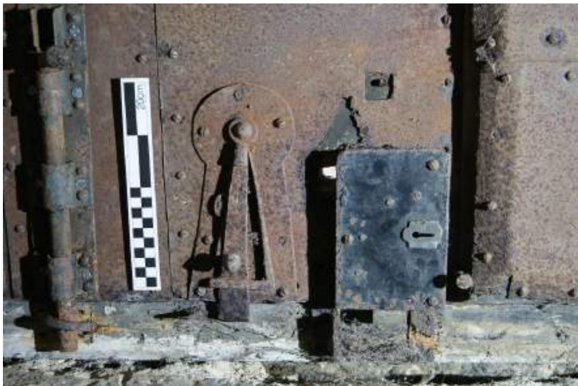
P33. Room 25. Detail of door [8] showing a spring catch of a form known from the 1820s. Later iron-cased lock below. Scale 20cm.
