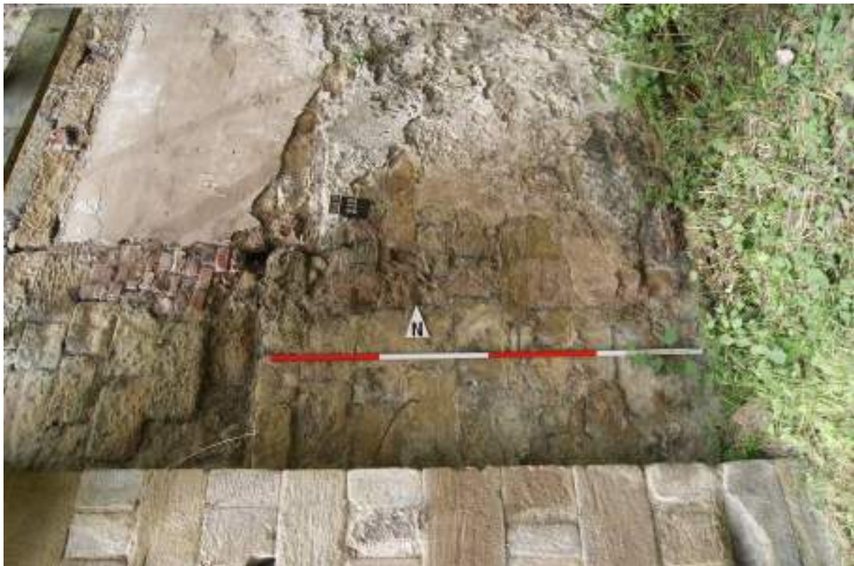
P17 (below). Interior of the coach-house looking west, with west jamb of the entrance (left), showing brick patching [212] in the west wall, and remains of plaster render. Scale 2m. NGA2/023
