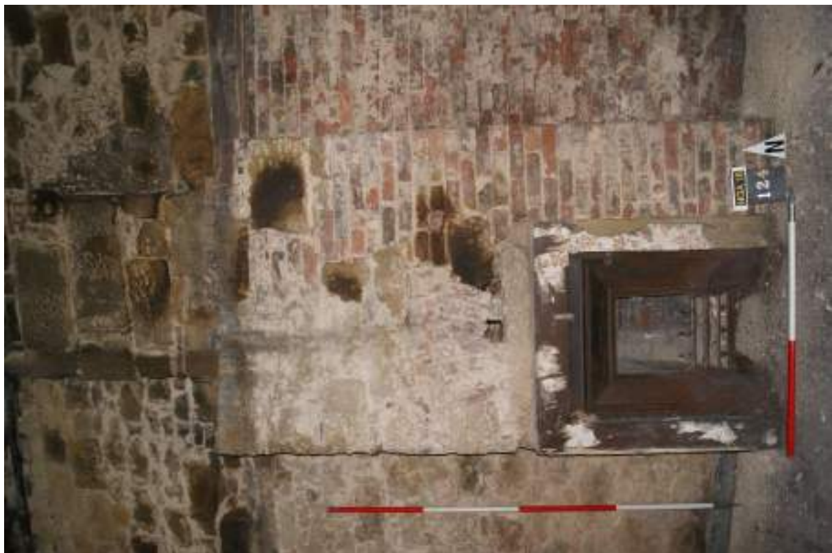
P106 (below). Room 20, detail of fire [124] in a patched brick and masonry breast, with brick north wall behind rising to sandstone rubble. Scales 1m and 2m.
