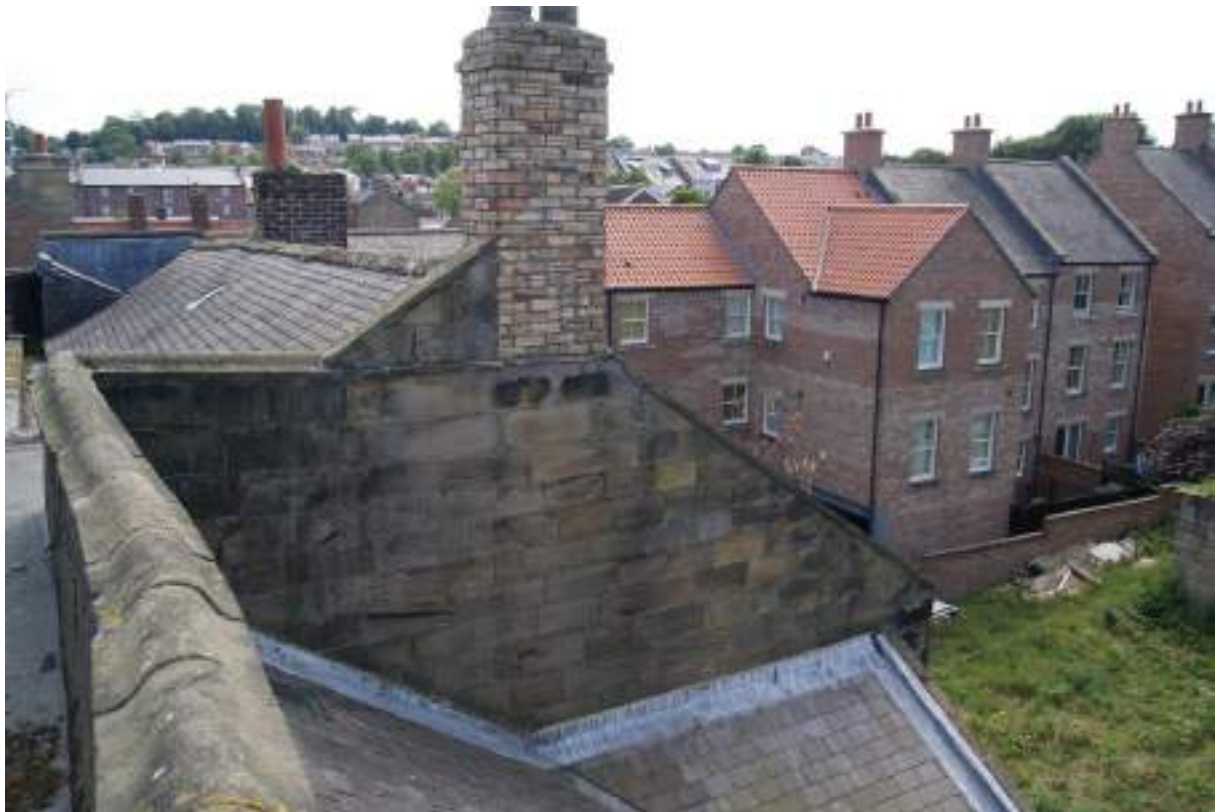
P132 (top). The western parapet looking south-east, showing deflection in the stonework, chimney [191] and junction of the parapet with the ashlar facing of the western extension. No scale.
