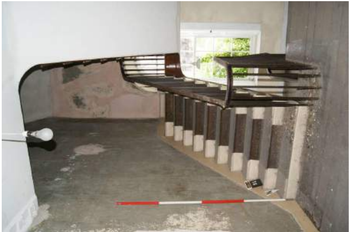
P81 (top). Room 8, looking south-west to the third flight of the principal stairs [91] showing bannister, balusters, and areas of modern plaster patching. Window [92] in background. Scale 2m.
