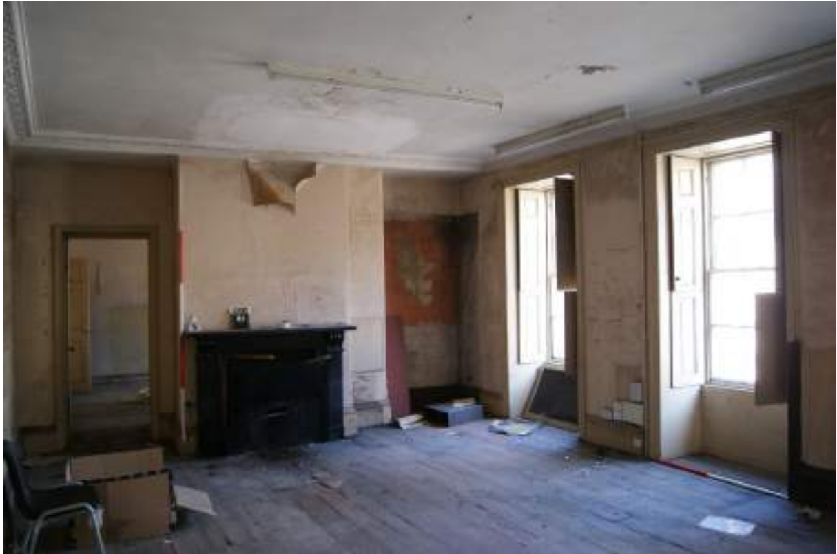
P61 (top). Room 3 looking north-east showing fire [61], door [62] to Room 4 on its left, alcove [60] to the right, windows [58] and [59], and decorative cornice. Scales 1m and 2m.
