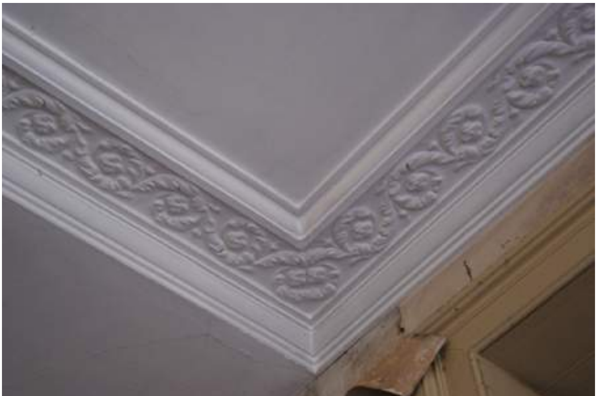
P64 (below. Room 3, north-east corner of ceiling showing cornice and frieze running across alcove [60]. No scale.
