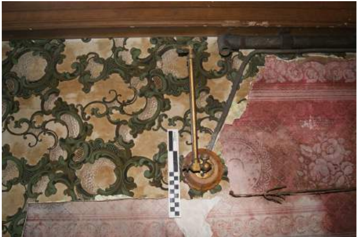
P97 (top). Room 17, gilt-brass swinging-arm gas-light fitting [196] between windows [105] and [106]. Scale 20cm.
