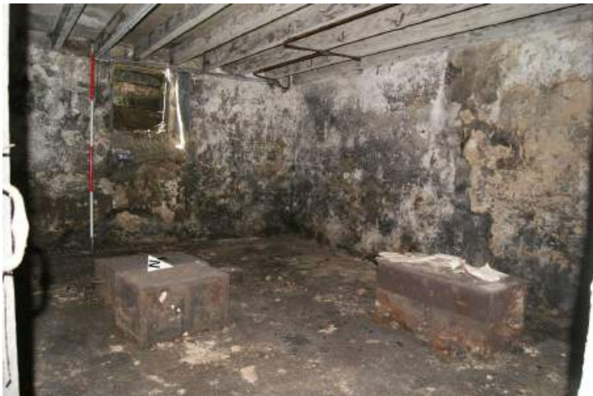
P43. Room 27 looking north-west, showing lightwell opening [34], sawn joists to 1st floor, and cast-iron safes. Scale 2m.
