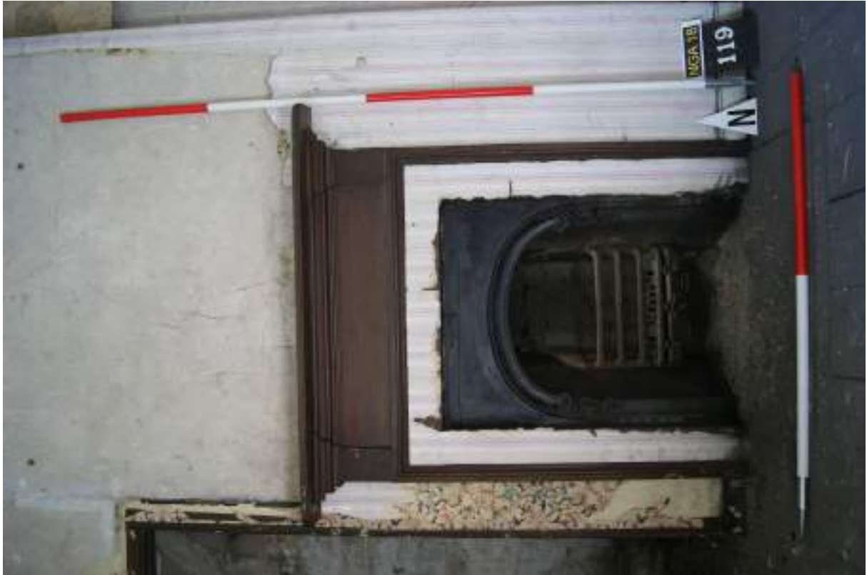
P103 (top). Room 19, fire [119] showing arch plate, grate, and timber overmantle. Scales 1m and 2m.
