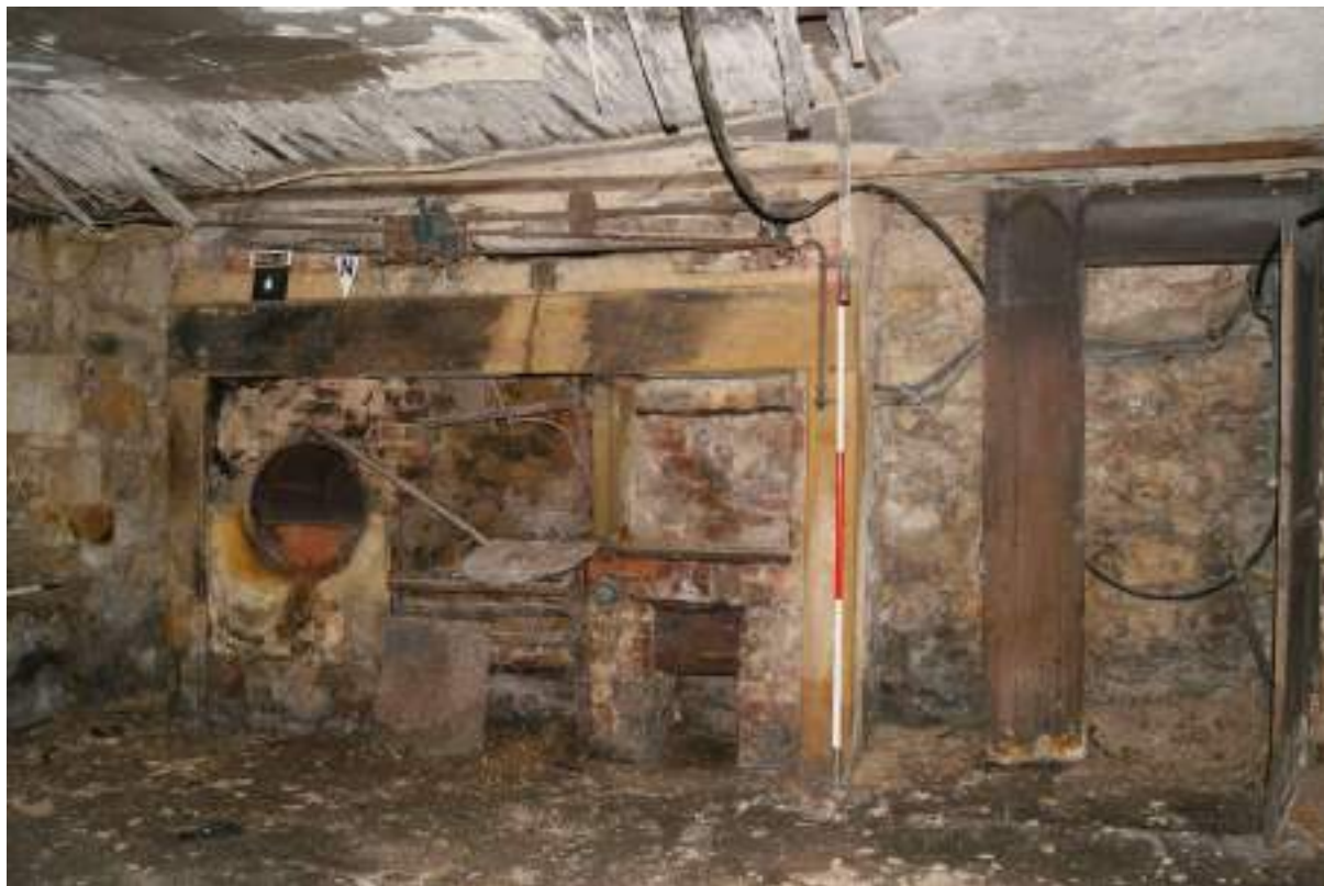
P29. Room 22 looking south-east, showing range [4] with oven, pot-crane, and boiler, and cupboard [5] on the right. Lath and plaster ceiling collapsing. Scale 2m.
