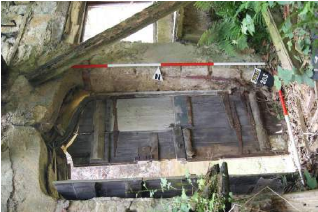
P6 (top). Stables: interior looking south-west to the inner face of the stable door [203] showing two-section door leaf with hinges and bolts and inner face of ogee lintel. Scales 1m and 2m. NGA2/010
