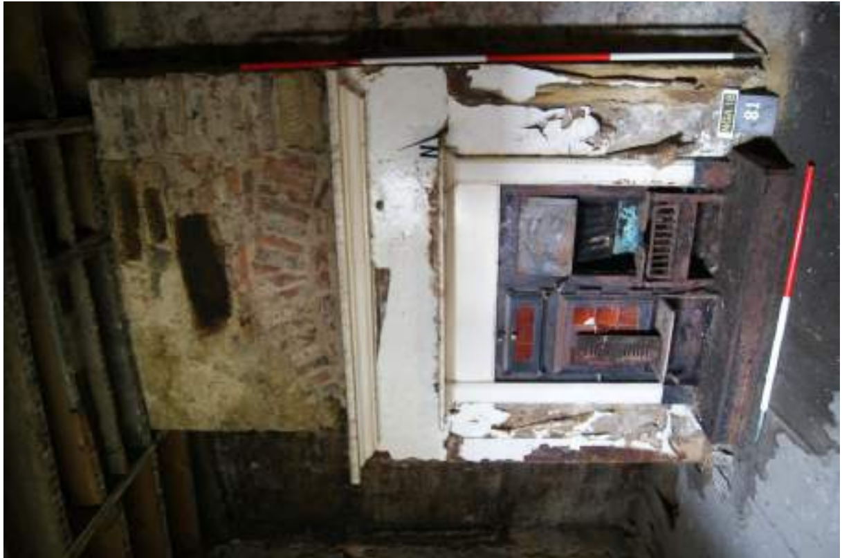
P77 (top). Room 15c, north wall showing detail of range [81] with earlier brick and stoned chimney breast above. Scales 1m and 2m.
