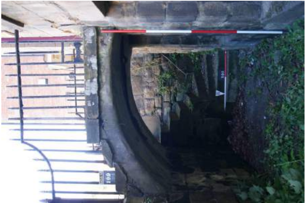
P24 (top). The 'flying' stairs to the front door of No.31 showing railings and boot-scraper, with steps from basement forecourt to street behind. Scales 1m and 2m.
