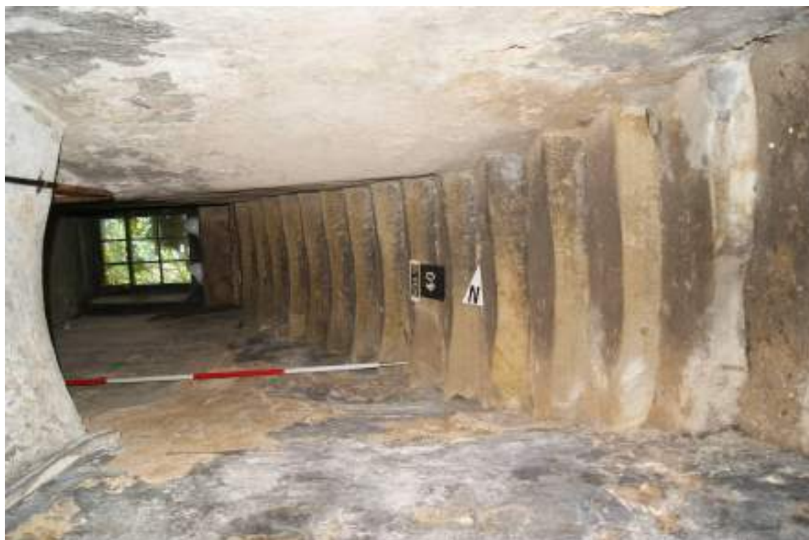
P44. Room 26, looking west up steps [40], showing worn treads, edge of vaulted brick ceiling, and kink in the south side of stair passage. Window [46] visible at the top. Scale 2m.
