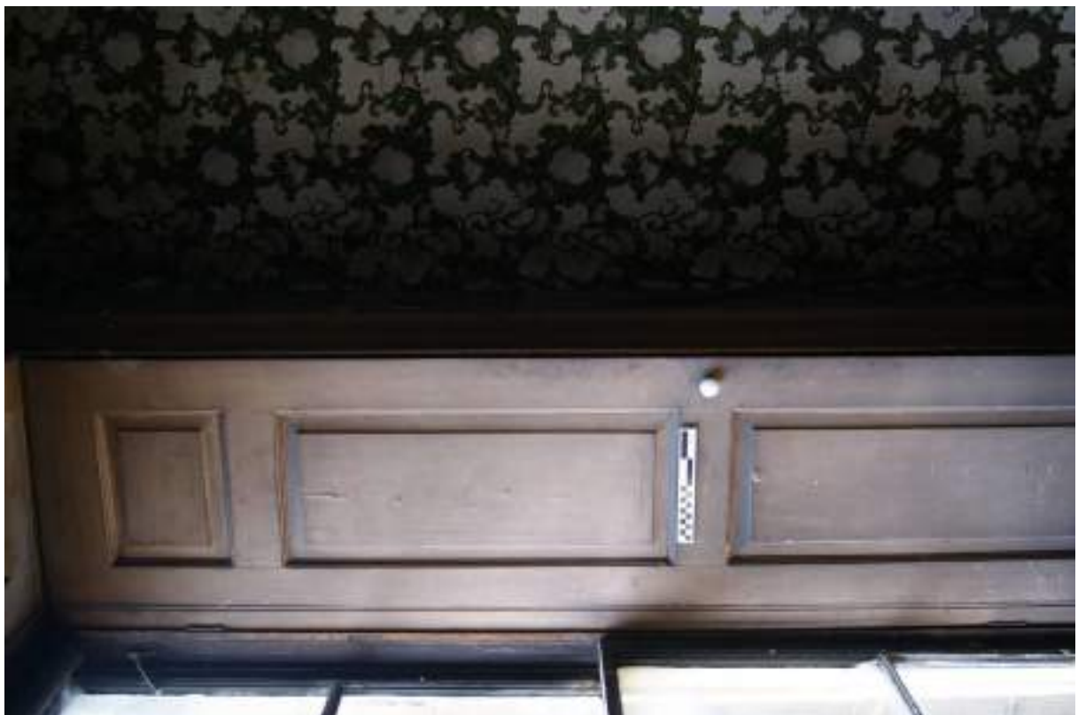
P96 (below). Room 17, southern shutter to window [104] showing (faintly) stencilled decoration to the raised and fielded panels. Scale 20cm.
