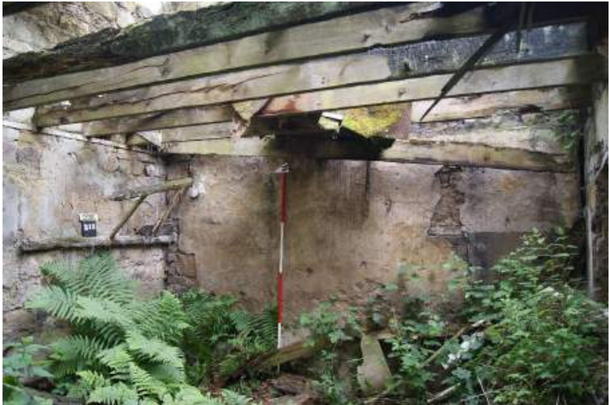
P8 (top). Stables interior looking north-east, showing east partition and butt joints with outer walls, remains of manger (left) and fallen/collapsing joists. Scale 2m. NGA2/011
