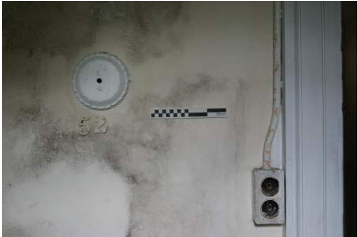
P55 (top). Room 8/9, east wall, north of door [45], showing a decorative wooden gas-light mounting [52] and late 1950s-early 1960s electric light switches and ducting. Scale 20cm.
