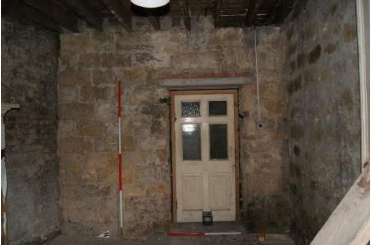
P75 (top). Room 15c looking east to door [181], showing butt joint between west and north walls, and ceiling joists exposed by removal of lath and plaster soffit. Scales 1n and 2m.
