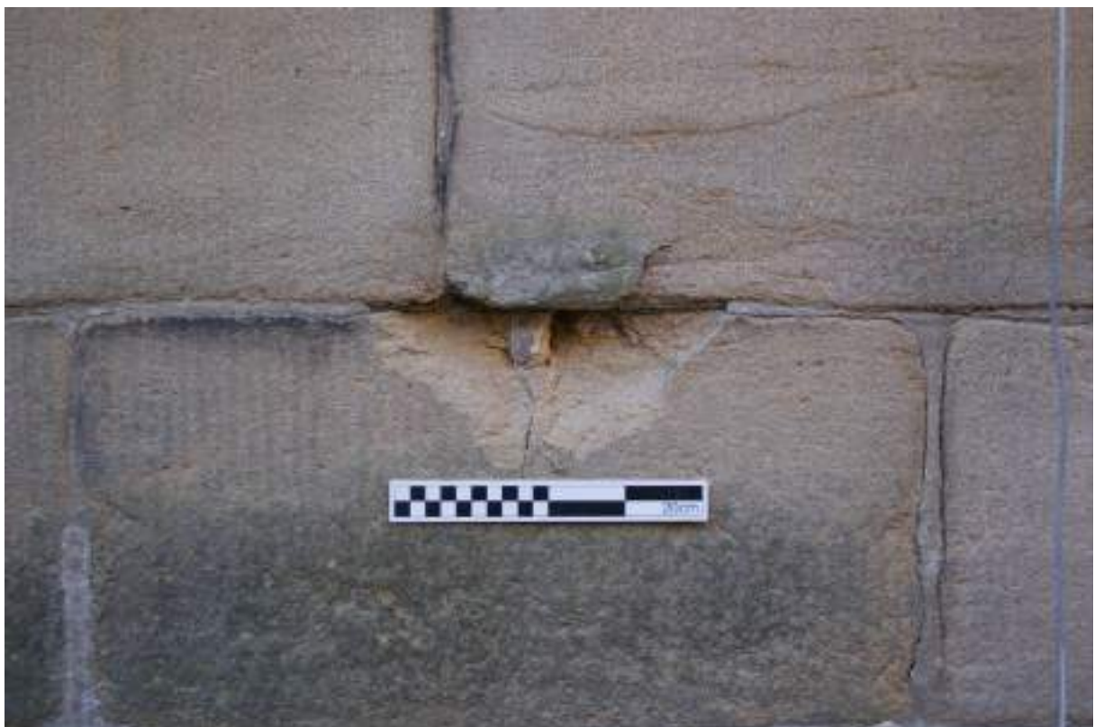
P23 (below). Detail of the ashlar facing to Narrowgate House at basement level, showing an example of the spalling around a leaded-in iron fixing. Scale 20cm.
