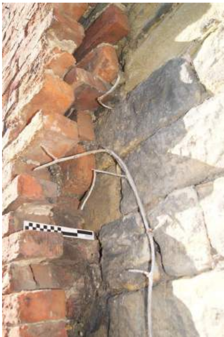
P3 (top). Detail of the 'hot wall' structure showing keying-in bricks, flues, and sooting on the earlier masonry boundary wall. Scale 20cm. NGA6/058
