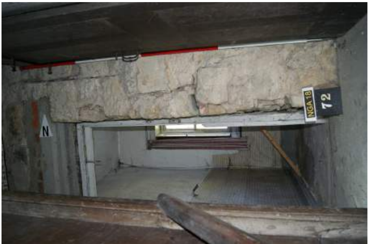
P72 (below). Room 15, looking west from the north stairs to the basement, showing vertical joint on masonry exposed by removal of wall-plaster. Door [72] to Room 15a is on the left, with inserted concrete lintels. Scale 2m
