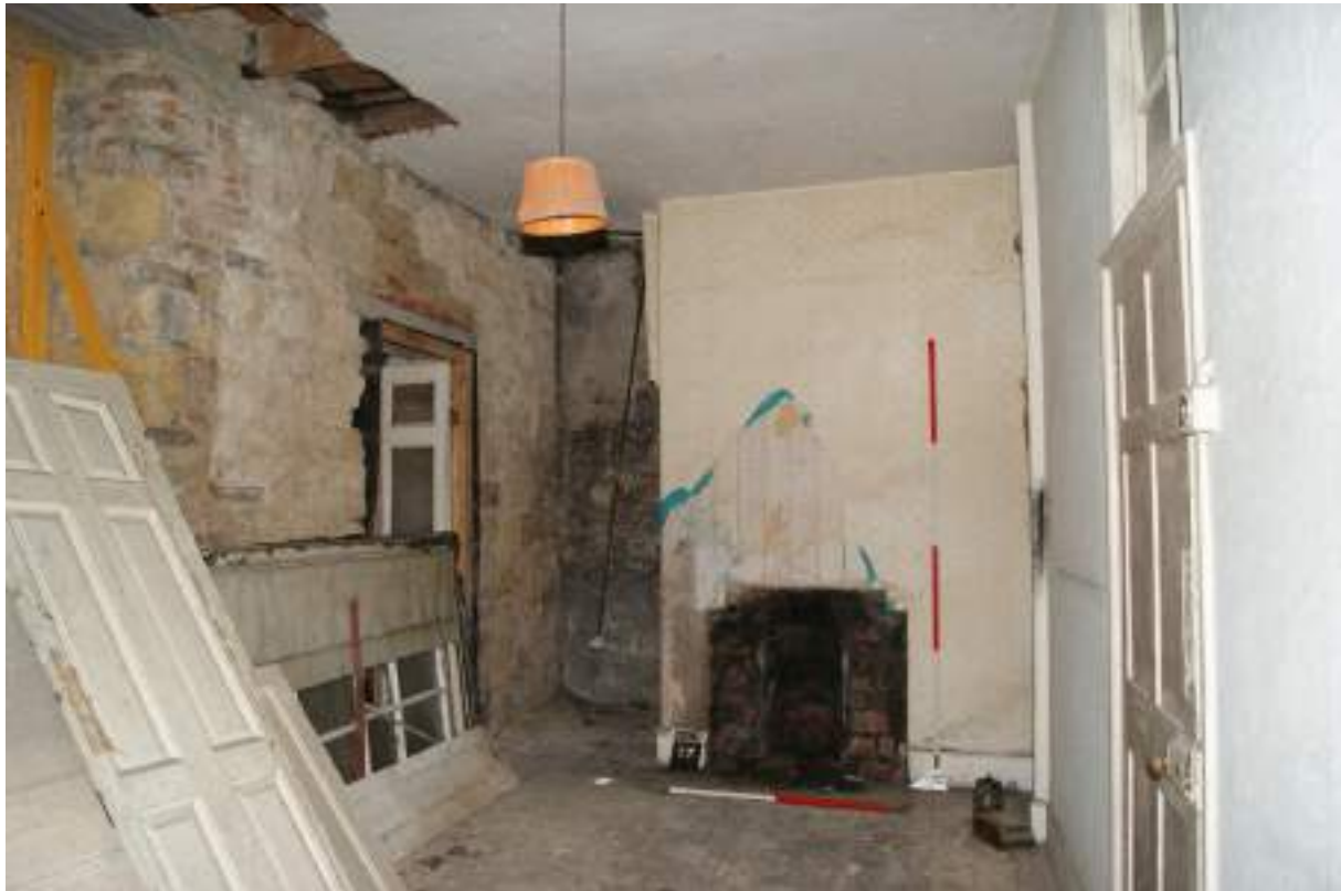
P73 (top). Room 15b looking north-west. Door [76] from passageway Room 6.1 on the right, fire [81] with former wall-cupboard [129] to left, and door [181] to Room 15c in the west wall, with inserted concrete lintel above, and detached fittings Scales 1m and 2m.
