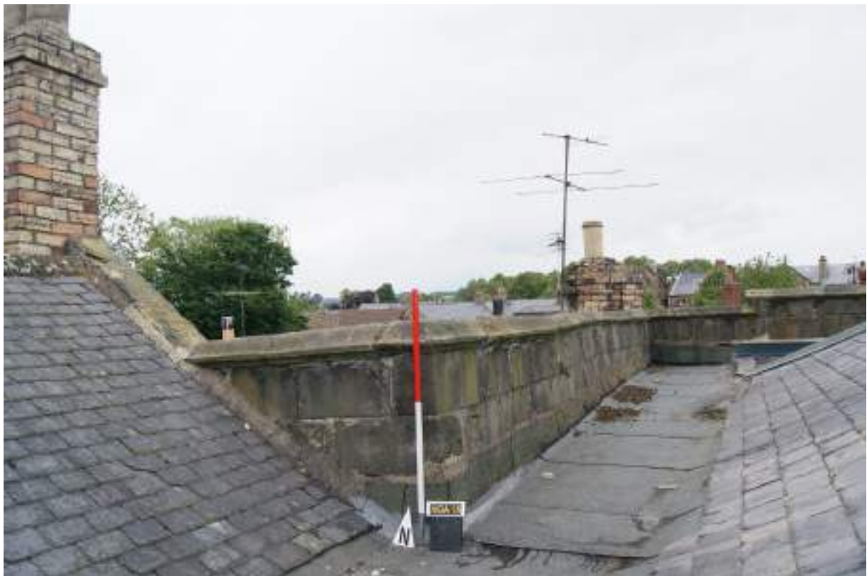
P131 (below). Detail, looking north, showing the return on the western parapet to join the north wall of the western extension, Chimney [191] and the 'step' on the northern parapet. Scale 1m.
