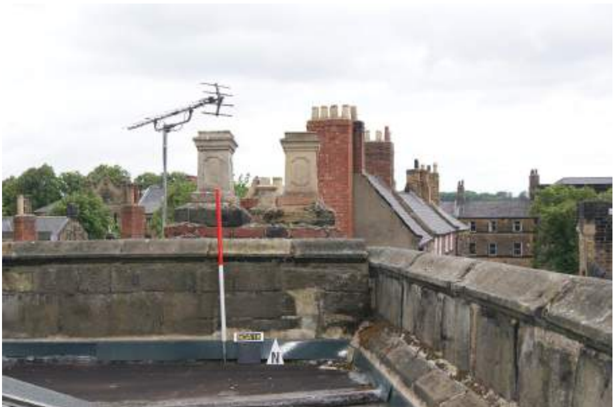
P133 (below). The north-eastern angle of the parapet looking north, showing base chamfer to the eastern parapet and evidence for remodelling shown in the 'step' on the coping. Scale 1m.
