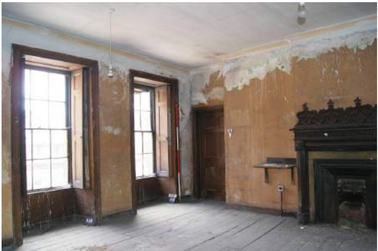
P98 (below). Room 16 looking south-east showing fire [112], door [110] to Room 17, windows [114] and [115], and modern ceiling soffit and replastering. Scale 2m.
