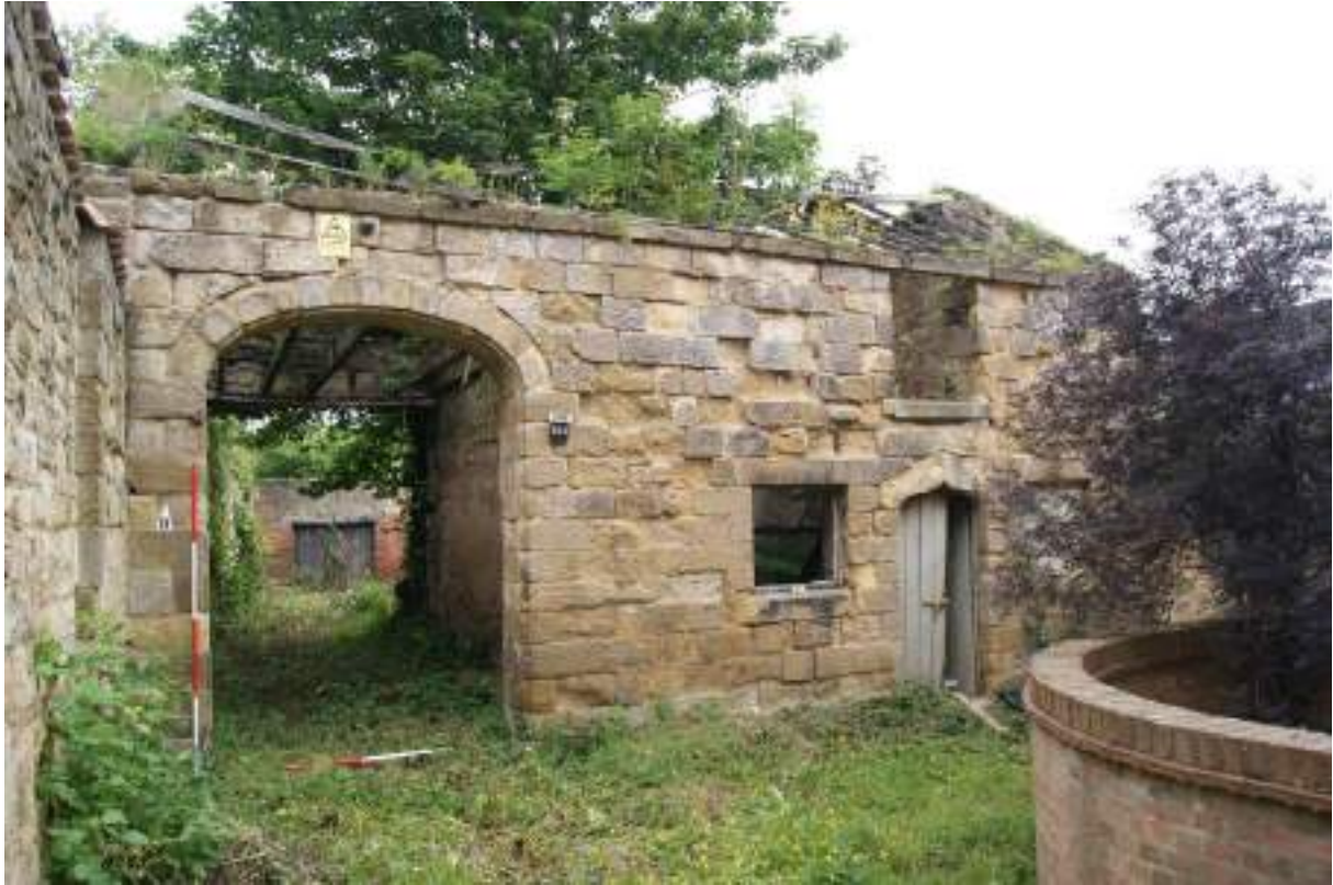
P4 (top). The coach-house and stables, south elevation, looking north-east. The carriage entrance [201] is on the left, window [202] and stable entrance [203] with pitching-eye [205] above is on the right. Scales 1m and 2m. NGA2/001
