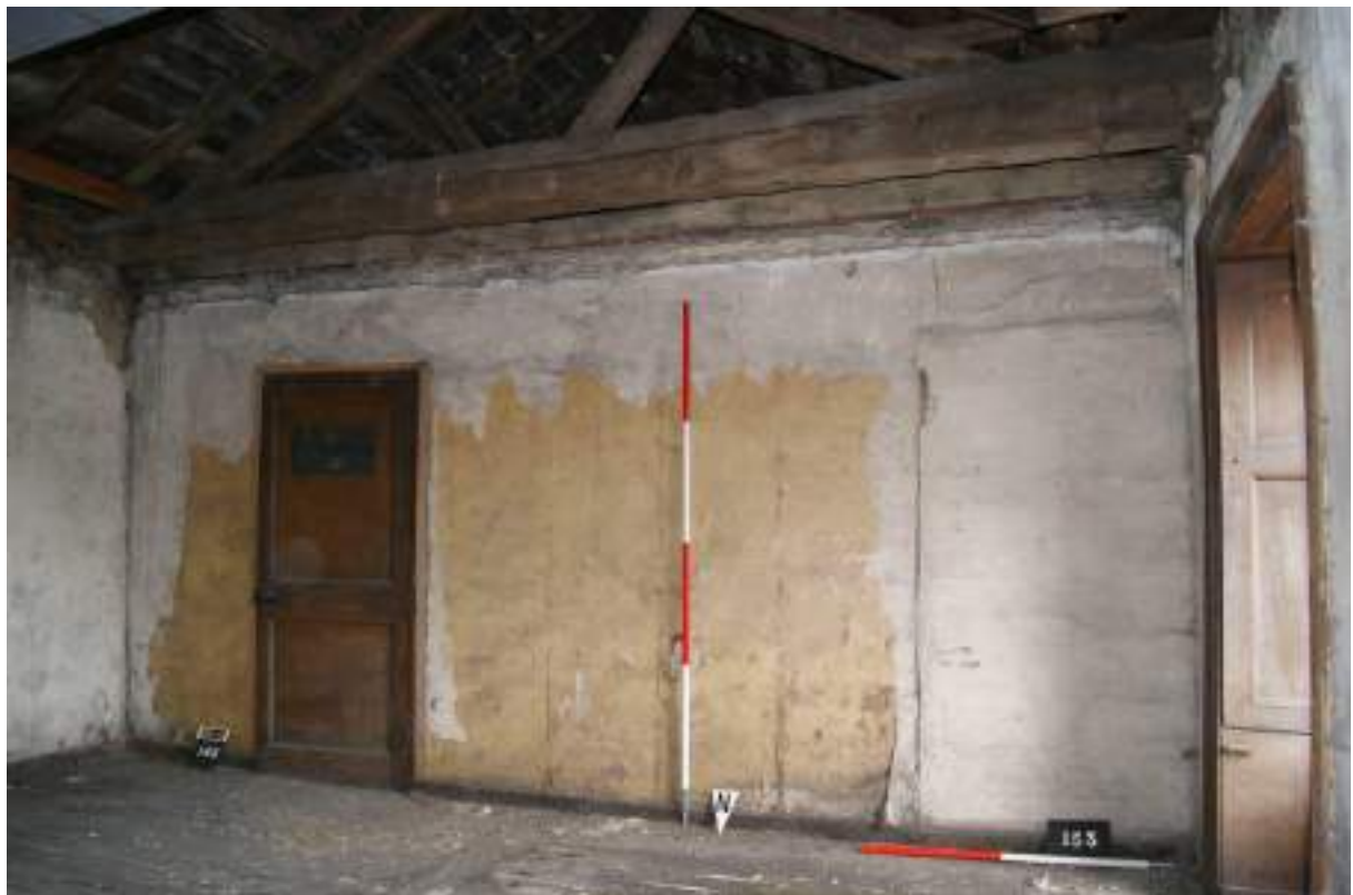
P112 (below). Room 36 looking north-west, showing door [143], blocked door [153] and roof-timbers. Horizontal and vertical lines of tacks for lining paper are visible in the plaster. Scales 1m and 2m.
