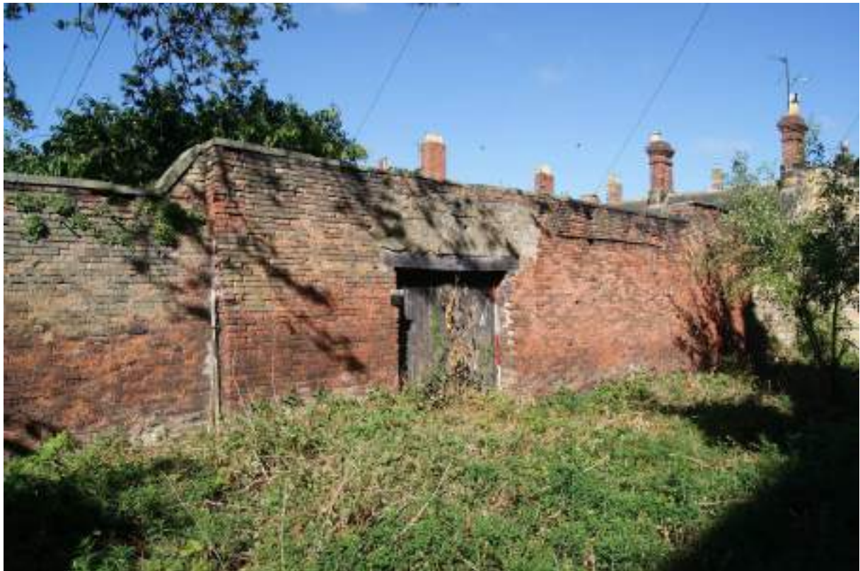
P1 (top). The north burgage boundary wall looking north-east showing the start of the 'hot wall', pierced by a later double-door vehicle access. Scale 2m. NGA5/060
