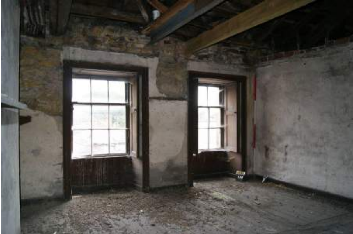
P119 (top). Room 34 looking east, showing windows [158] and [159], sandstone rubble masonry below lime-washed render, and roof timbers resting on scarcement on east wall. Thick deposits of pigeon droppings on floor. Scale 2m.
