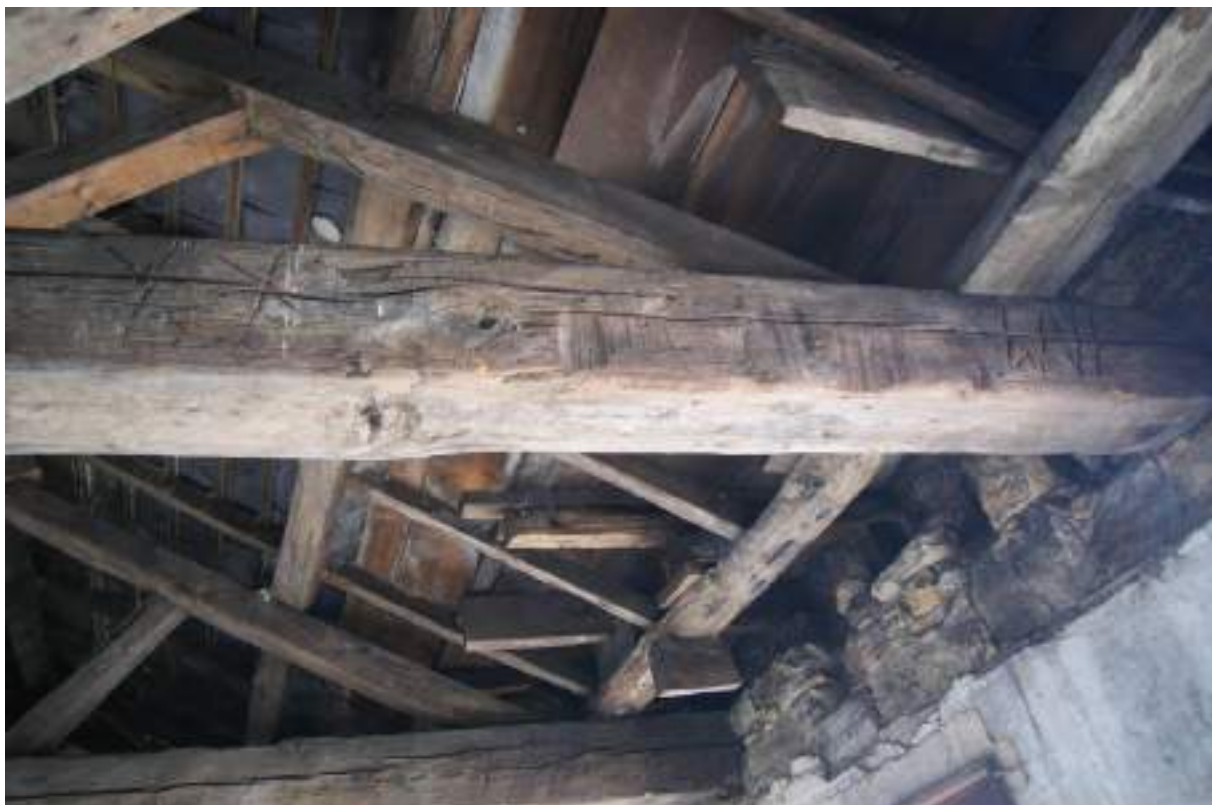
P114 (below). Room 36, detail of roof timbers resting on offset in east wall, with possible timber-merchant's and carpentry marks. No scale.
