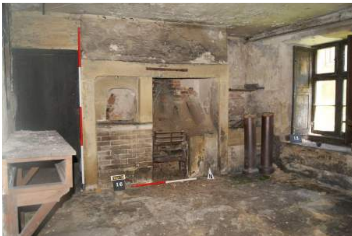
P34. Room 23. Looking north-east, showing range [16], alcove cupboard [17] (left), stone sink [15] (right, behind drainpipes) and window [13] (right). Scales 1m and 2m.
