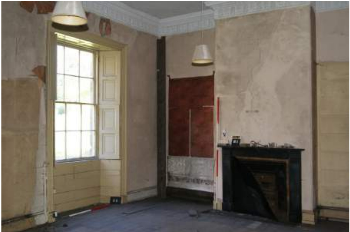
P69 (top). Room 7 looking north-west, showing fire [85], window [83] and decorative cornice. An area of wallpaper formerly concealed by shelving is visible in alcove [87] to the left of fire. Scales 1m and 2m.
