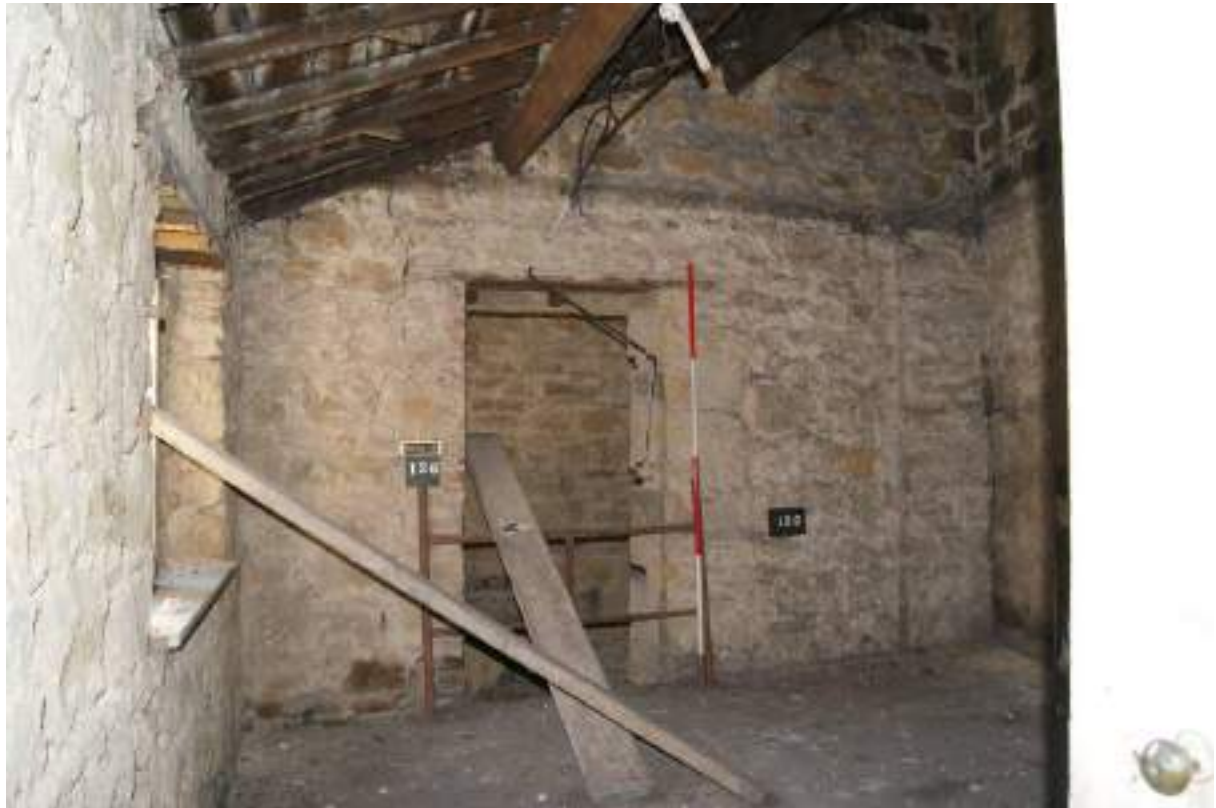
P105 (top). Room 20 looking west to opening [126] leading to Room 21, reveal of blocked opening [125] to the right, and butt-joint between the west and north walls. The scars of the lath and plaster ceiling soffit and a shelved wall cupboard are visible. Scale 2m.
