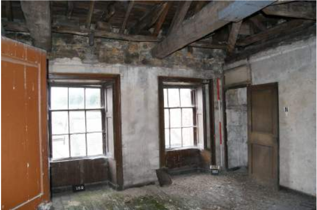
P111 (top). Room 36 looking south-east, showing cupboard [150], windows [151] and [152], and beams resting on offset on east wall. Scale 2m.
