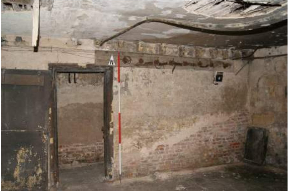
P31. Room 22 looking north-east showing door [7], servant's bells [6], and truncated north-south joists to 1 st floor. A detached stone sink leans against the east wall. Scale 2m.
