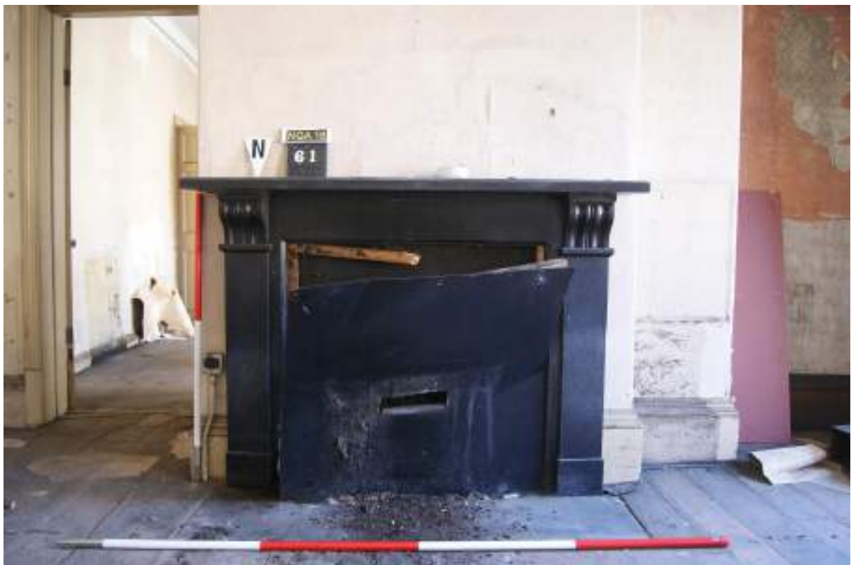
P62 (below). Room 3. Detail of fire [61] showing sheet iron blanking-plate associated with a late 20 th century gas fire (removed). Scales 1m and 2m.
