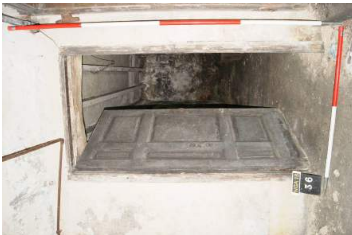
P42. Room 30 looking west into doorway [36], showing assymetric panel leaf. An H-hinge on frame to door [33] (Room 29) is just visible on right. Scales 1m and 2m.
