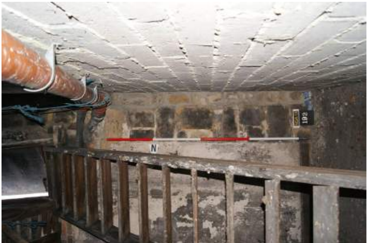
P108 (below). Room 40 looking east showing quoins of single pile house, ladder to rooftop, and 2003 breezeblock rebuilt south gable to the right. Scale 2m.
