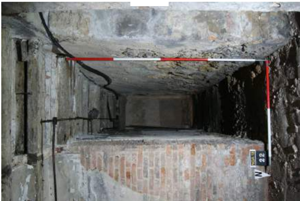
P37. Doorway [22] into R24 looking south along corridor R21, showing finished return to brick partition wall and east-west joists to first floor. Scales 1m and 2m.
