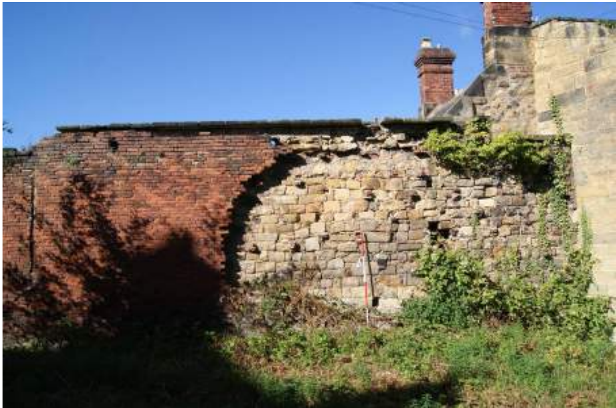
P2 (below). Collapsed section of the 'hot wall' showing keying-in bricks and the exposed stone wall behind, with coping slabs and vents. Scale 2m. NGA6/059
