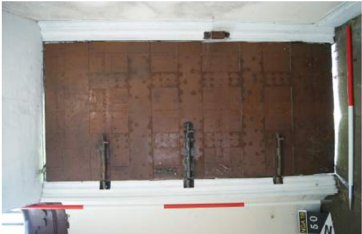
P51 (top). Room 8, looking west to the inner face of door [50] showing iron sheeting. Scales 1m and 2m.
