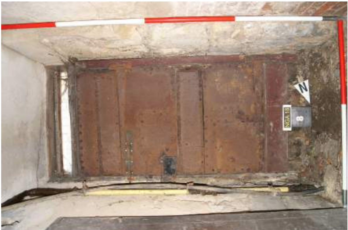
P32. Room 25 looking east to door [8] showing sheet-iron backing. Door [9] to wall-cupboard is visible on the left. Scales 1m and 2m.
