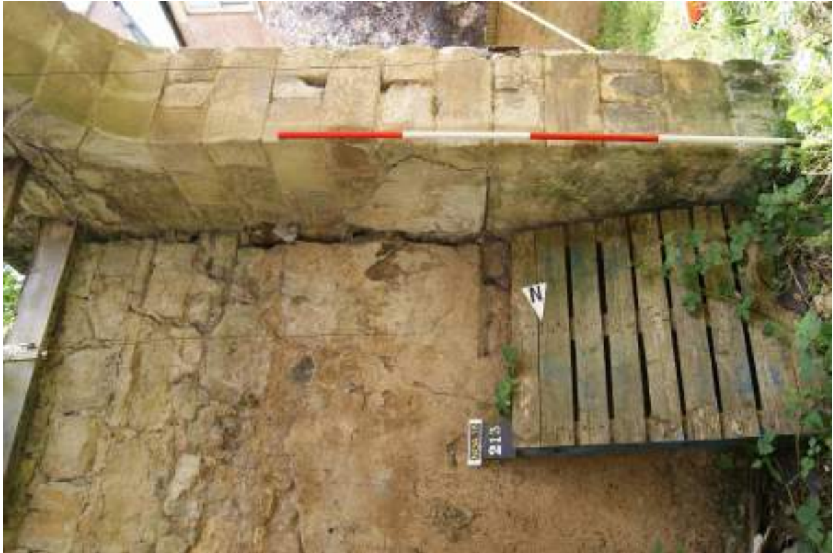
P16 (top). Interior of the coach-house, looking south-east, showing the east jamb of the entrance [201], the butt-joint between the internal and external walls, and the scar of missing shelf [213]. Scale 2m. NGA2/022
