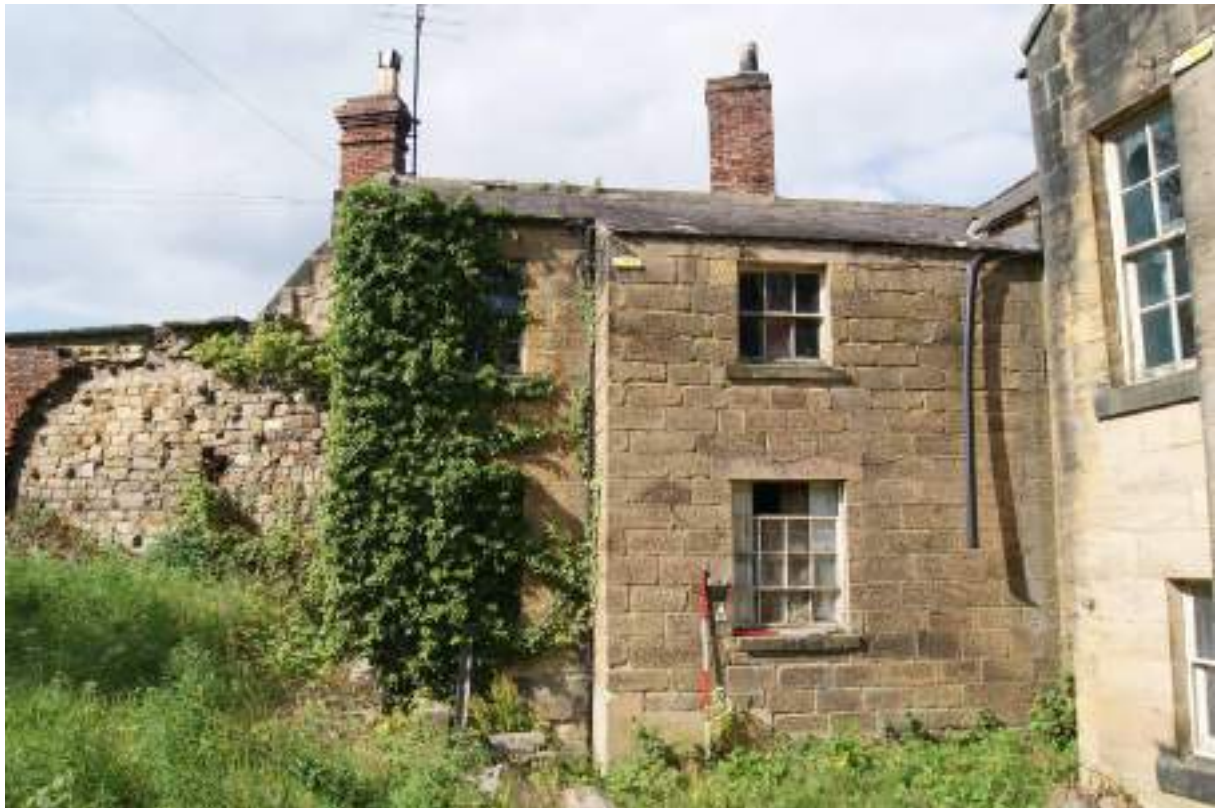
P28 (top). South facing facades of the western out-shots to No.33 showing chimney [195], windows [80], [82] (concealed by creeper), [123] and [127] (concealed by creeper). The brick "hot wall" is to the left. Scales 1m and 2m.
