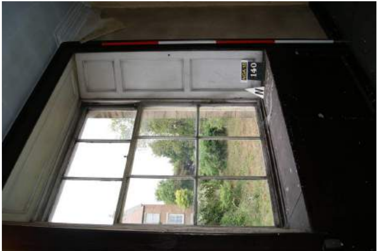
P87 (top). Room 12, detail of window [140] showing 6/3 sash, shutters, and window seat with hinged lid for storage. Scale 2m.
