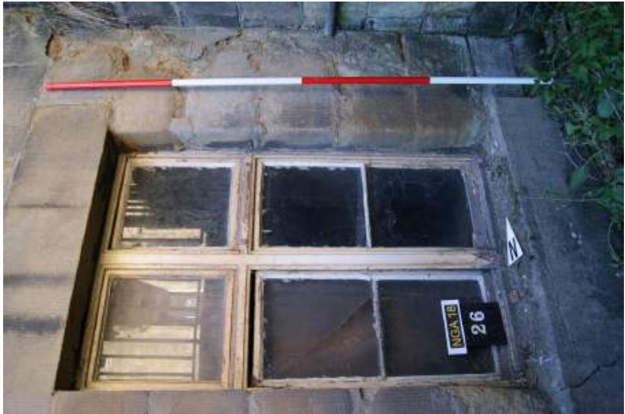
P22 (top). Basement window[26] showing casements, and the butt joint between the ashlar facing of Narrowgate House and the earlier masonry carrying the steps up to the door of No.33. Scale 2m.
