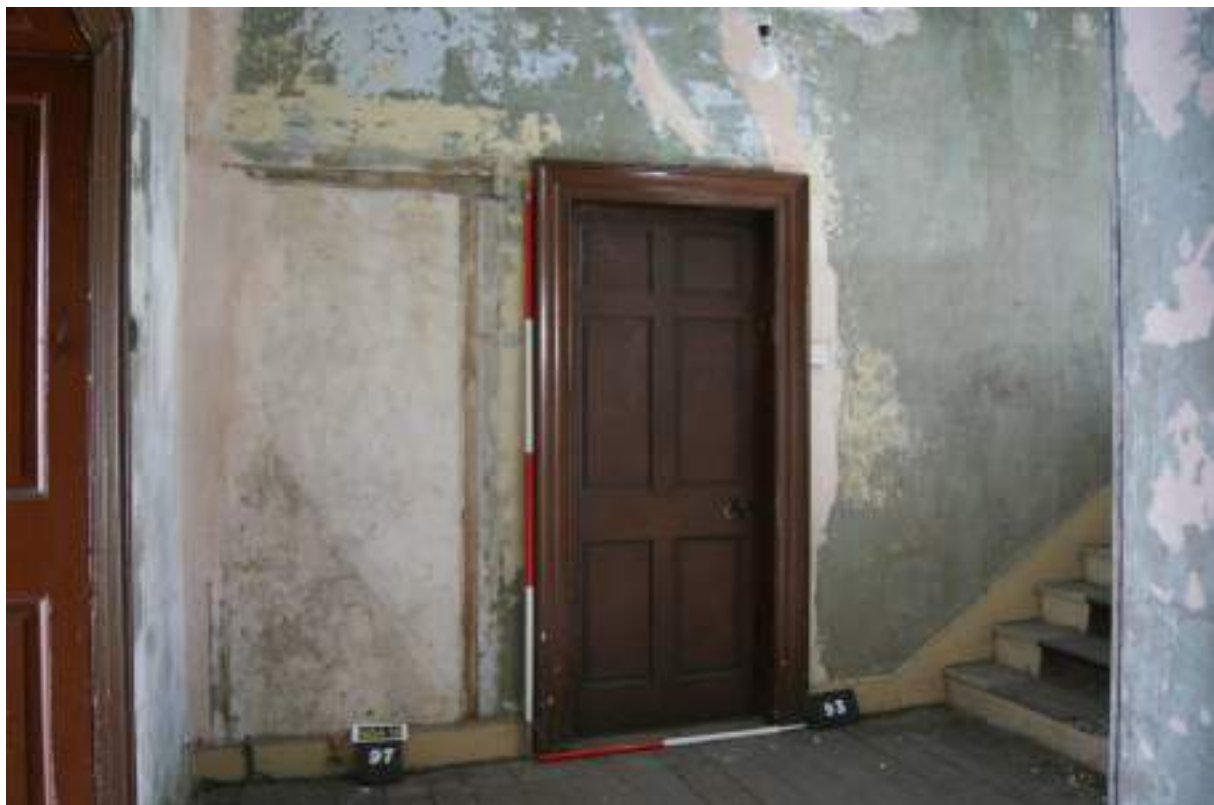
P82 (below). Room 8, looking south to doorway [93] into Room 10, also showing outline of blocked door [97]. Scales 1m and 2m.
