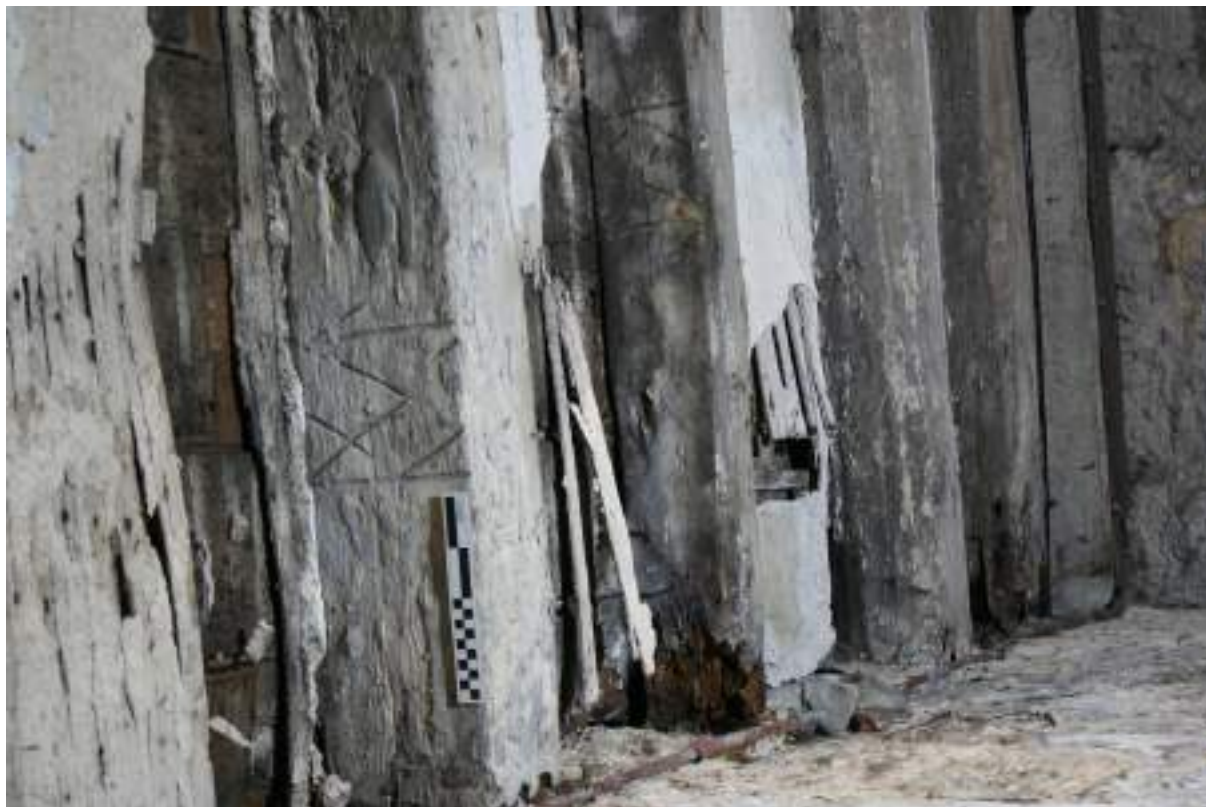
P41. Room 24, detail of joists to 1 st floor looking north, showing timber-merchant's mark. Scale 20cm.
