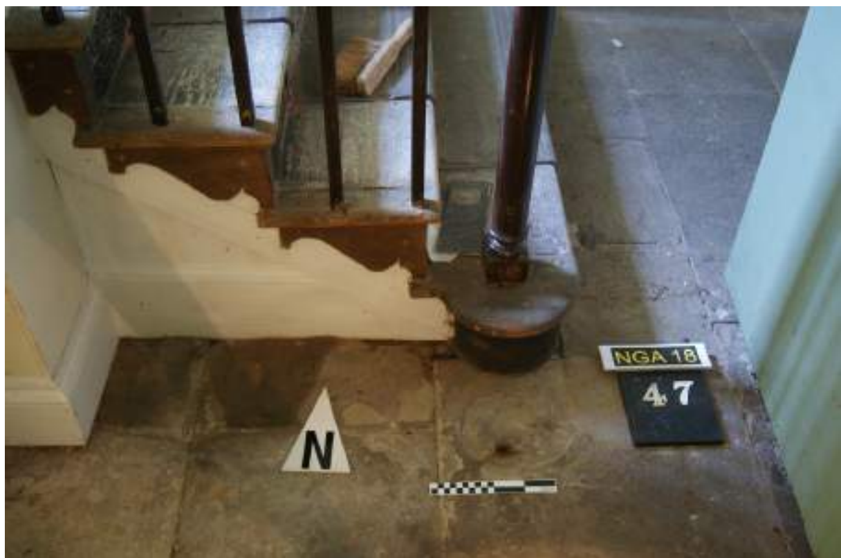
P50 (below). Room 8/9 showing scar of former curtail step on the south side of stair [47] with iron fixing in the flagged floor. Scale 20cm.
