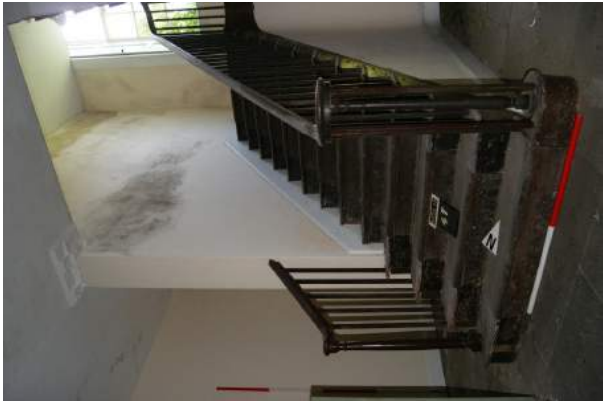
P49 (top.) Room 8/9 looking south-west, showing first flight of main stair [47] and altered southern handrail. Scale 1m.
