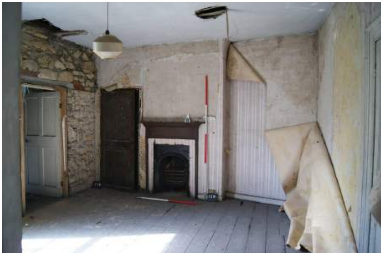
P102 (below). Room 19 looking north-west, showing fire [119] with wall-cupboard [120] to the left, and the west wall stripped of render with modern concrete lintel and repairs above door [122] leading to Room 20. Scales 1m and 2m.
