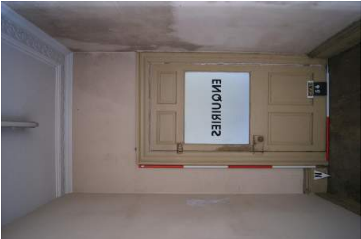
P58 (below. Room 3, looking south to door [54] showing the decorative cornice cut by the west partition wall of Room 3.1. Scales 1m and 2m.
