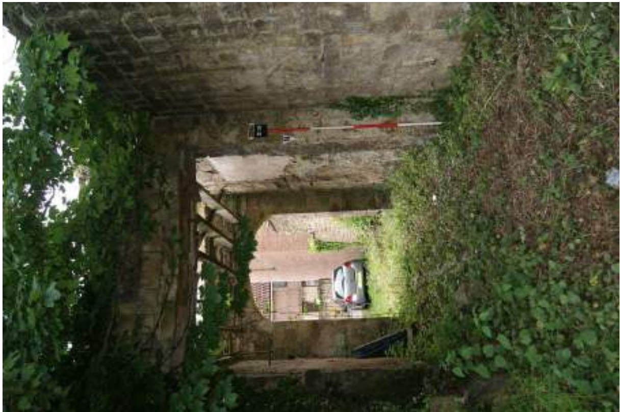
P14 (top). Looking south into the coach-house through the inserted double-doorway [209], showing timber lintel and joists to first floor. Scale 2m. NGA2/019
