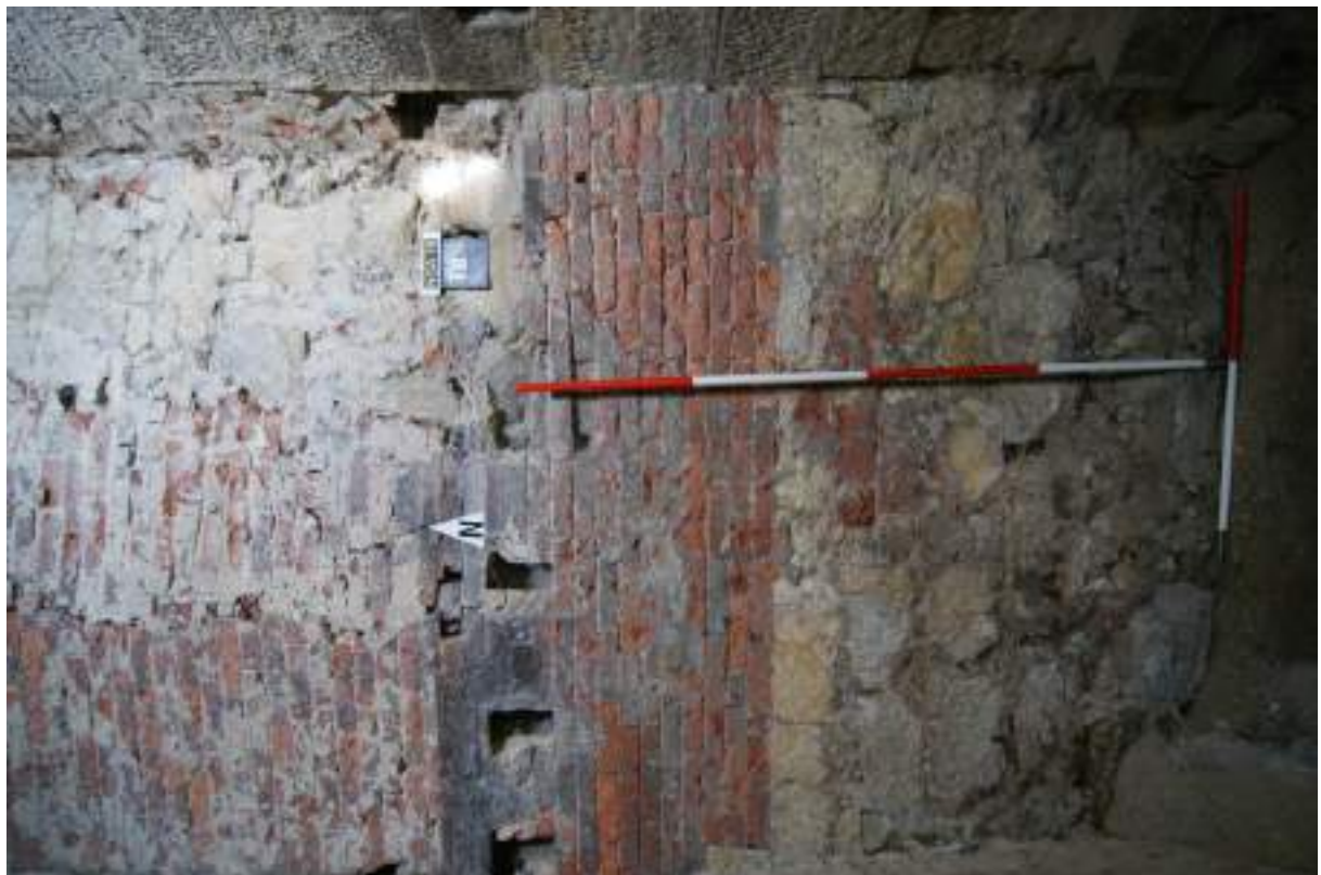
P78 (below). Room 15d. North wall, showing sandstone base with brickwork above containing sockets for former floor joists, and patched brickwork forming part of the external 'hot wall', cut back' to accommodate (missing) timber stairs. Scale 1m and 2m.
