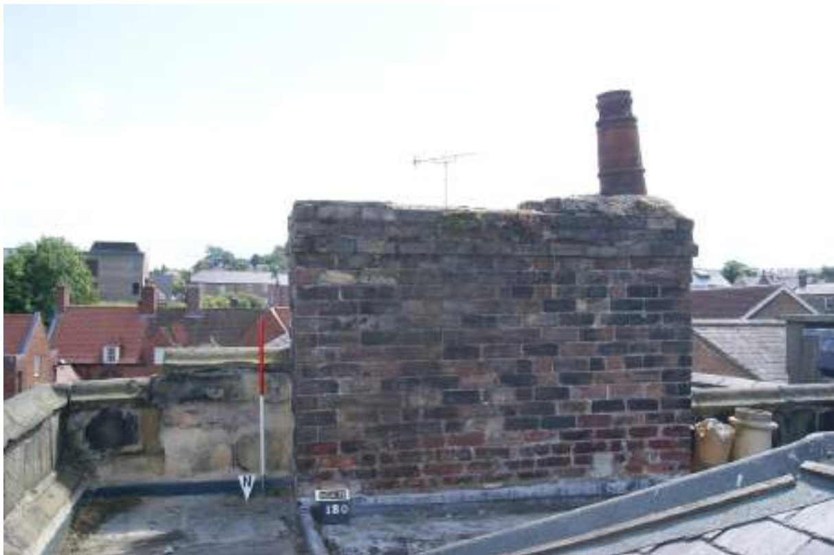
P135 (below). Detail of the south-eastern angle of the parapet showing evidence for remodelling, and chimney [180]. Scale 1m.
