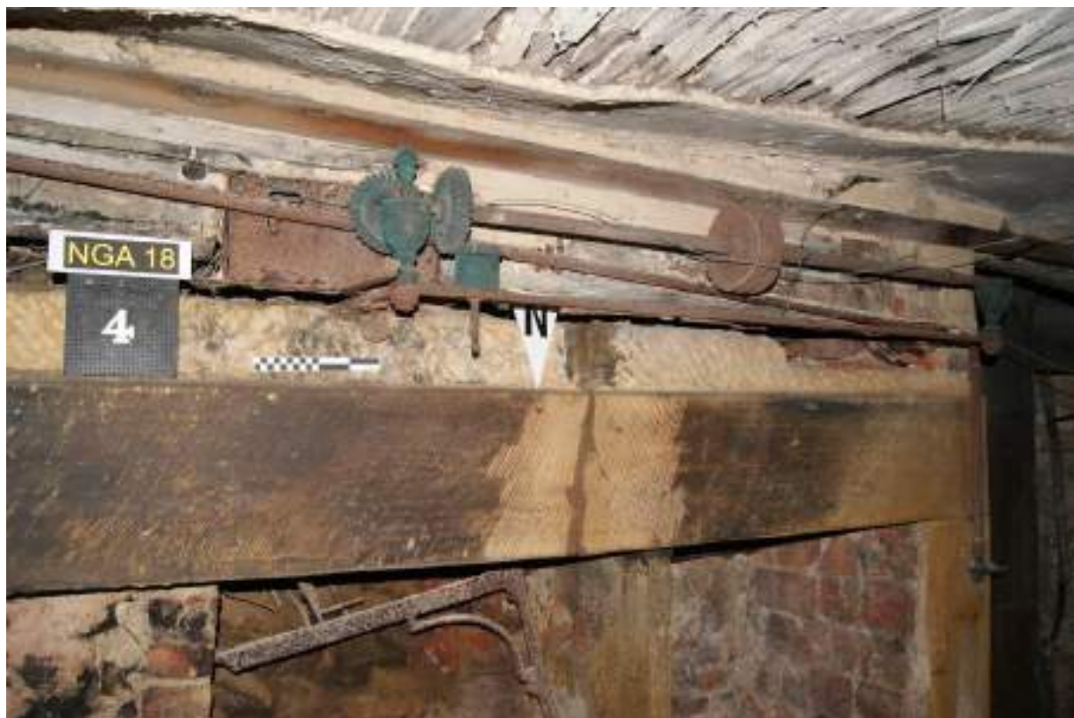
P30. Room 22. Detail of range [4] showing opposed gearing for a roasting spit driven by a fan in the flue, and the pot-crane. Scale 20cm.
