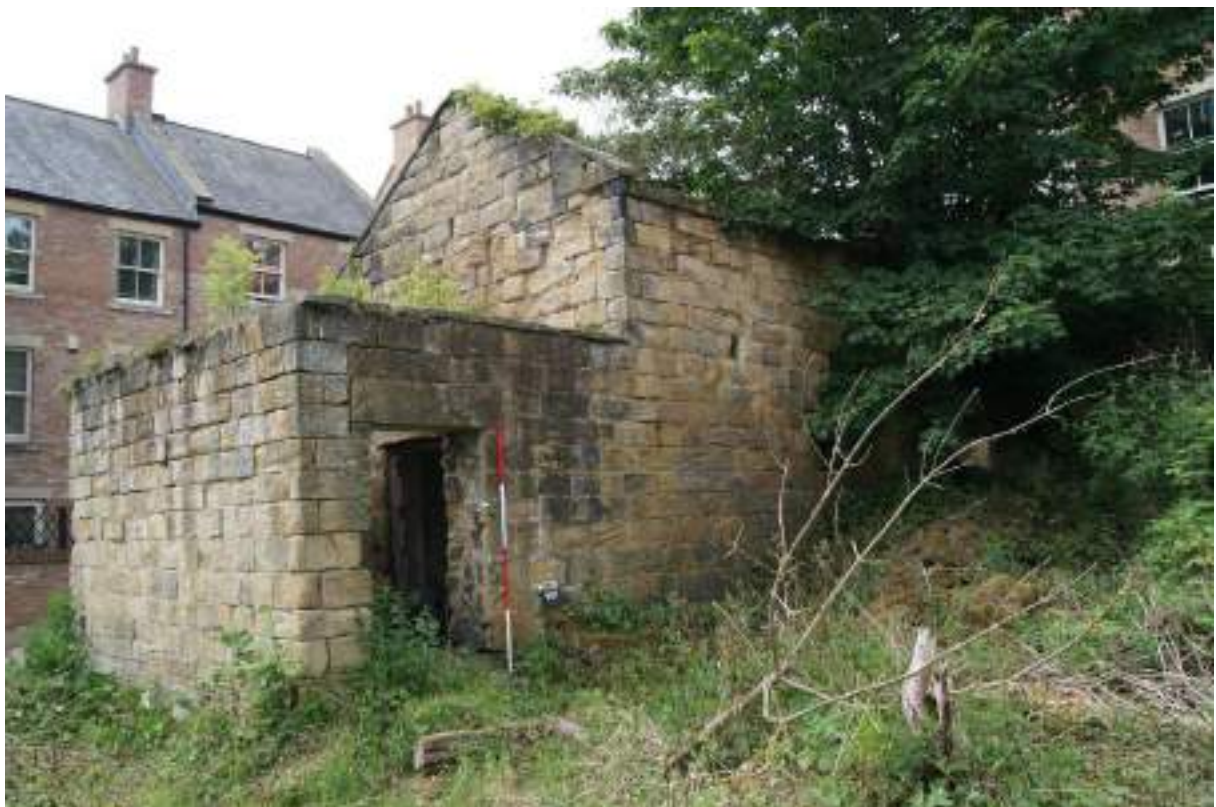
P13 (below). The stables and yard looking south-west, showing the north doorway [207] to the yard and one of the beam-slots [208] in the north wall of the stables. Scale 2m. NGA2/016
