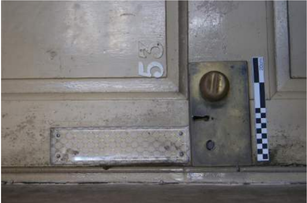
P65 (top). Room 3, detail of door [53] showing 19 th century brass-cased lock (inverted) with ball handle and late 20 th century perspex finger plate. Scale 20cm.
