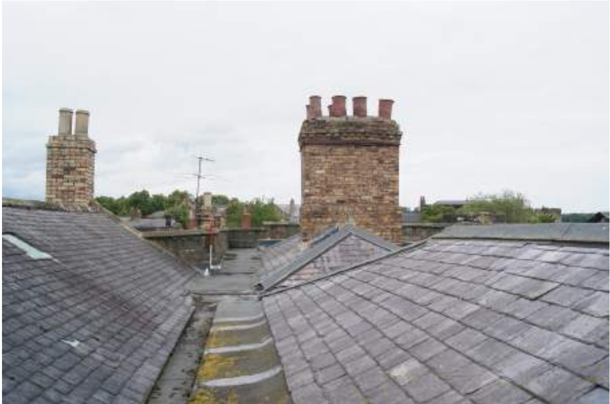
P130 (top). Looking north along the valley gutter from roof access door [194], showing (left) c himney [191] serving Rooms 39,13 and 7 of the western extension, and (right) chimney [193] serving Rooms 34/38,16/173/4 and 23/24, and the hipped roofs of the single-pile house. Scale 1m.
