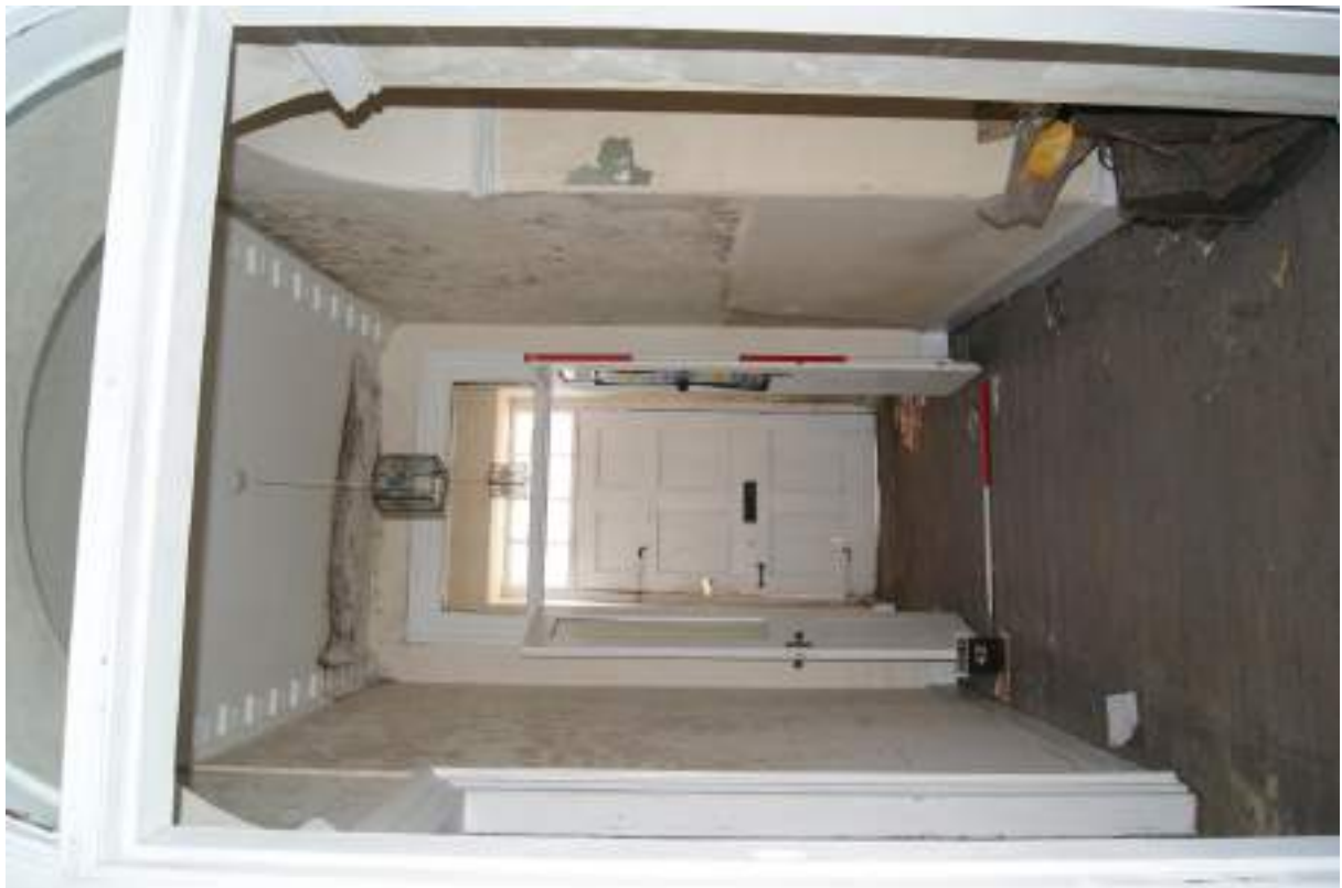
P46 (below). Room 2 looking east from doorway [45], showing lobby partition [42] cutting frieze. Scales 1m and 2m.
