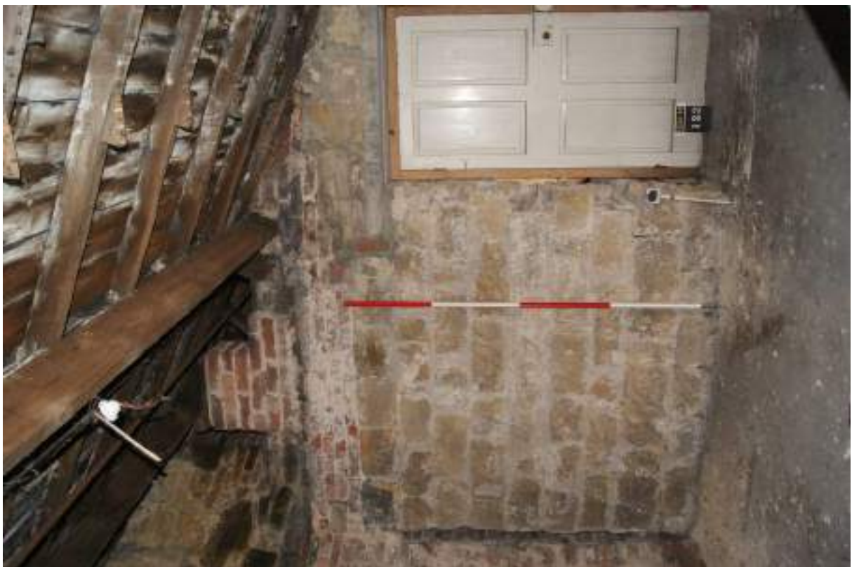
P104 (below). Room 20, looking east to door [122] in modern frame, butt-joint between east and north walls on the left, and brickwork raising the roof level above. Scale 2m.
