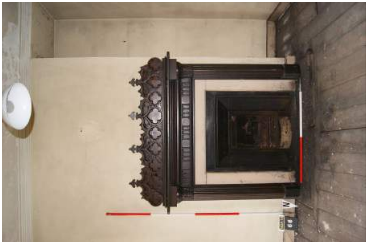
P84 (below). Room 18, fire [99] (photoboard inverted) with Gothic moulded timber surround. Scales 1m and 2m.
