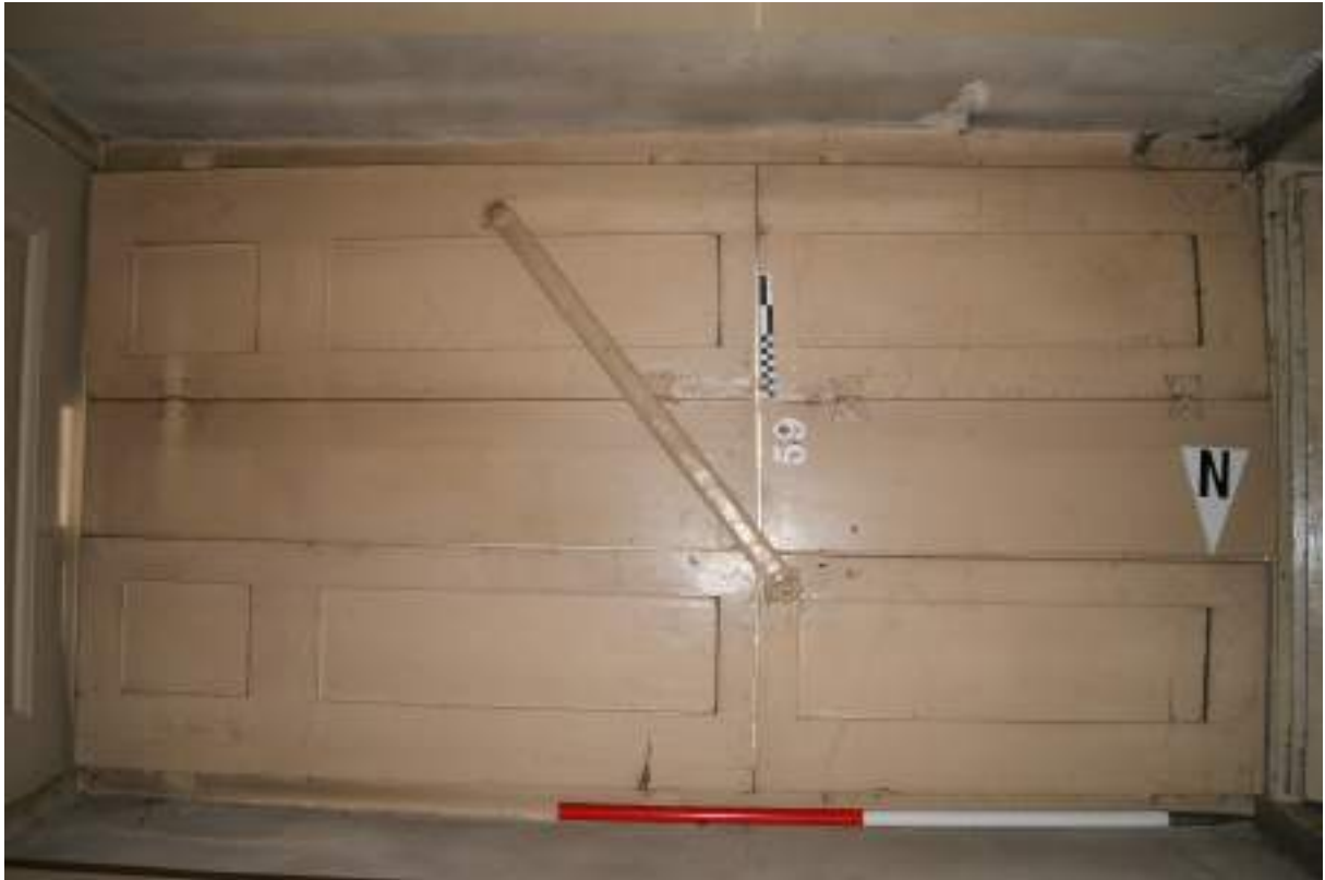
P63 (top). Room 3, window [59] showing internal view of shutters with plain central leaf and locking bar. Scale 1m.
