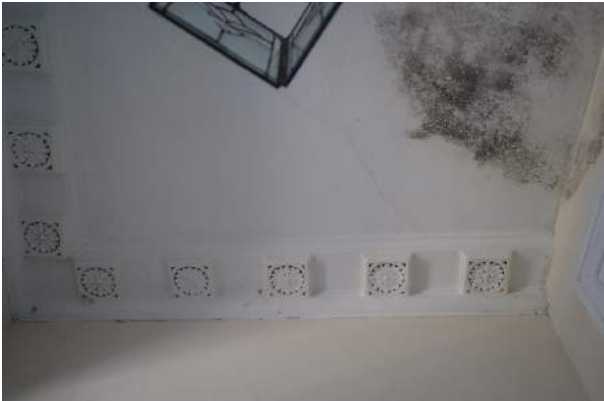
P47 (top). Room 2, ceiling showing a detail of the frieze cut by lobby partition [42] (on the right). Also showing damp staining from Room 18 above. No scale.
