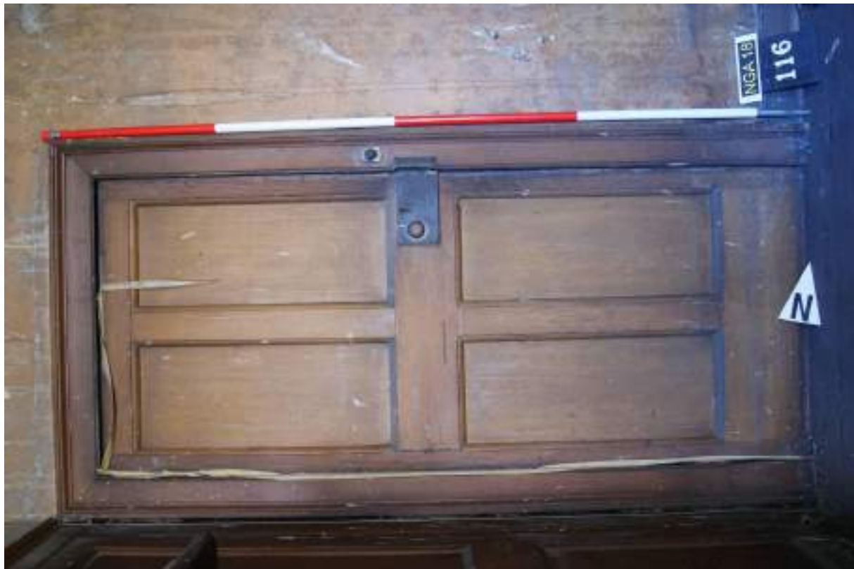
P101 (top). Room 16, detail of door [116] showing inverted brass-cased lock and ball handle with bell-knob in the architrave. Scale 2m.
