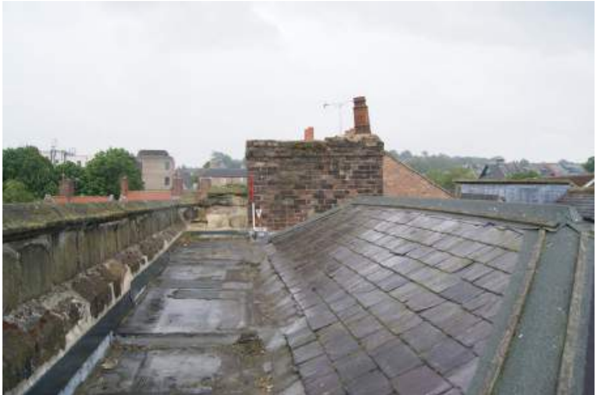
P134 (top). Looking south along the eastern parapet showing base chamfer, chimney [180] serving fires in Rooms 36,18 and 22, and the slated hipped roof over 31 Narrowgate. Scale 1m.
