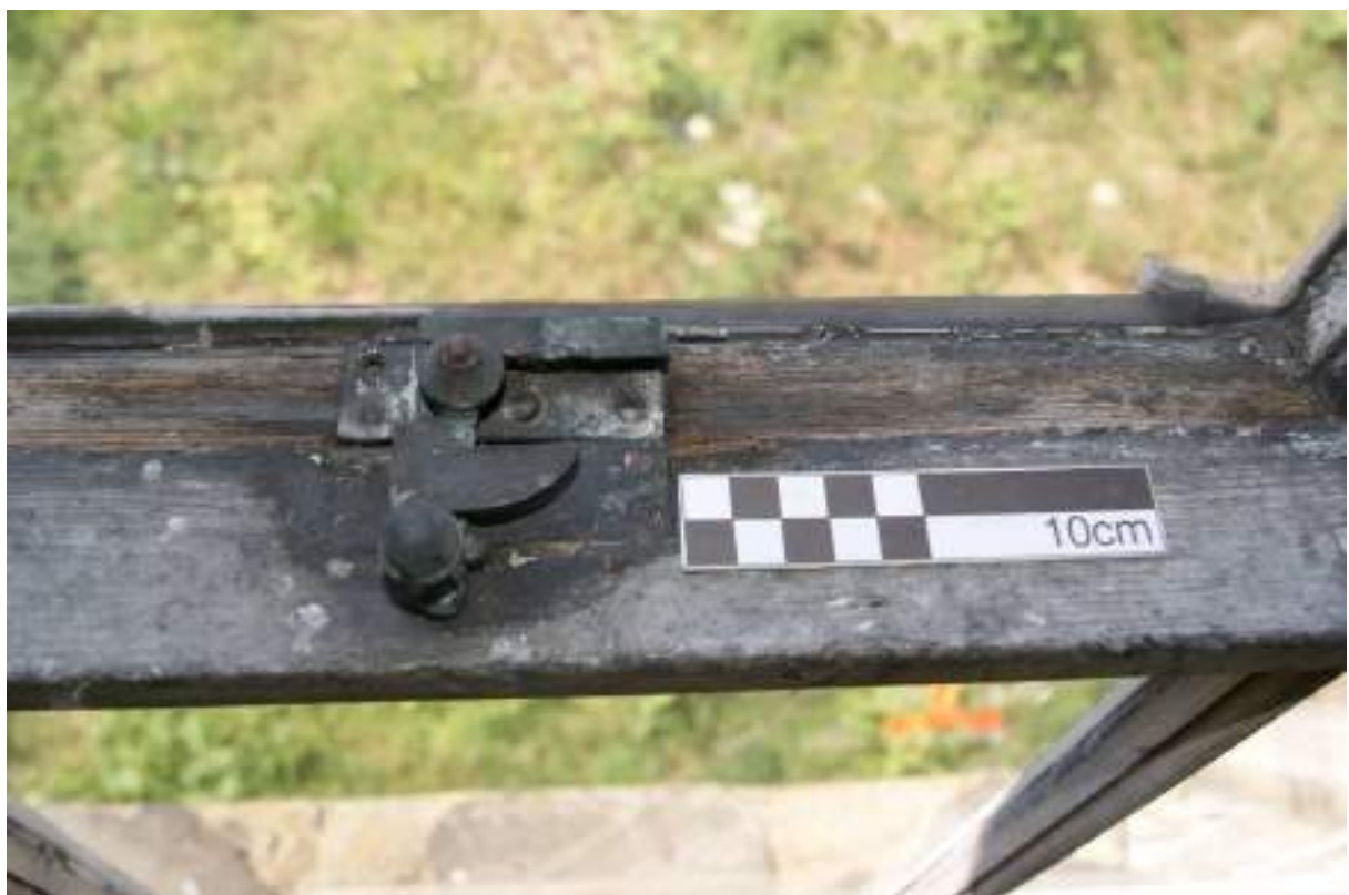
P88 (below). Room 12, detail of original cast brass catch on sash frames. Scale 10cm.
