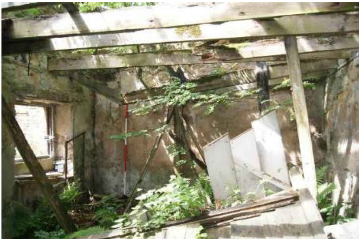
P7 (below). Stables: interior looking west, showing window [202], butt-joint between the west partition wall and the external south wall, and fallen/collapsing timberwork. Scale 2m. NGA2/008
