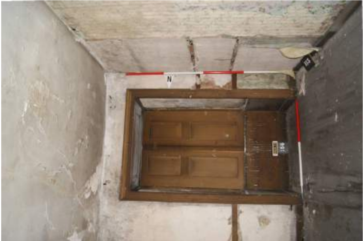
P115 (top). Room 35, looking east to window 156] with shutters closed. Scars of shelving visible on the adjoining walls. Scales 1m and 2m.
