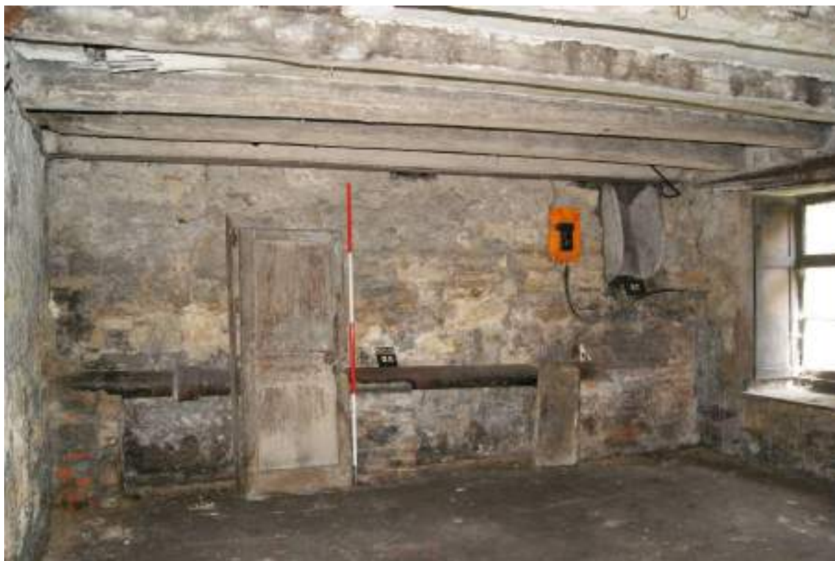
P39. Room 24 looking north-east, showing masonry wall, sewer pipe [28], chute [27] near window [26], and detached door leaf with H-hinges. Scale 2m.
