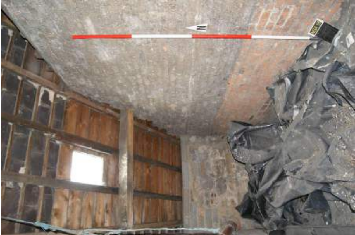
P109 (top). Room 40 looking north-west showing brick partition forming the south side of the stairwell and discolouration probably indicating the site of the bath of the 19 th century building. Scale 2m.
