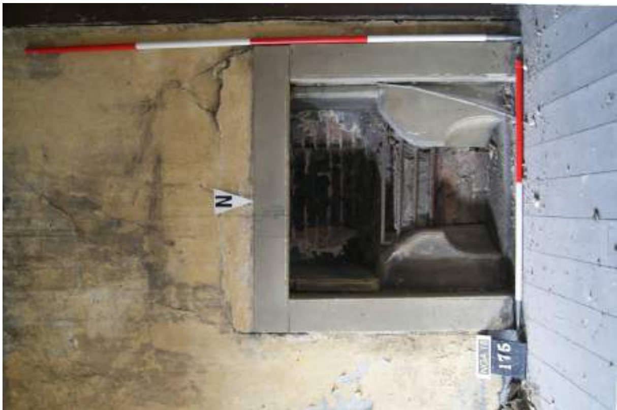
P126 (below). Room 38. Detail of fire [175] showing sandstone sides perhaps imitating a Bath grate Scales 1m and 2m.
