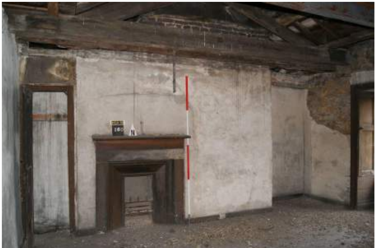
P120 (below). Room 34 looking north-east, showing fire [160] with brick breast rising above the lime-washed render, and wall-cupboard [161] on the left. Window [159] just visible on the right. Pigeon dung and carcasses on the floor. Scale 2m.
