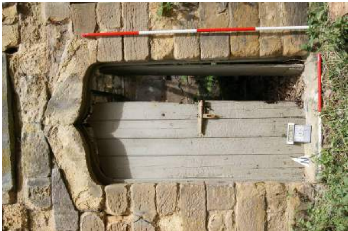
P5 (below) Stable entrance [203], showing ogee arch and two-section door leaf (left) with single leaf open. Scales 1m and 2m. NGA2/013
