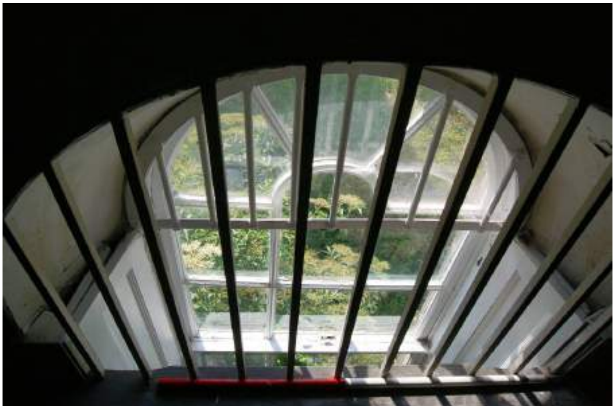
P80 (below). Window [92] transected by the half-landing of the lower flights of the principal stairs [47], showing iron grille and robust glazing bars. Scale 1m.
