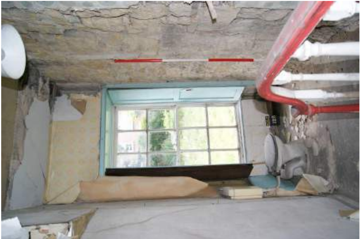
P91 (top). Rooms 11a and 11b, looking west from [130] to window [128] showing scars of former partition, and cut through the west wall of the first western extension to No.33 (right). Scale 2m.
