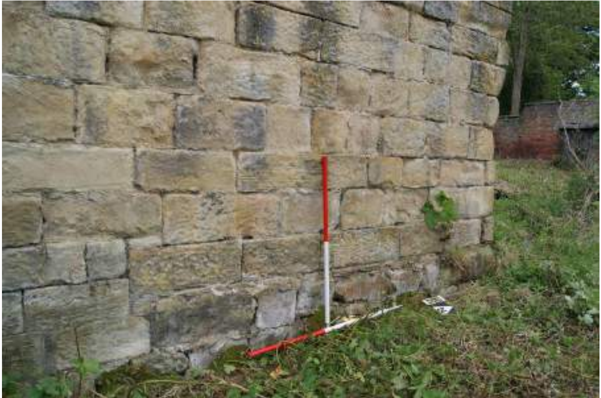
P12 (top). Detail of the east wall of the yard, showing construction joint and differences in the the build to the south and north. Scales 1m and 2m. NGA2/026
